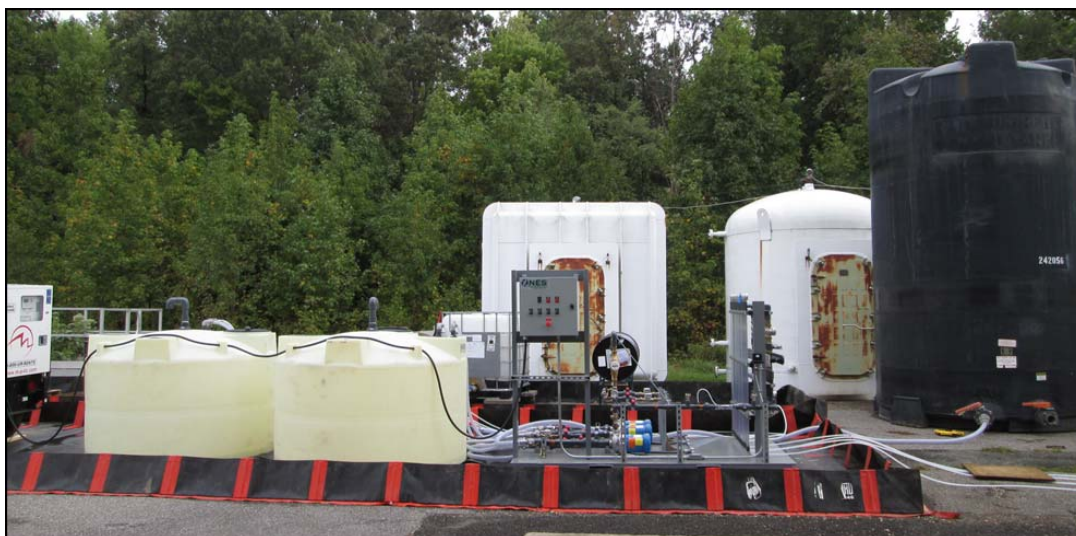
Figure 6.3: Injection Skid Assembly with all Components
