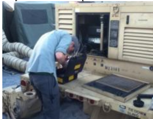
Figure 14: REACHE ADVON team installs automated sensors
