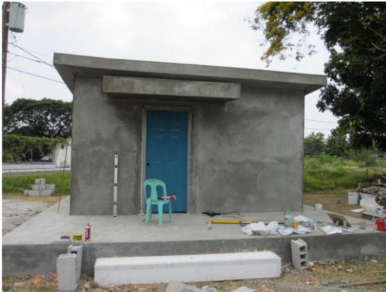
Figure 15: SABS 200 Sqft building construction at Camp Aginaldo
