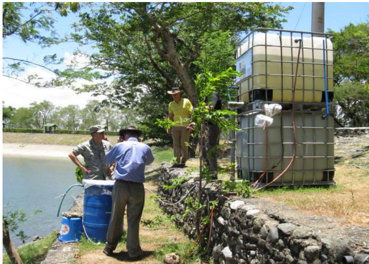
Figure 11: UH Slow Sand Filter deployed at Magsaysay
