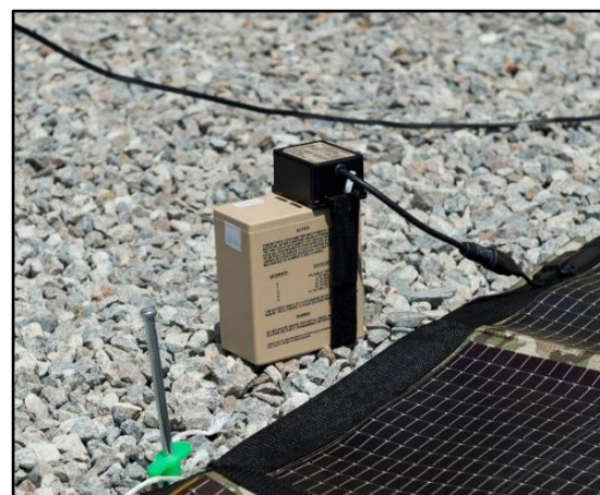
Figure 99: Battery Charged by Panel
