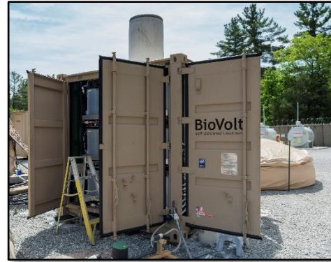
Figure 31: Wastewater Storage Tank (background-right)
