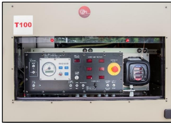
Figure 107: 100-Amp Shark Meter in T100
