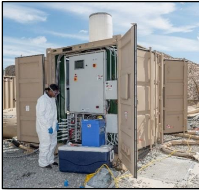
Figure 30: WWT-D2 Housed in a TRICON
