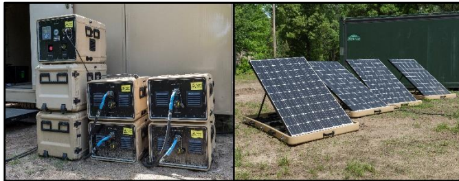
Figure 7: Microgrid and Photovoltaic Panels Array
