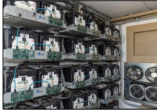
Figure 43: Inverter/Battery System
