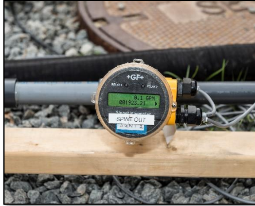
Figure 106: Water Flow Meter
