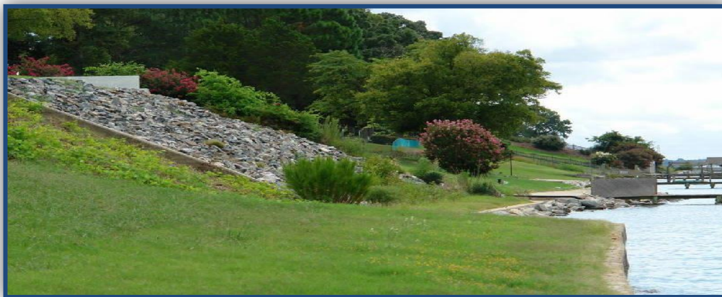
Figure 71. (a) Example of bulkheads along creek draining into Lafayette River, Norfolk. Tide was unusually high and yards were only about 0.3 m above the water surface. (b) Revetment installed by property developer along north shore of James River at Wareham's Pond Road, near Williamsburg, VA. (c) Professionally-installed bluff armoring, north shore of James River near Newport News. Photographs 24-25 August 2010.
