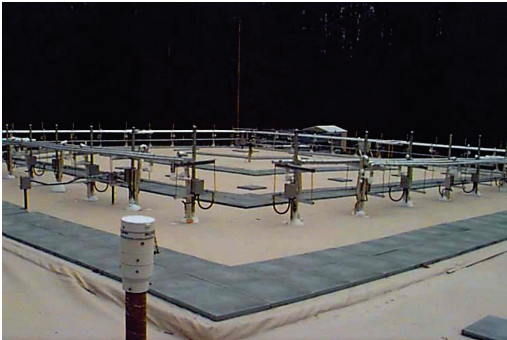
Figure 5. Thermosyphon system for hazardous waste containment at Oak Ridge National Laboratory, Tennessee.
