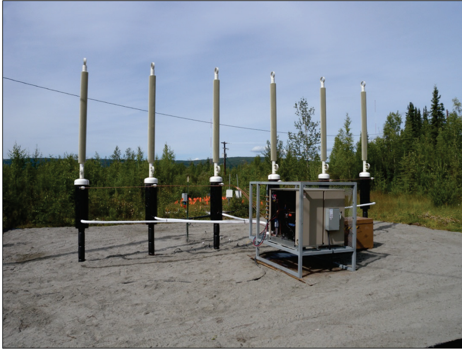
Figure 14. Complete installation of the hybrid thermosyphons and refrigeration unit.
