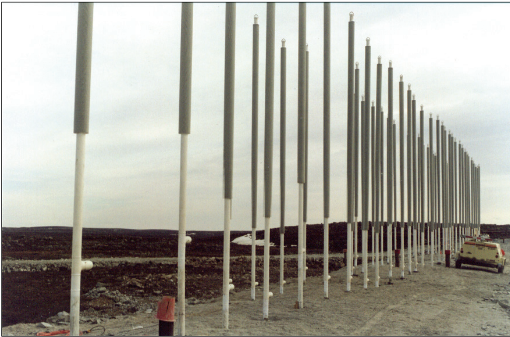
Figure 6. Thermoprobes at the Long Lake Outlet Dam, Ekati Diamond Mine, Northwest Territory, Canada.
