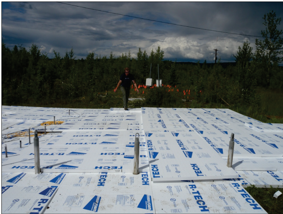
Figure 13. Insulation installation.
