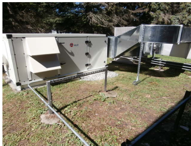
Figure 10. The Installed LDDX-WF Prototype
