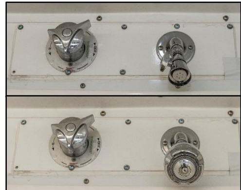
Figure C-41. Baseline showerheads (top) and low-flow showerheads (bottom)
