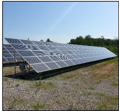
Figure C-69. Solar panels arranged into solar array
