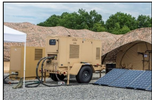
Figure C-21. Generator, MSDU, and Solar Array (left to right)
