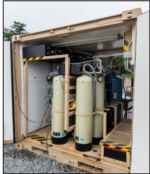
Figure C-78. UF GWRS – Interior View
