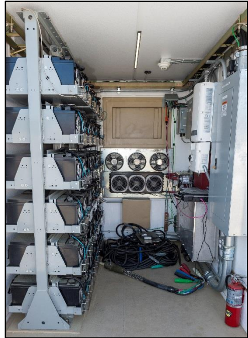
Figure C-28. Energy Storage System
