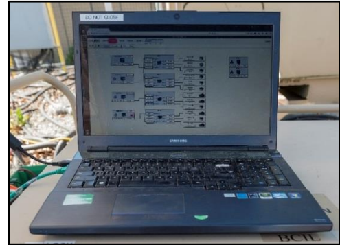
Figure C-25. Laptop to monitor power and status of the microgrid
