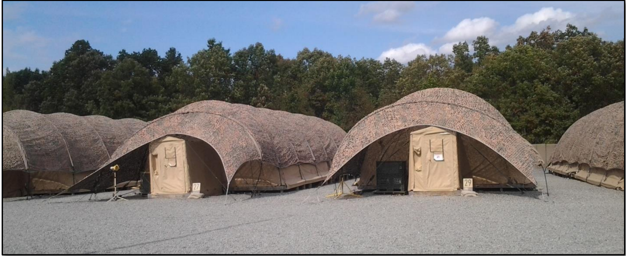
Figure 8: Air Supported Shelter (external view)
