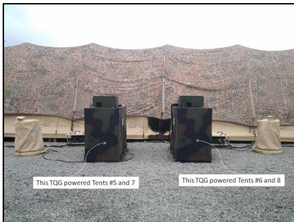
Figure 9: TQGs Powering South Camp
