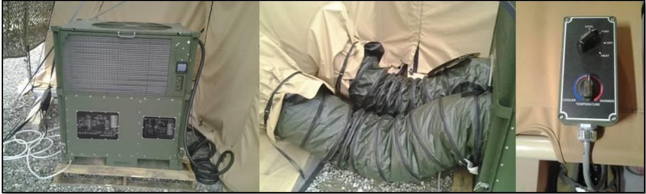
Figure 14: IECU, Ductwork, and Potentiometer
