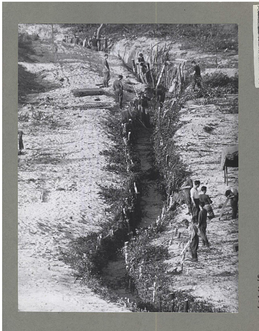
Figure 1-4: Berlin, Germany (E): A Ditch, Reminiscent of World War I Trenches, Runs Along the Edge of the “Death Strip” in the Rudow District of East Berlin. The communist evacuated residents and razed buildings in the strip to provide border guards with a clear field of fire at West Germans attempting to escape to freedom in the West. Source: USIS Bad Godesberg/H-38946. U.S. Information Agency 1982-10/1/1999. U.S. Information Agency. Press and Publication Service. Visual Services Branch. Photo Library. 1953 – 1977. (Predecessor). International Communications Agency. Press and Publication Service. Publication Division. 1978 – 1982. (Predecessor). Series: Master File Photographs of U.S. and Foreign Personalities, World Events, and American Economic, Social, and Cultural Life, ca. 1953 – ca. 1994. Unrestricted Use. Courtesy National Archives. Identifier: 6037811 Local Identifier: 306-PS-D-61-11909 Record Group 306. https://research.archives.gov/id/6037811 .
