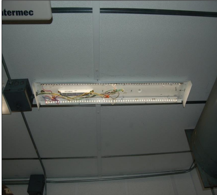
Figure 1-2. Eaton Metalux WNLED utility wraparound strip light luminaire without lens cover.
