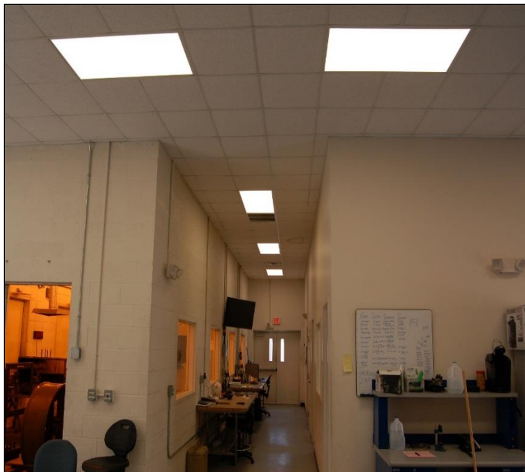
Figure 1-12. Upgraded Sylvania LEDVANCE lighting in Building 734.
