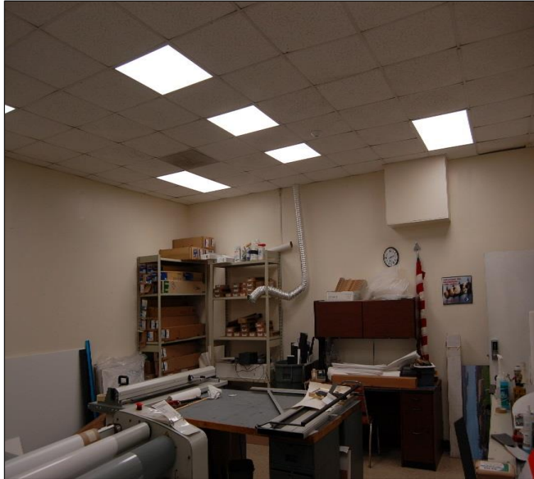
Figure 1-5. New LED Sylvania LEDVANCE luminaires in matting room of Building 322.
