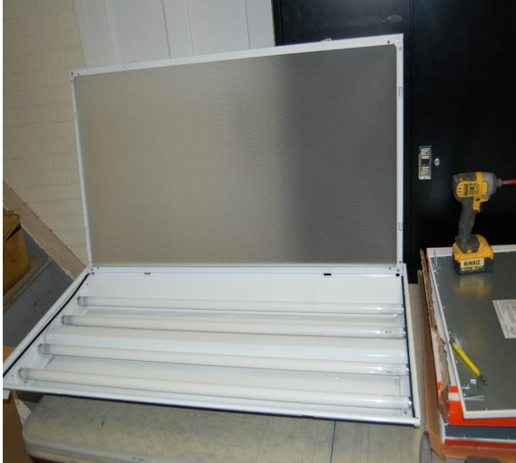
Figure 1-14. Typical 128 W. Fluorescent Lamp Fixture.
