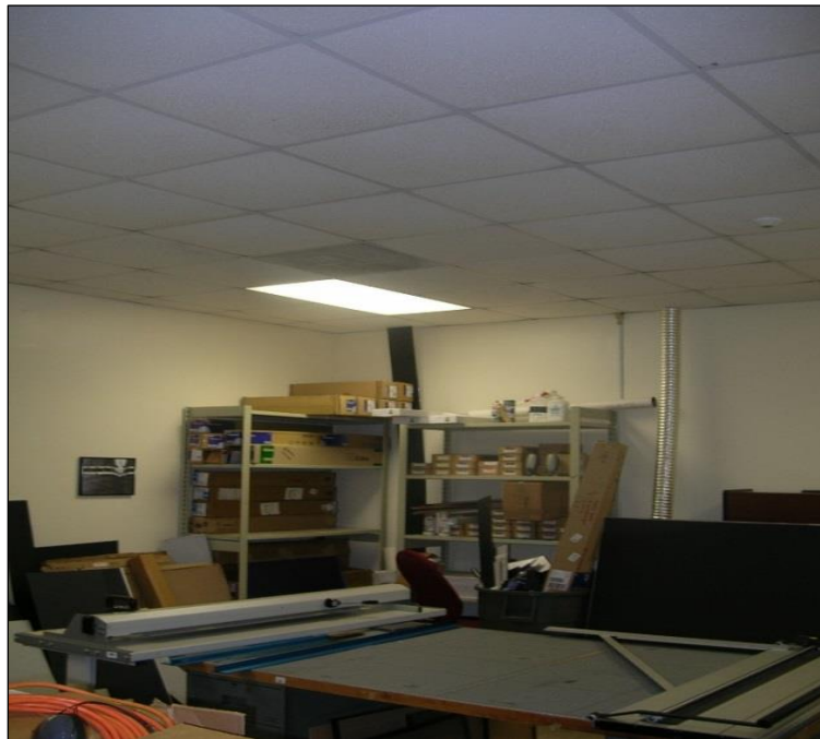
Figure 1-4. Inadequate fluorescent lighting in matting room of Building 322.
