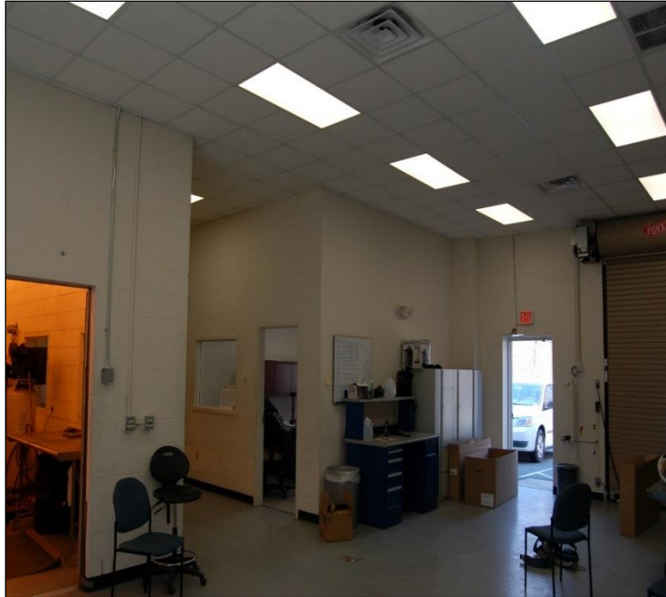
Figure 1-13. Upgraded Sylvania LEDVANCE LED lighting in Building 734.
