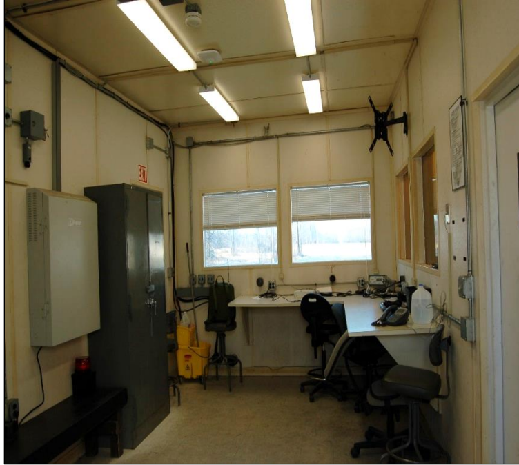
Figure 1-7. New LED Eaton Metalux wraparound luminaires installed in Building 726.
