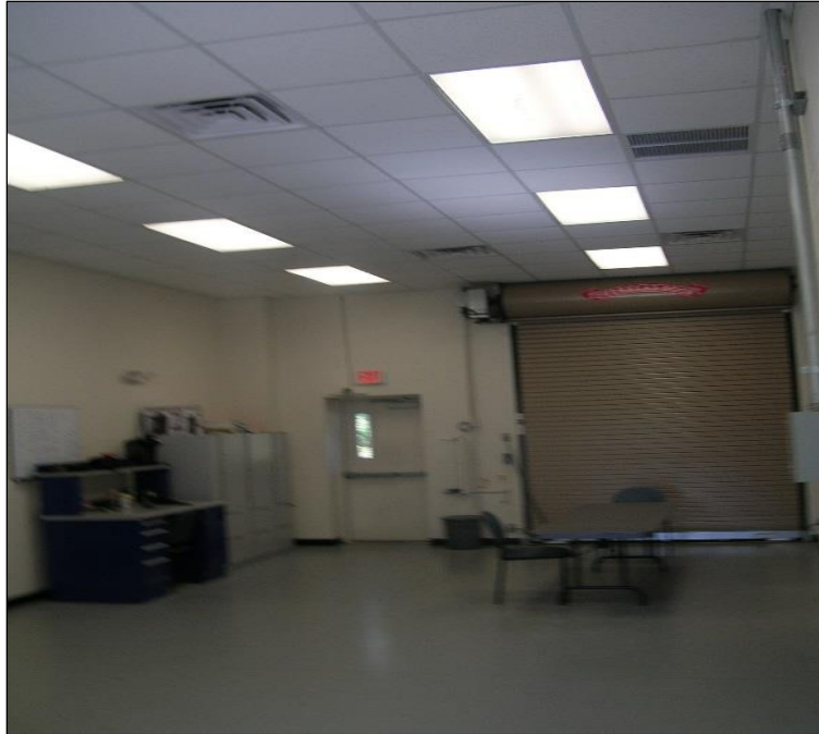
Figure 1-11. Fluorescent lighting in Building 734.
