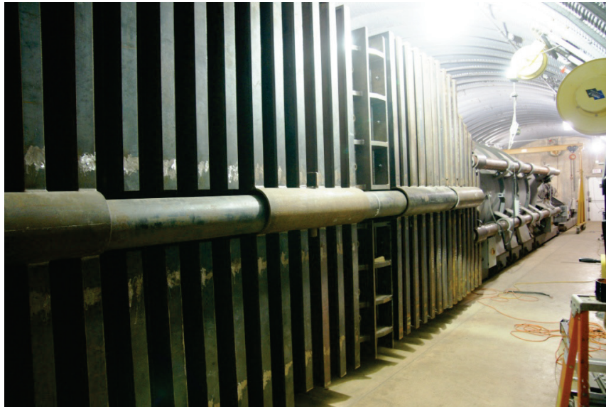
Figure 2. View from exterior of 8x8 configuration.
