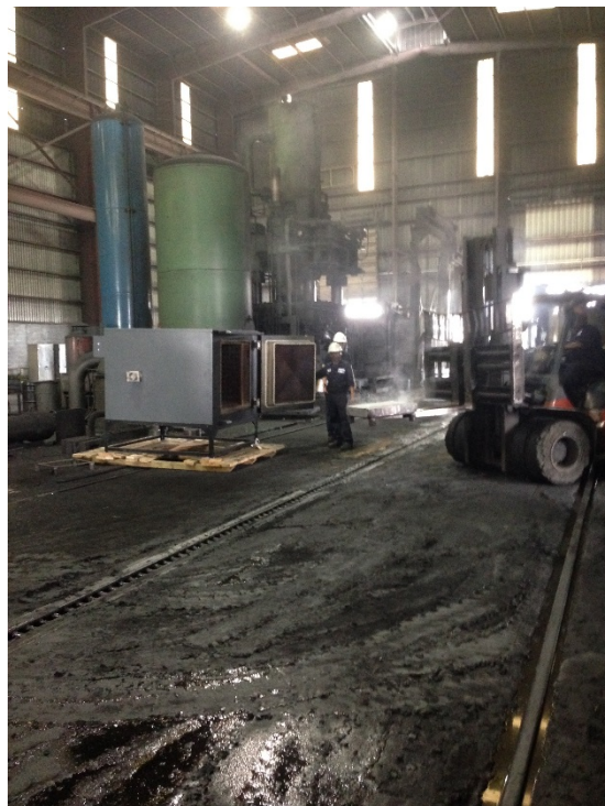
Fig. B-26 View of the box furnace used for preheating, solutionizing, and reheating the AA5083 billets
