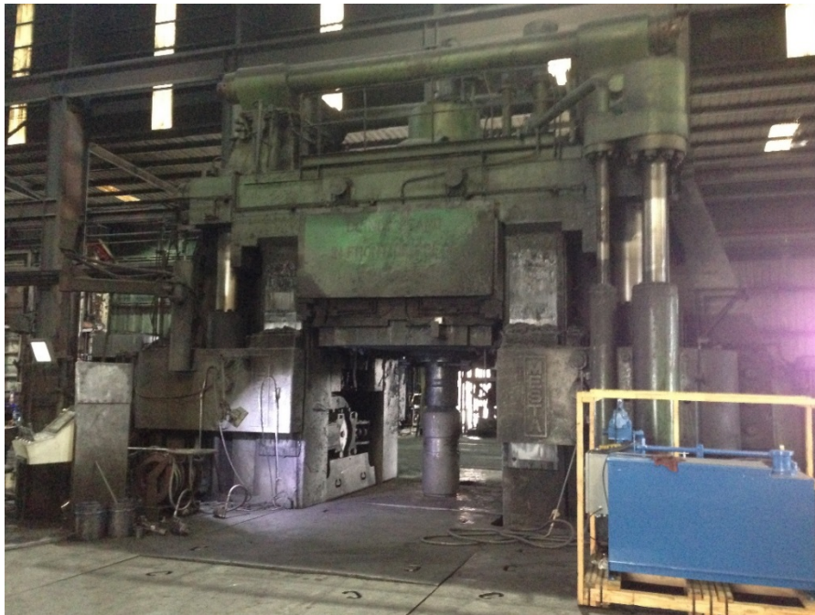
Fig. B-2 Front view of the Ellwood Texas Forge, Inc. (ETF) 11,000-ton forging press. On the right side of the press is the blue-colored auxiliary hydraulic power control unit for the ejection of the billet from the Engineered Performance Materials, Inc., (EPM) equal channel angular extrusion (ECAE) tool.
