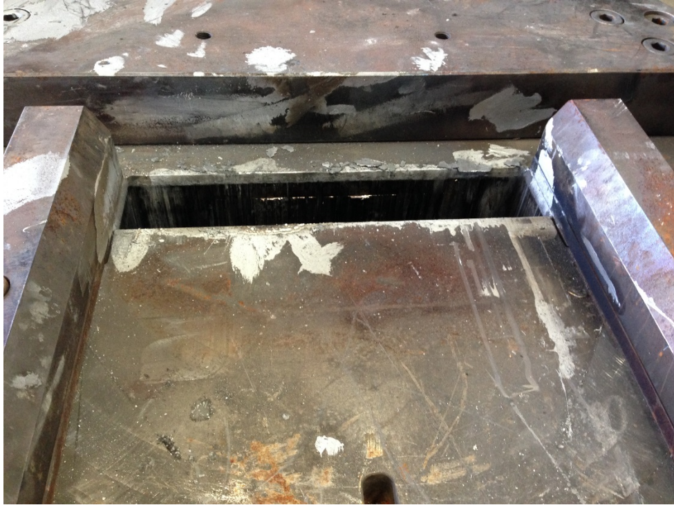
Fig. B-41 Top of the ring assembly showing slight damage to the input channel
