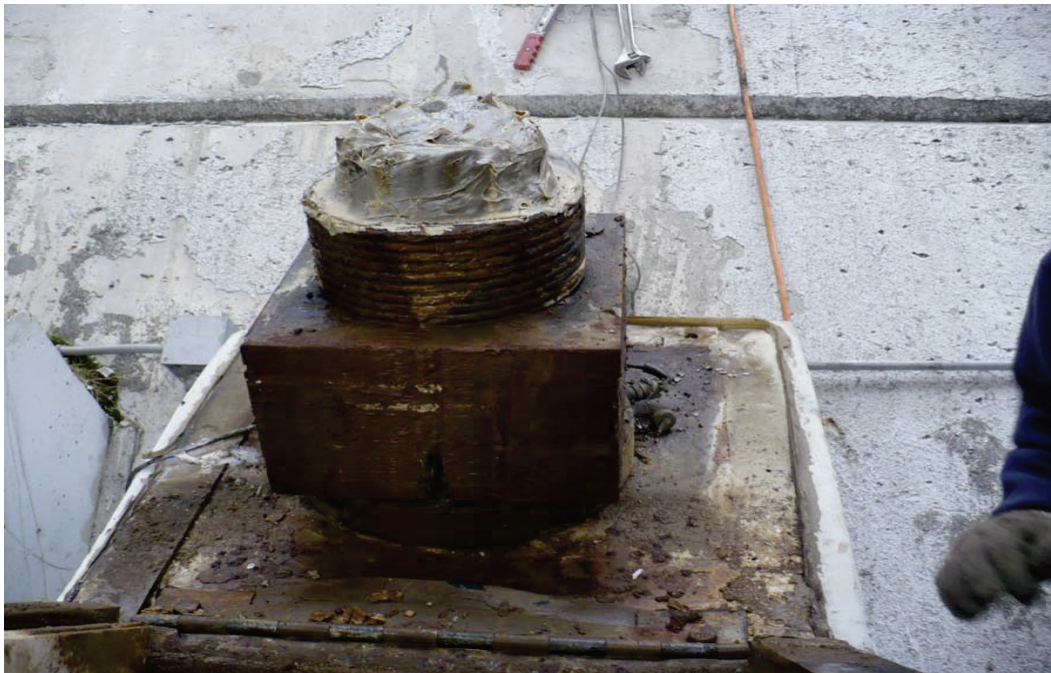
Figure 2.11. Freshly greased anchor head (Cornforth Consultants 2009).
