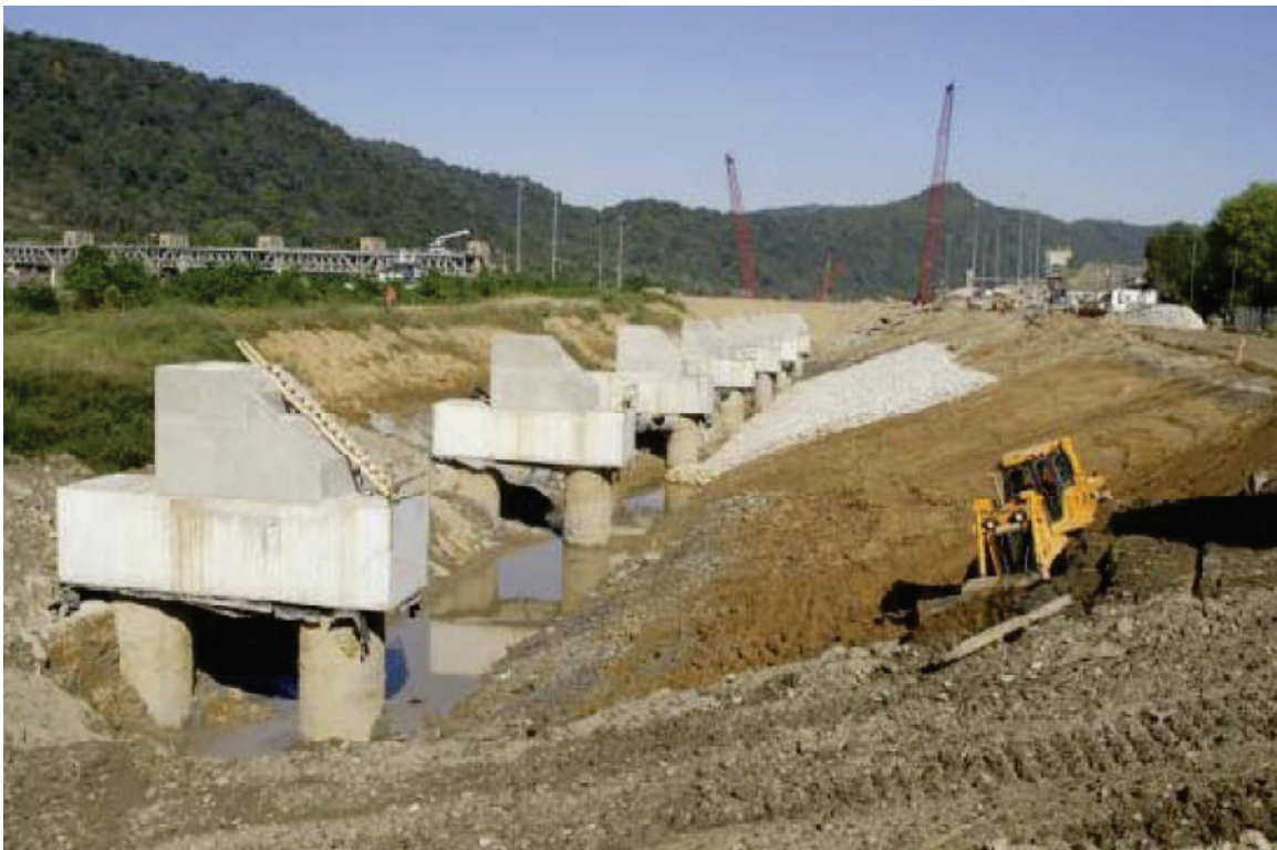
Figure 1.2. A set of two-DIP bents at Marmet approach wall to be used to support impact beam sections.
