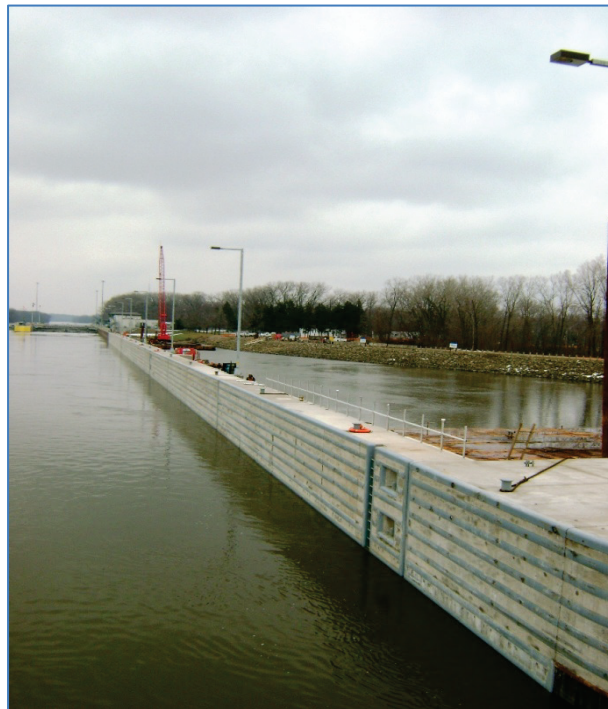
Figure 1.9. The finished pile-founded impact deck approach wall at Lock and Dam 3.
