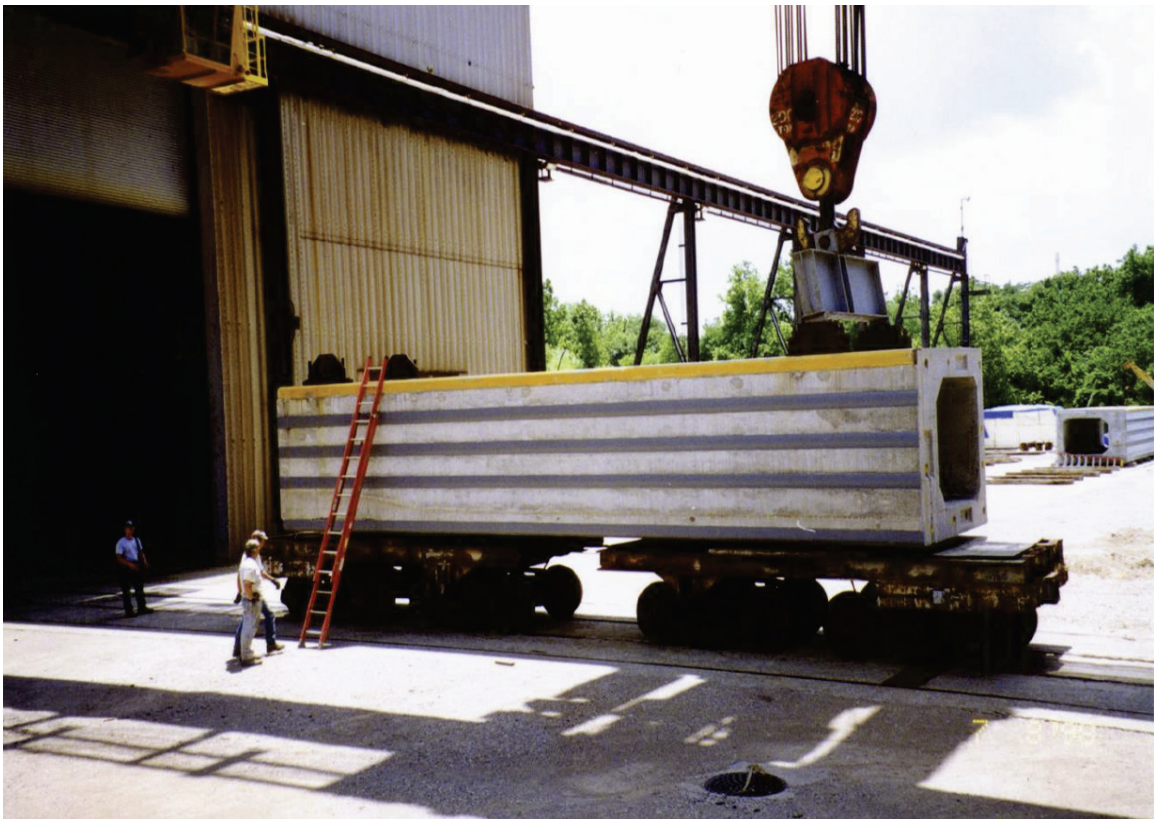
Figure 1.6. Another view of the impact beams used for the approach wall for Winfield Lock and Dam.
