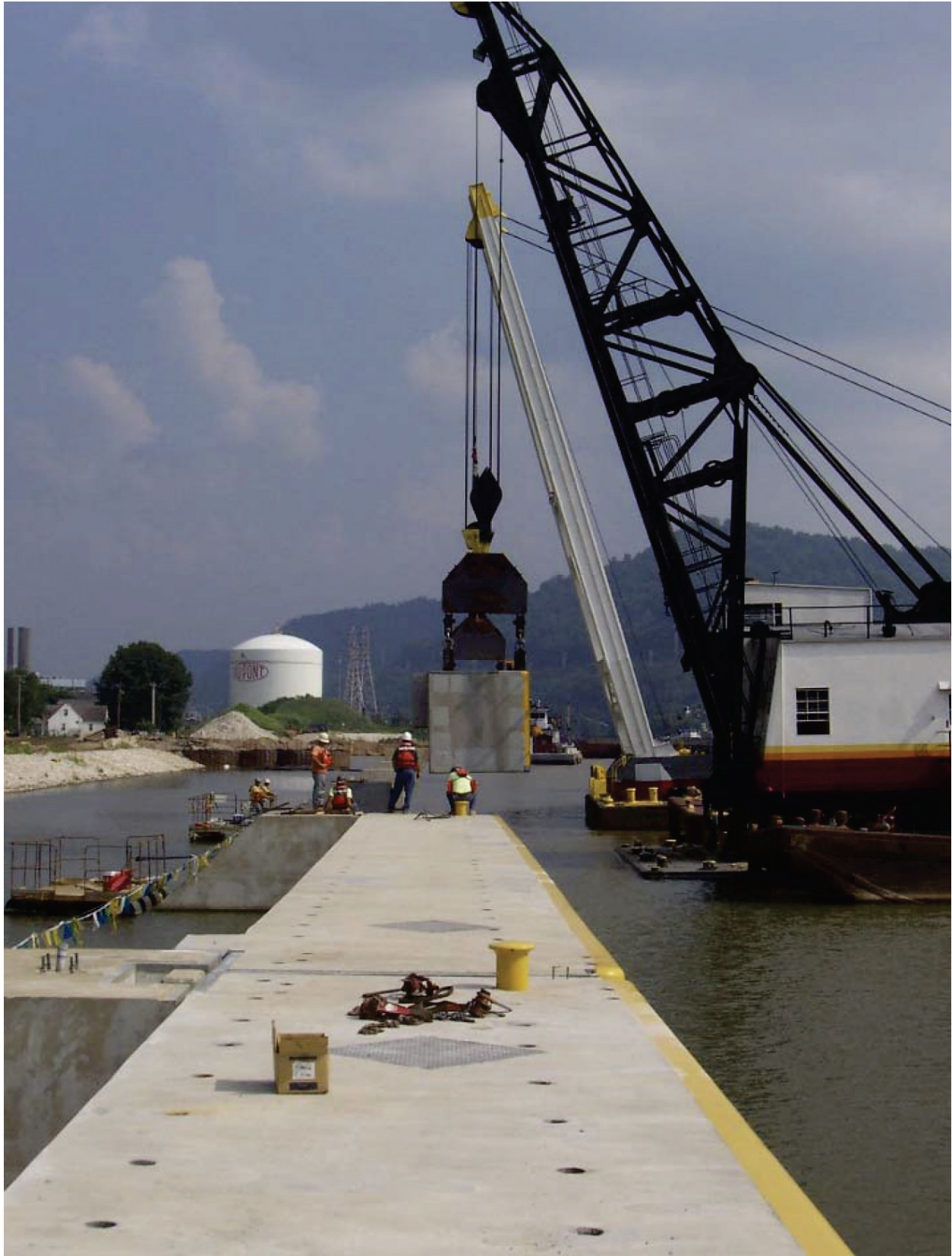
Figure 1.4. Installation of the Marmet approach wall impact beam sections.
