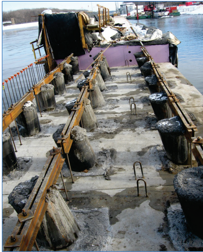
Figure 1.8. In-the-wet construction for the impact deck at Lock and Dam 3.
