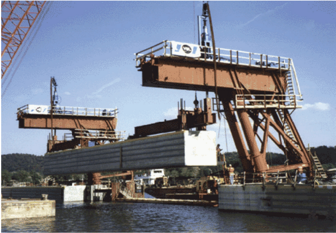
Figure 1.5. Installation of impact beam sections for the Winfield Lock and Dam approach walls.
