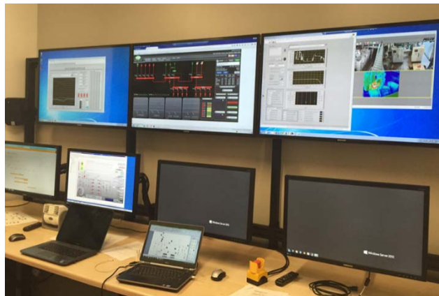
Figure 8. Power House Control Room
