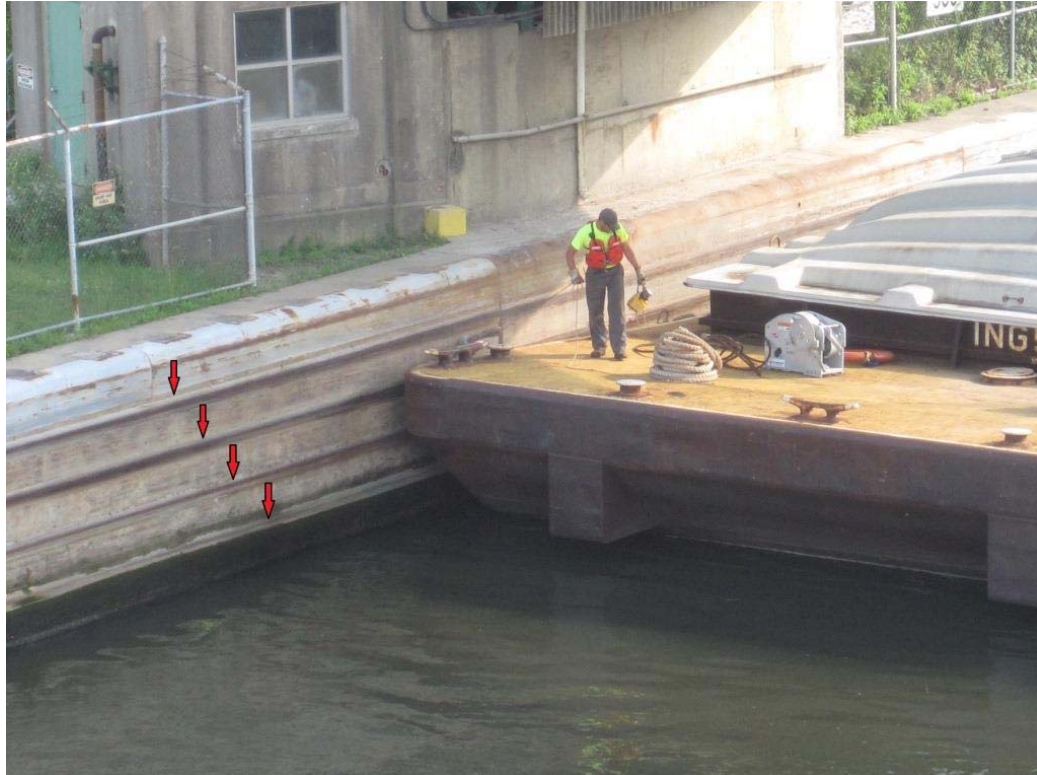
Figure 16. Close-up of rub-rails on LDB approach wall.
