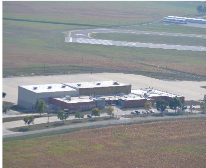
Figure 11. Waterloo Army Aviation Support Facility (AASF/ARMORY)
