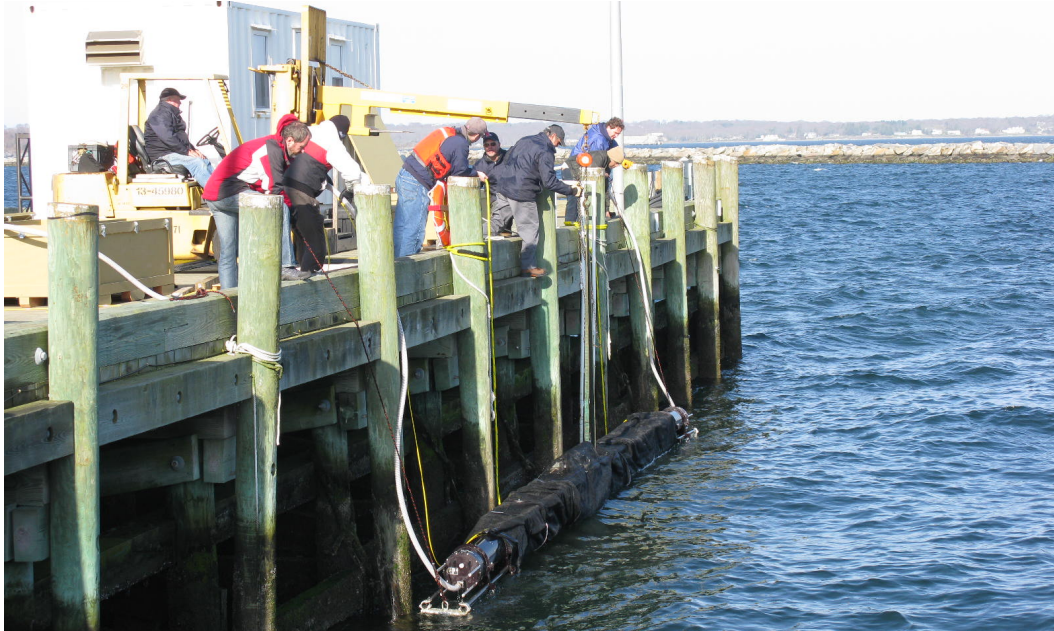
Figure 5. Truss assembly being removed from the water of Narragansett Bay, RI, on 31 March 2016.
