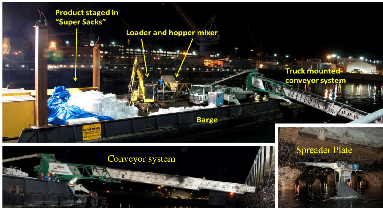
Figure 6. Amendment Application Method at Pier 7 Showing Barge Staged with "Super Sacks" of Product That Were Loaded into the Hopper Mixing Prior to Deployment with a Truck Mounted Conveyor System That Distributed the Product in the Berthing and Under Pier Areas. (PSNS&IMF Photo, approved for release; distribution is unlimited).
