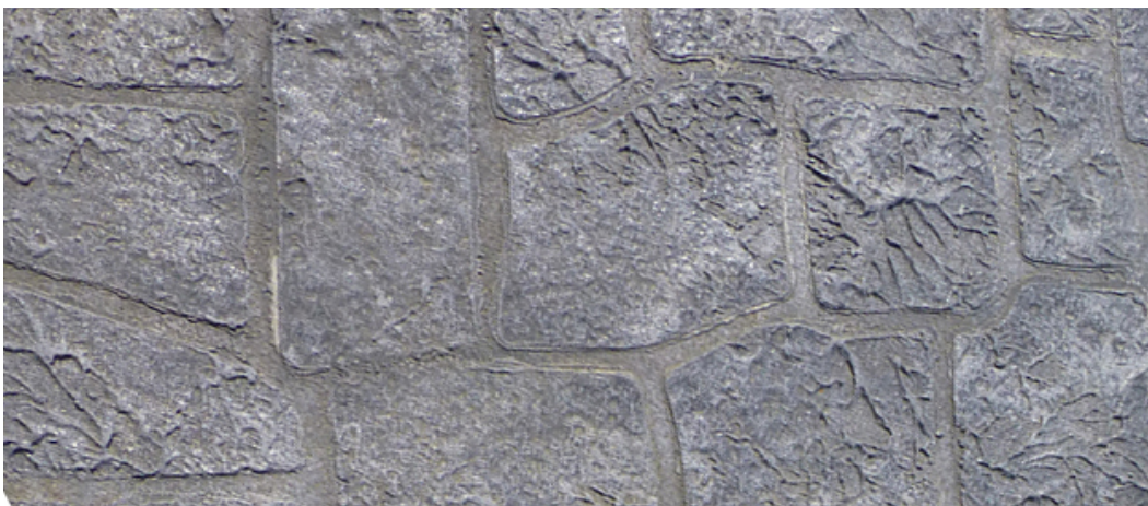
Figure 58. Looking down at the replacement stamped concrete on the former ceremonial drive (ERDC-CERL, 2015).
