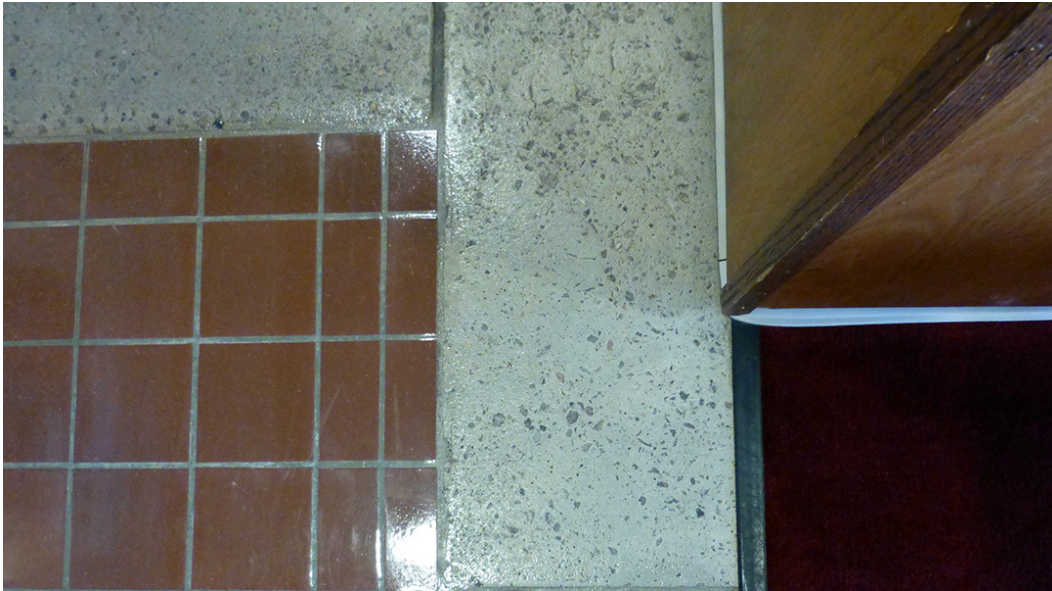
Figure 52. Looking down at the contrast between the original quarry tile and the concrete banding on the floor of the ceremonial lobby on the 4 th floor of Building 300 (ERDC-CERL, 2015).
