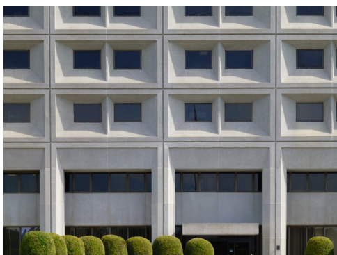
Precast architectural concrete window panels and column panels.
