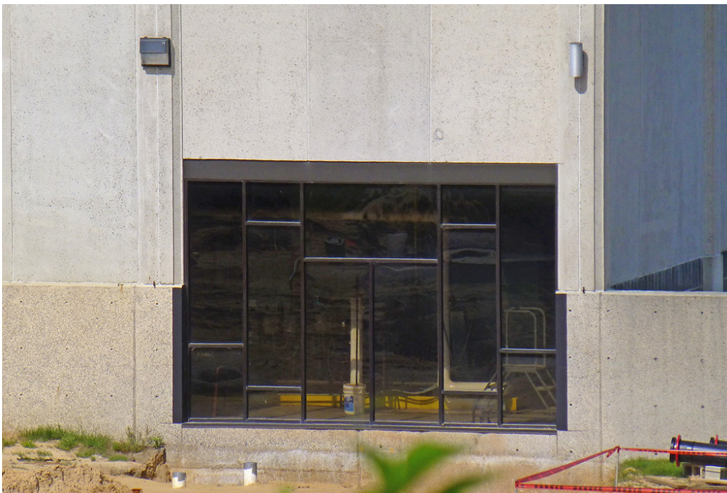
Figure 72. Detail of anodized bronze metal-framed windows on the east side of Building 310 (ERDC-CERL, 2015).
