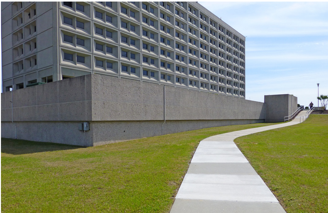
Figure 41. Detail of the southwest corner of Building 300, showing cast-in-place concrete plinth and sidewalk leading to Myer Plaza (ERDC-CERL, 2015).
