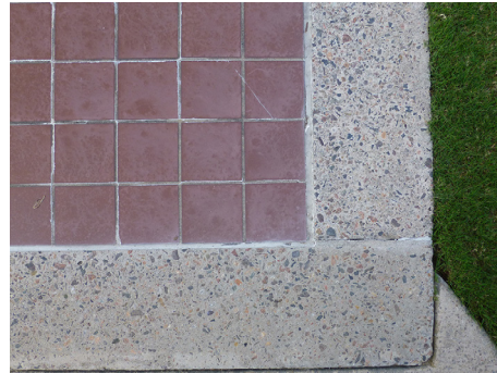
Quarry tile flooring with exposed concrete banding on the floor of the exterior colonnade.
