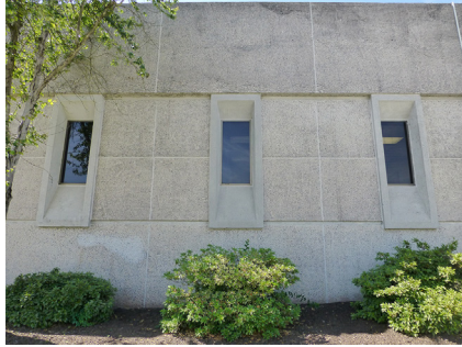
Combination of cast-in-place concrete walls and precast concrete window sections.
