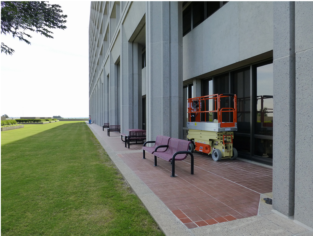
Figure 64. Looking east, showing the quarry tile floors and concrete banding on the floor of the colonnade (ERDC-CERL, 2015).
