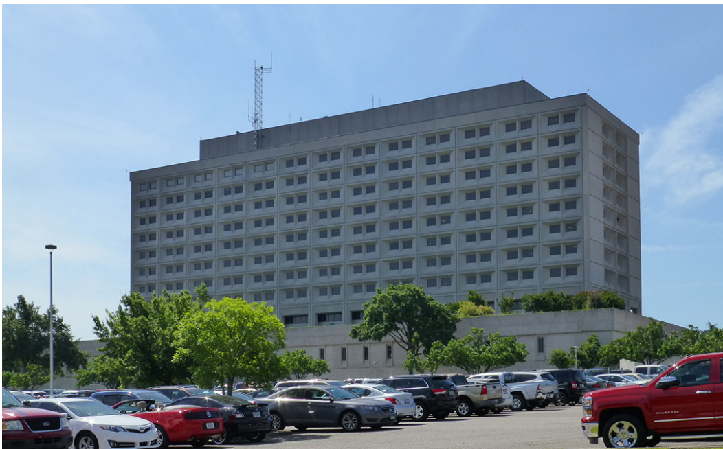
Figure 47. Northwest oblique of Building 300, showing the 2 nd and 3 rd floor cast-in-place concrete walls of the plinth (ERDC-CERL, 2015).
