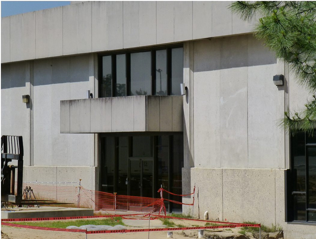
Figure 71. Detail of anodized-bronze metal-framed windows and doors at entrance on the east side of Building 310, with a concrete balcony above (ERDC-CERL, 2015).
