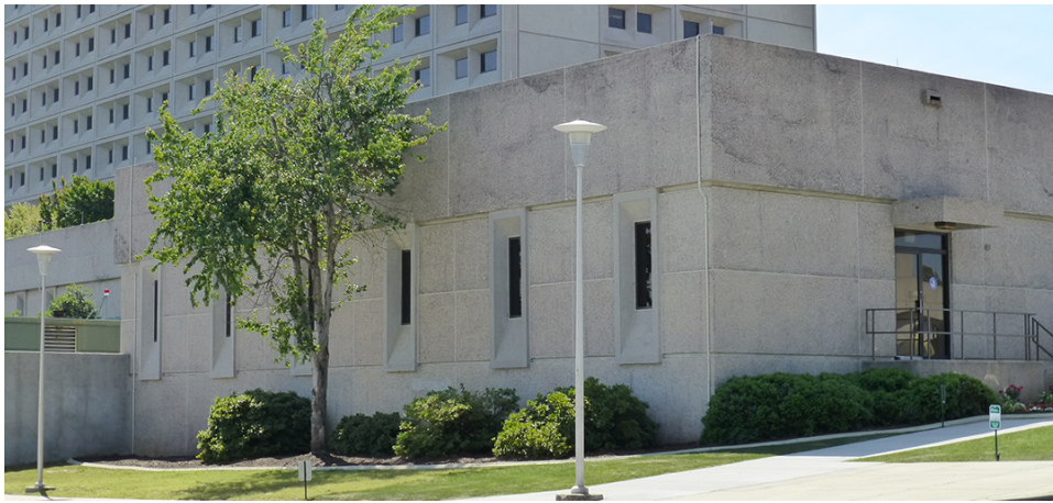
Combination of cast-in-place and precast concrete window sections
