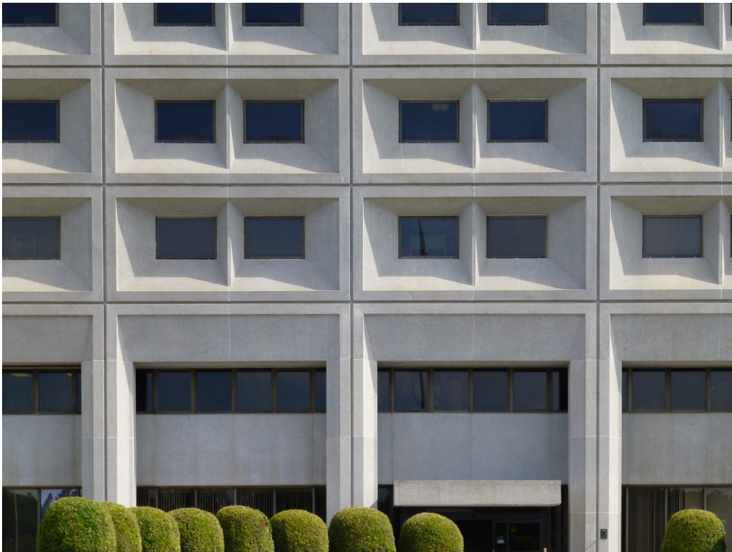
Figure 40. Detail of the south side of Building 300, showing precast concrete window panels and column panels (ERDC-CERL, 2015).
