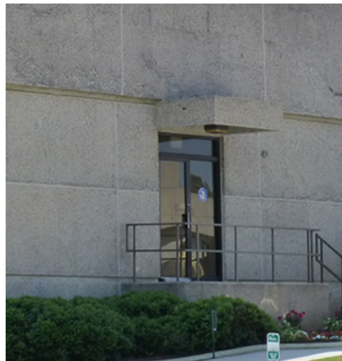
Concrete door canopy and anodized-bronze door frames.
