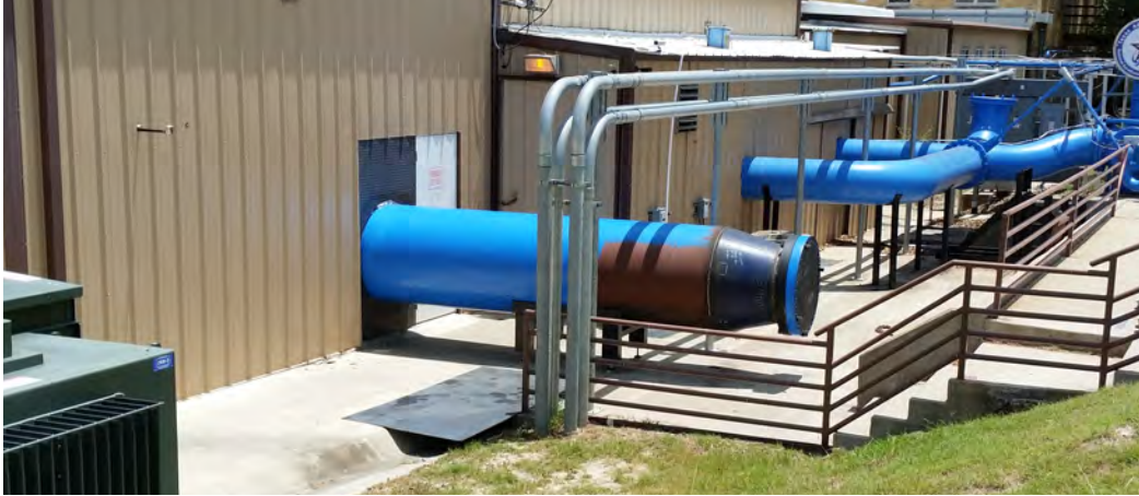
FIG. 25 Tailpipe during installation.
