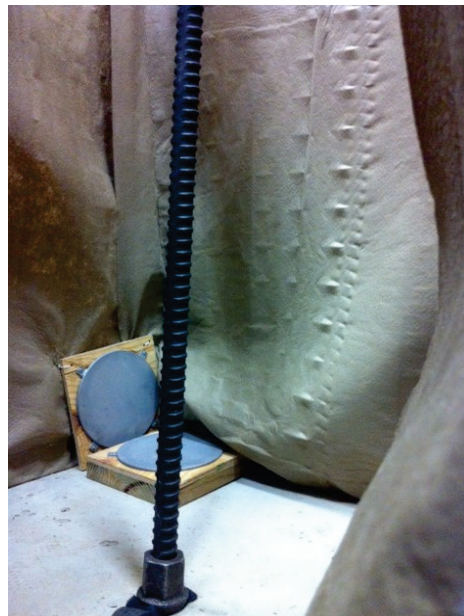
Figure 9. Interior of unfilled HESCO bastion showing threaded rod vertically penetrating the concrete pad.
