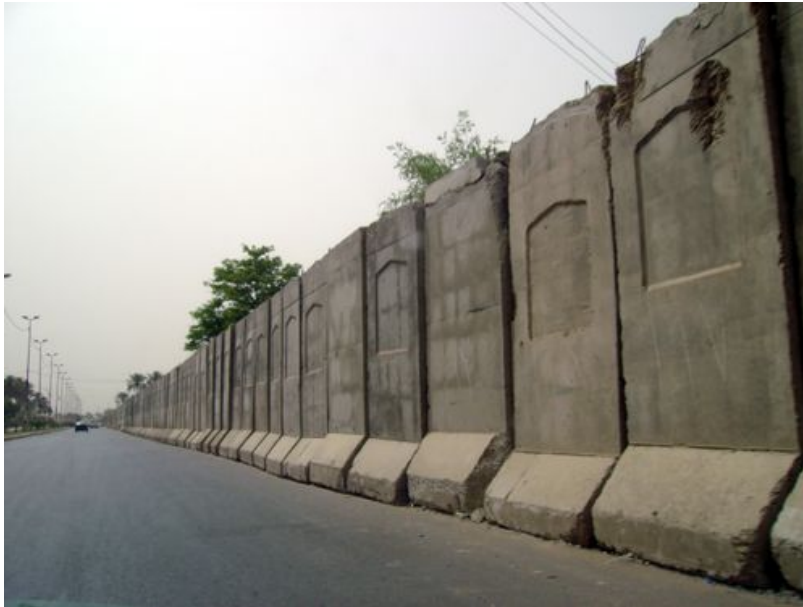
Figure 5.3: An Example of a Traditional 8 Foot Tall Cast Concrete Blast Wall in Baghdad, Iraq. Source: [100]
