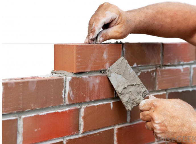
Figure 5.1: Traditional Brick Laying Technique. Source: [84]
