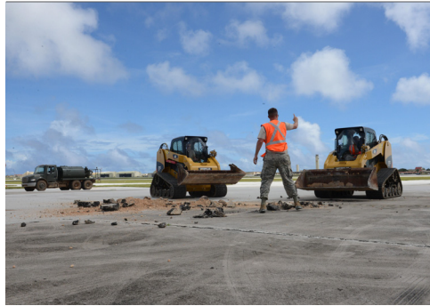
Airmen clear debris during airfield damage repair training at Andersen Air Force Base, Guam. Rapid runway repair can help a base sustain air operations while under attack.
