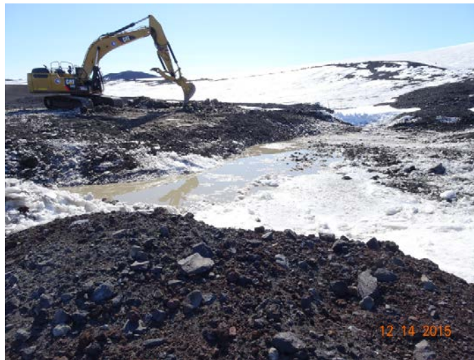
Figure 14. Digging the secondary pond.
