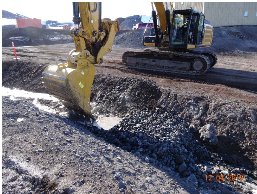
Figure 11. Rock weir using the 2 to 8 in. rocks. The excavator created a sump upstream of the weir.
