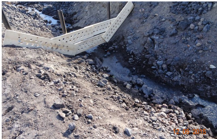
Figure 9. Prototype anchored wooden weir tested along the channel on Gasline Alley.
