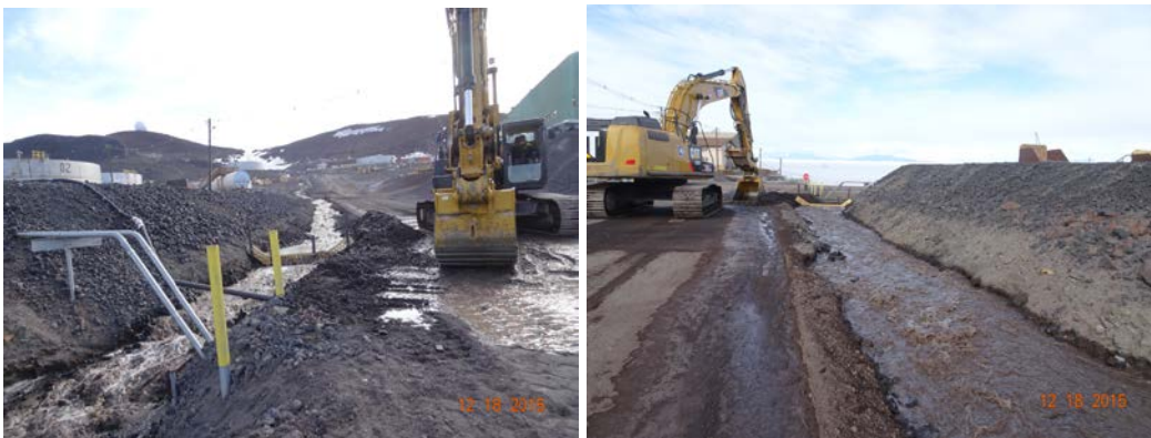
Figure 23. Extreme runoff around 9 a.m. in the drainage channel along Gasoline Alley. The left image shows downstream, and the right image shows upstream of the weir.
