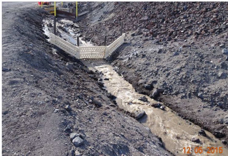
Figure 8. Prototype anchored wooden weir tested along the main channel.
