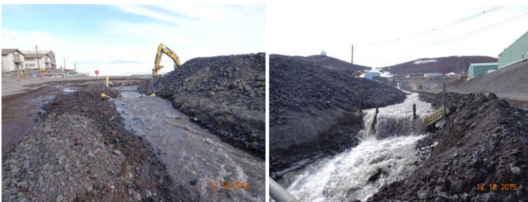
Figure 24. Extreme runoff around 3 p.m. in the drainage channel along Gasoline Alley. The left image shows upstream, and the right image shows downstream of the weir.
