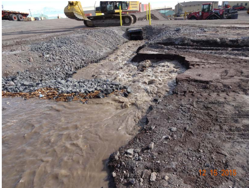
Figure 22. Example of a collapsed bank adjacent to the weir when excessive amounts of runoff occurred.
