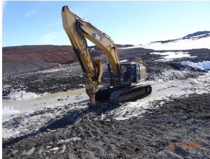
Figure 13. Digging the primary pond at Pond 3C.
