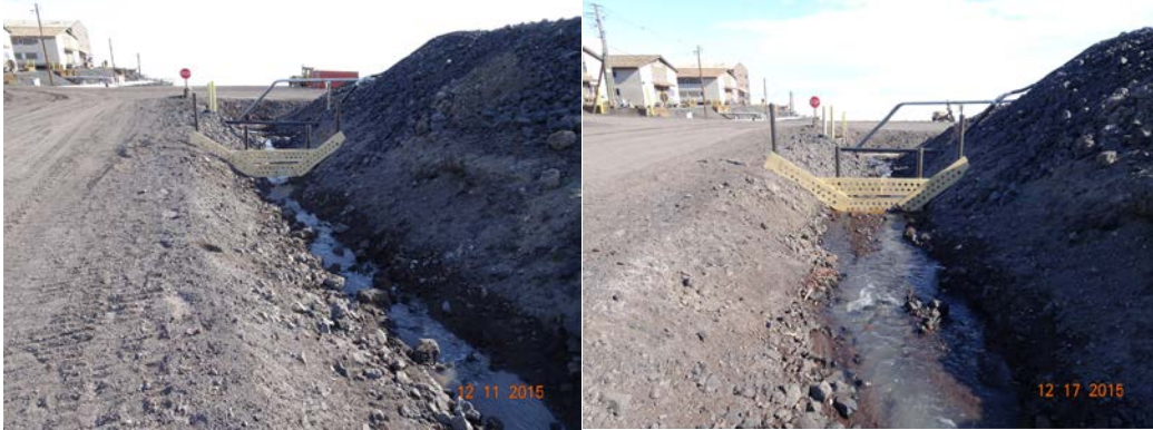
Figure 20. Water stage and sediments upstream of the anchored wooden weir.
