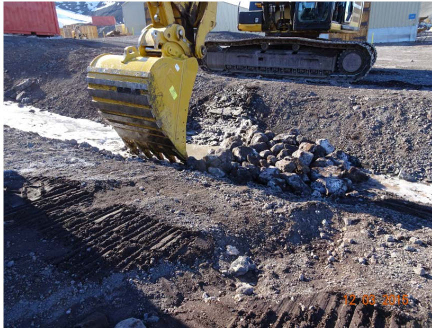
Figure 12. Rock weir using 8 to 12 in. rock sizes with a sump upstream of the weir.
