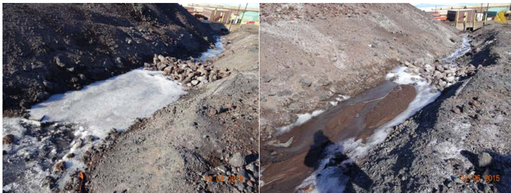
Figure 18. Water stage and sediments upstream of the rock weirs during light flow.
