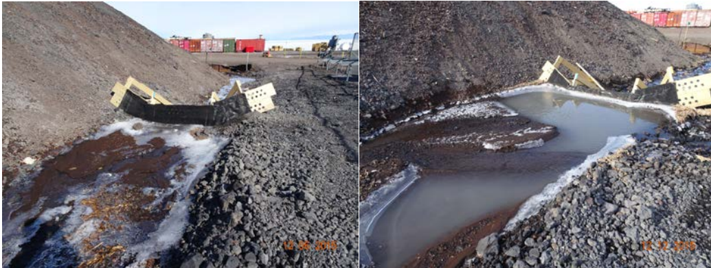
Figure 19. Water stage and sediments upstream of the unanchored wooden weir.
