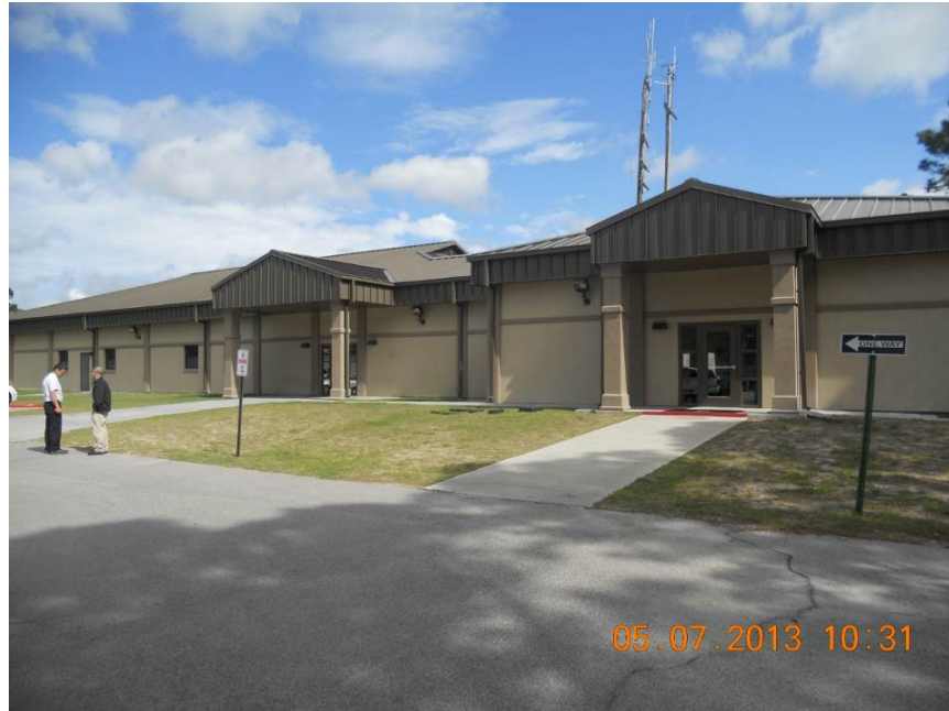
Figure 5.1. Building 584, MCAS, Beaufort, SC.
