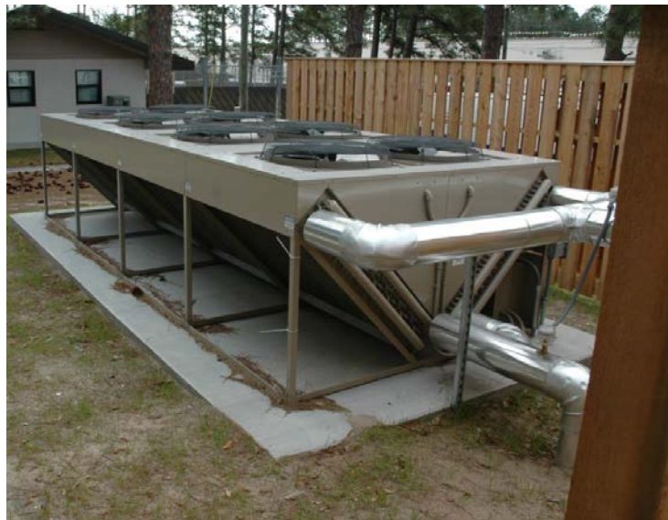
Figure 5.5. Dry Fluid Cooler Installed at Building 584.
