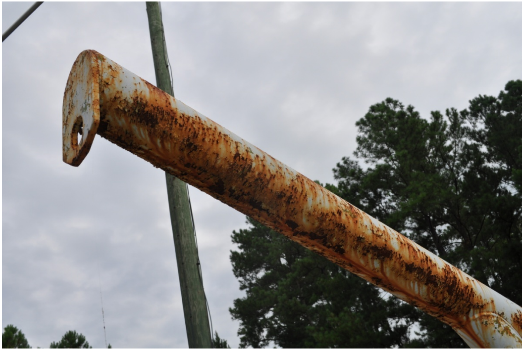
Figure 2. Corroded jib crane.
