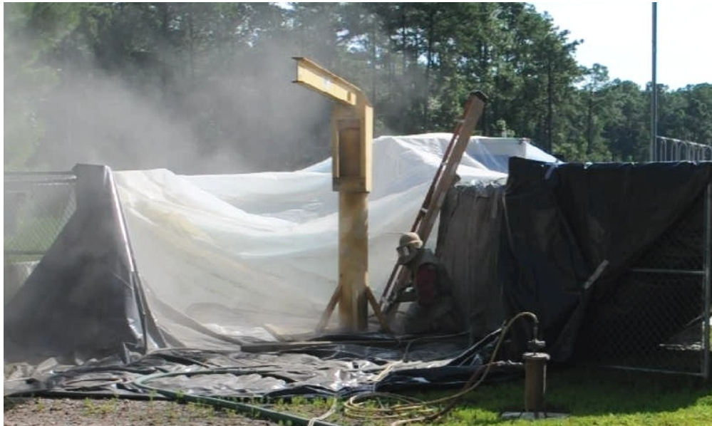
Figure 5. Abrasive blasting of jib crane.
