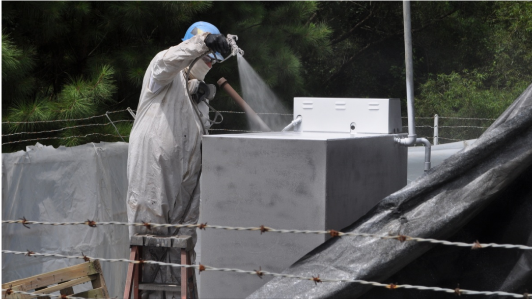
Figure 6. Applying epoxy barrier coat.
