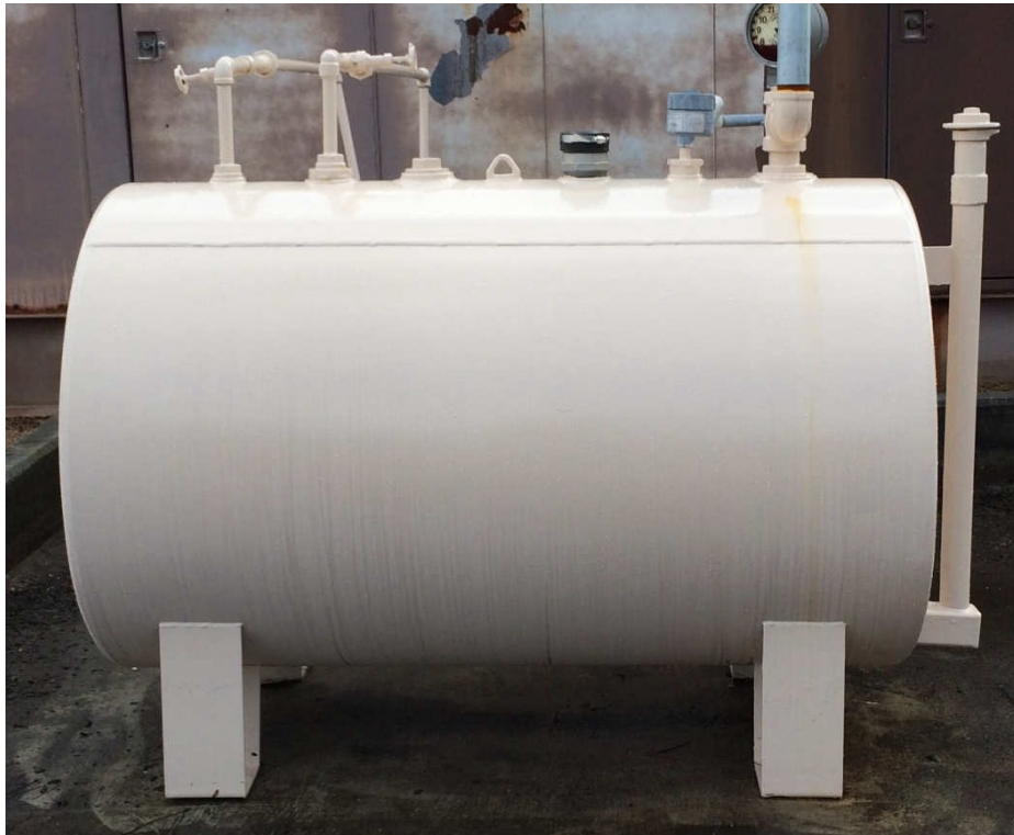
Figure A12. Lift Station 9 fuel tank after 6 months of exposure.
