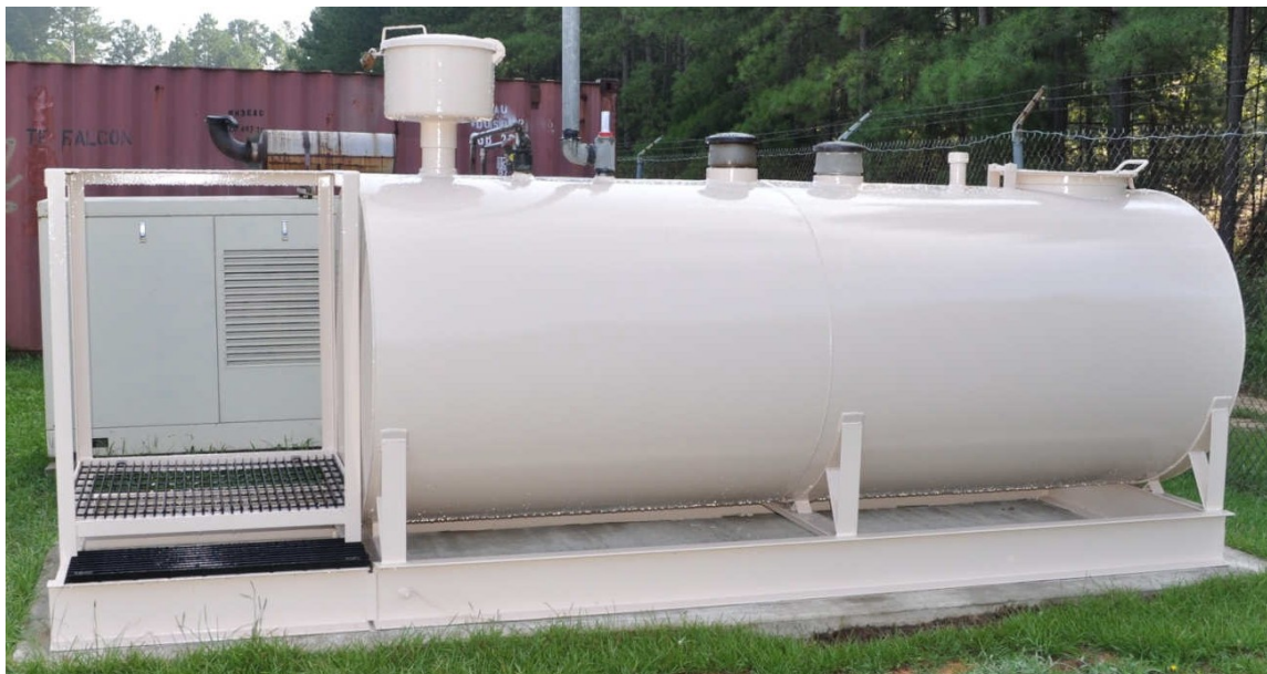
Figure A13. Lift Station 7 fuel tank after 6 months of exposure.
