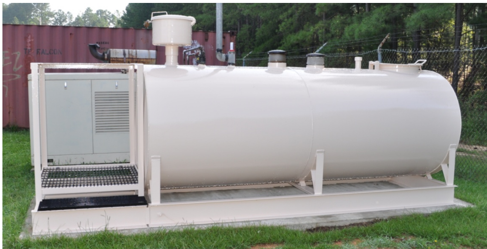
Figure 7. Finished fuel storage tank at Lift Station 7.
