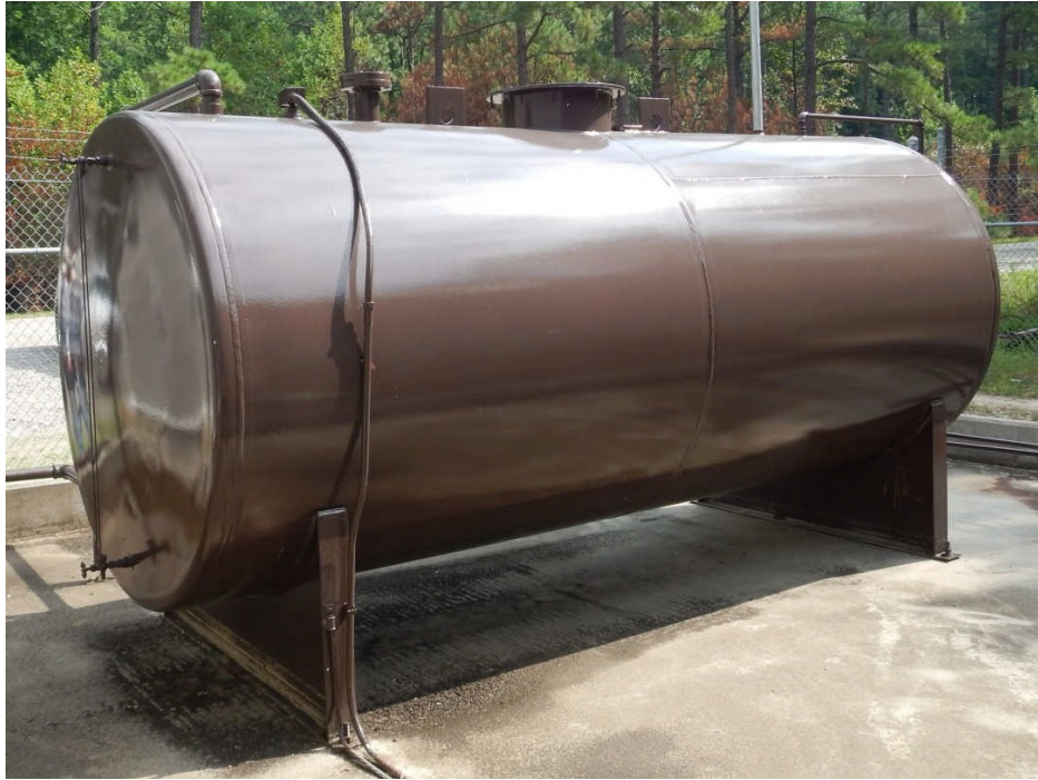
Figure B4. Lift Station 1 fuel tank after 12 months of exposure.
