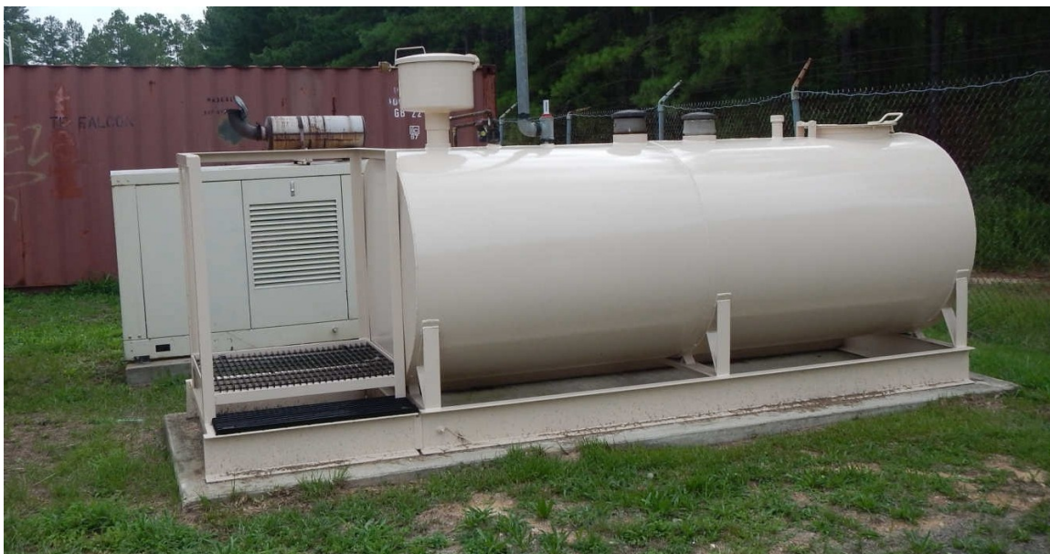
Figure B6. Lift Station 7 fuel tank after 12 months of exposure.
