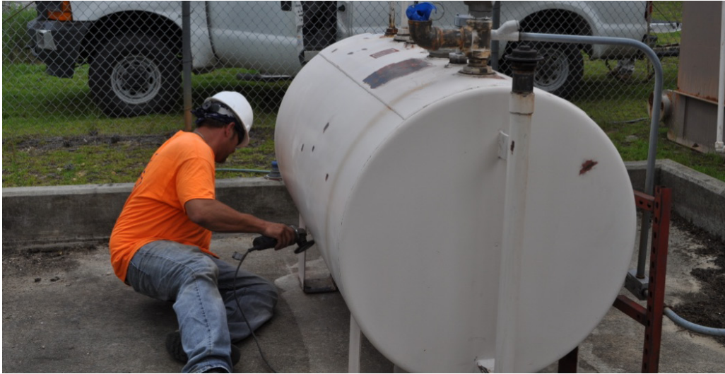
Figure 4. Hand tool corrosion removal.
