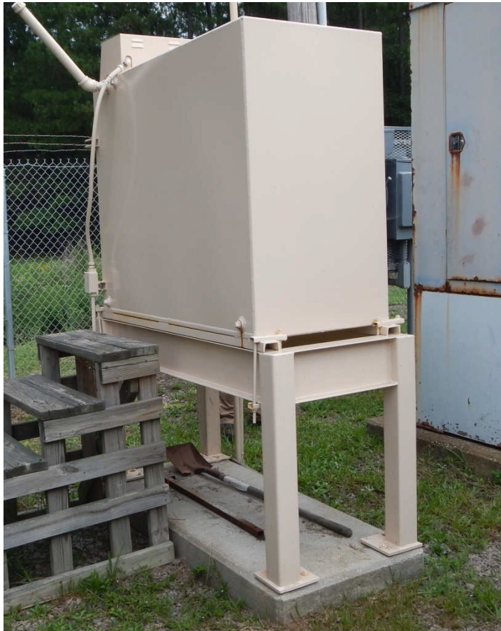
Figure B7. Lift Station 8 fuel tank after 12 months of exposure.
