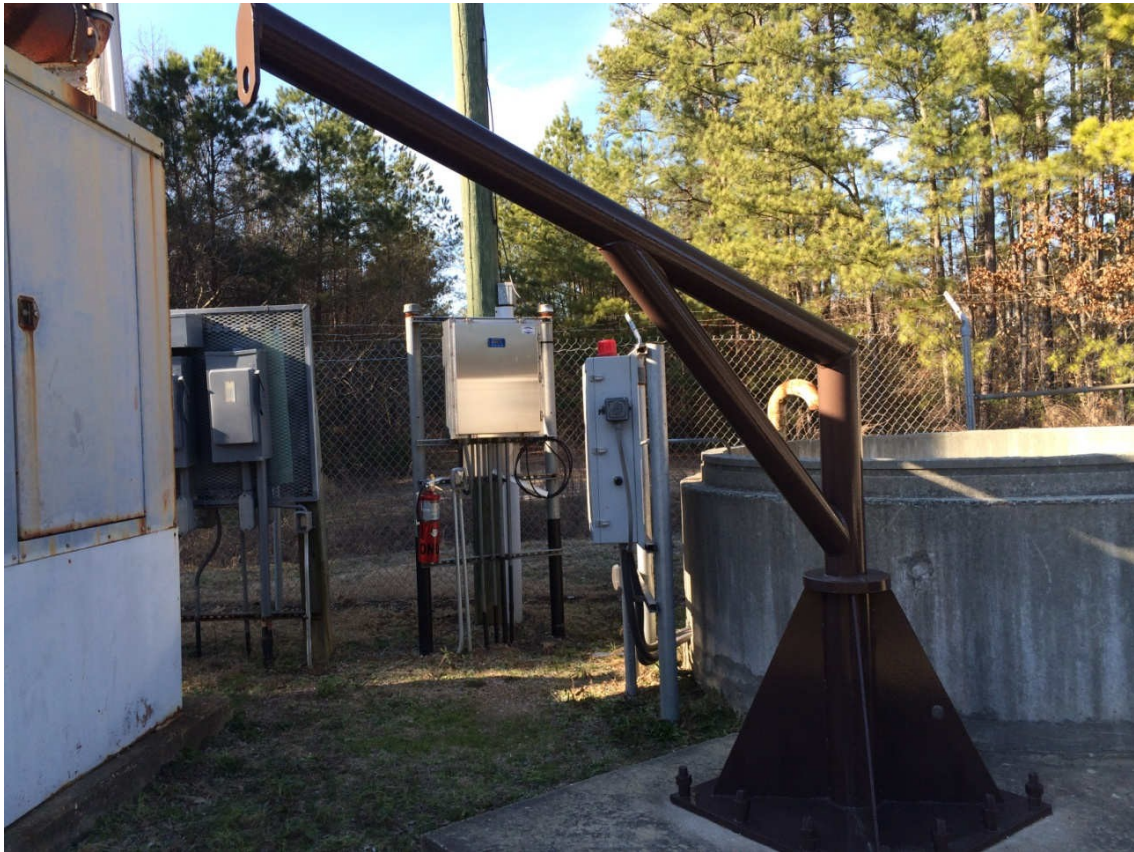
Figure A7. Lift Station 8 crane after 6 months of exposure.
