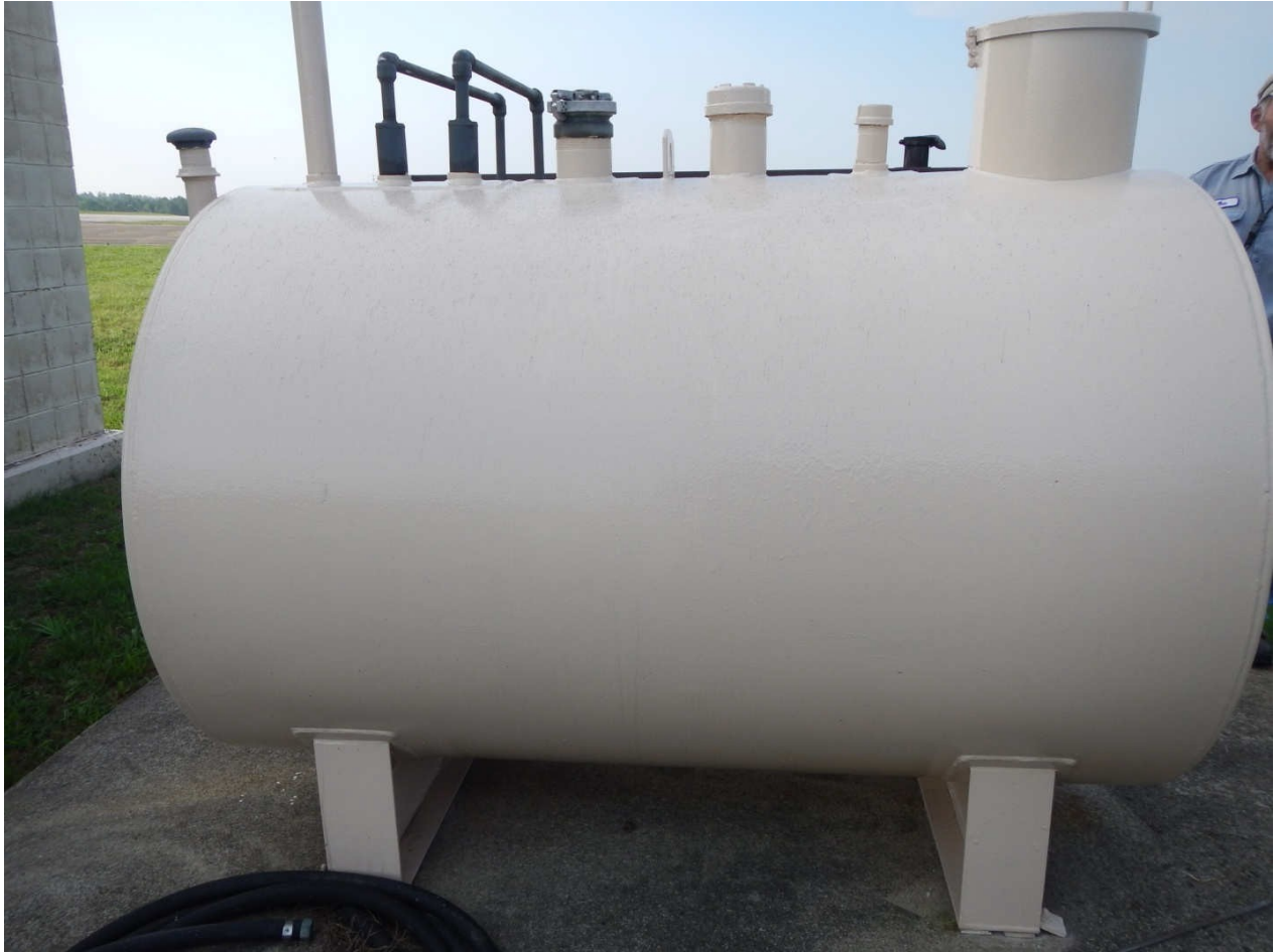
Figure B5. Lift Station 6 fuel tank after 12 months of exposure.
