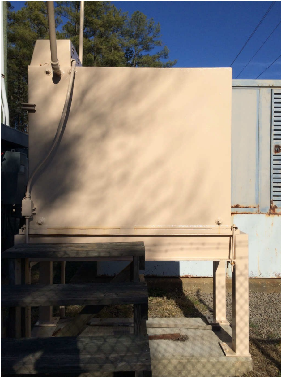
Figure A6. Lift Station 8 fuel tank after 6 months of exposure.
