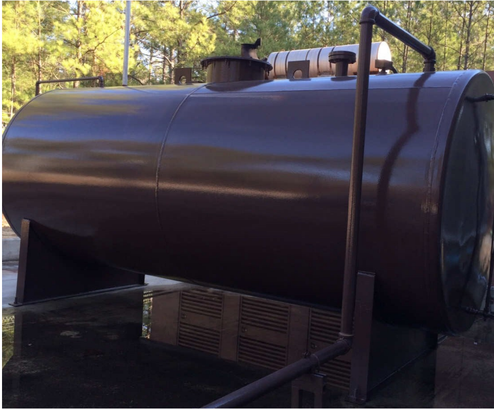
Figure A10. Lift Station 1 fuel tank after 6 months of exposure.
