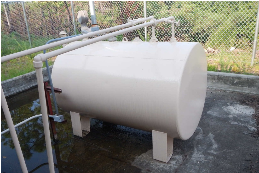
Figure B9. Lift Station 9 fuel storage tank after 12 months of exposure.
