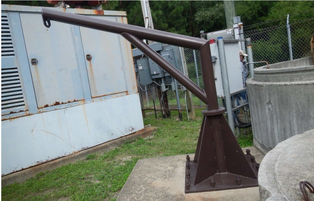
Figure B8. Lift Station 8 jib crane after 12 months of exposure.
