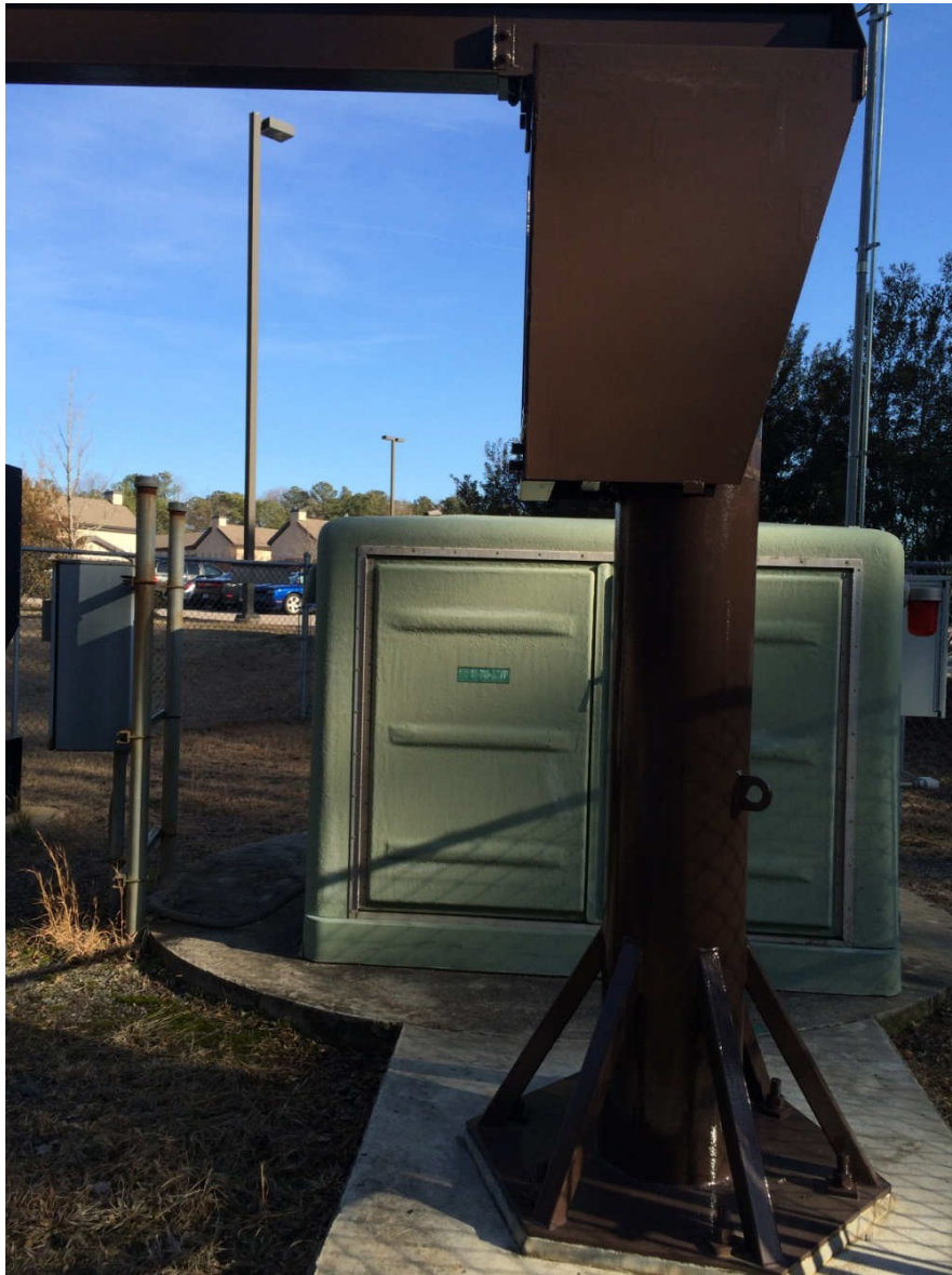
Figure A9. Lift Station 11 crane after 6 months of exposure.
