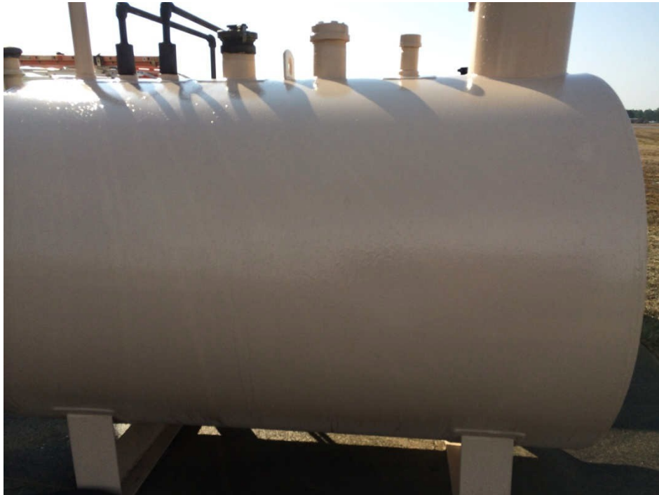
Figure A11. Lift Station 6 fuel tank after 6 months of exposure.
