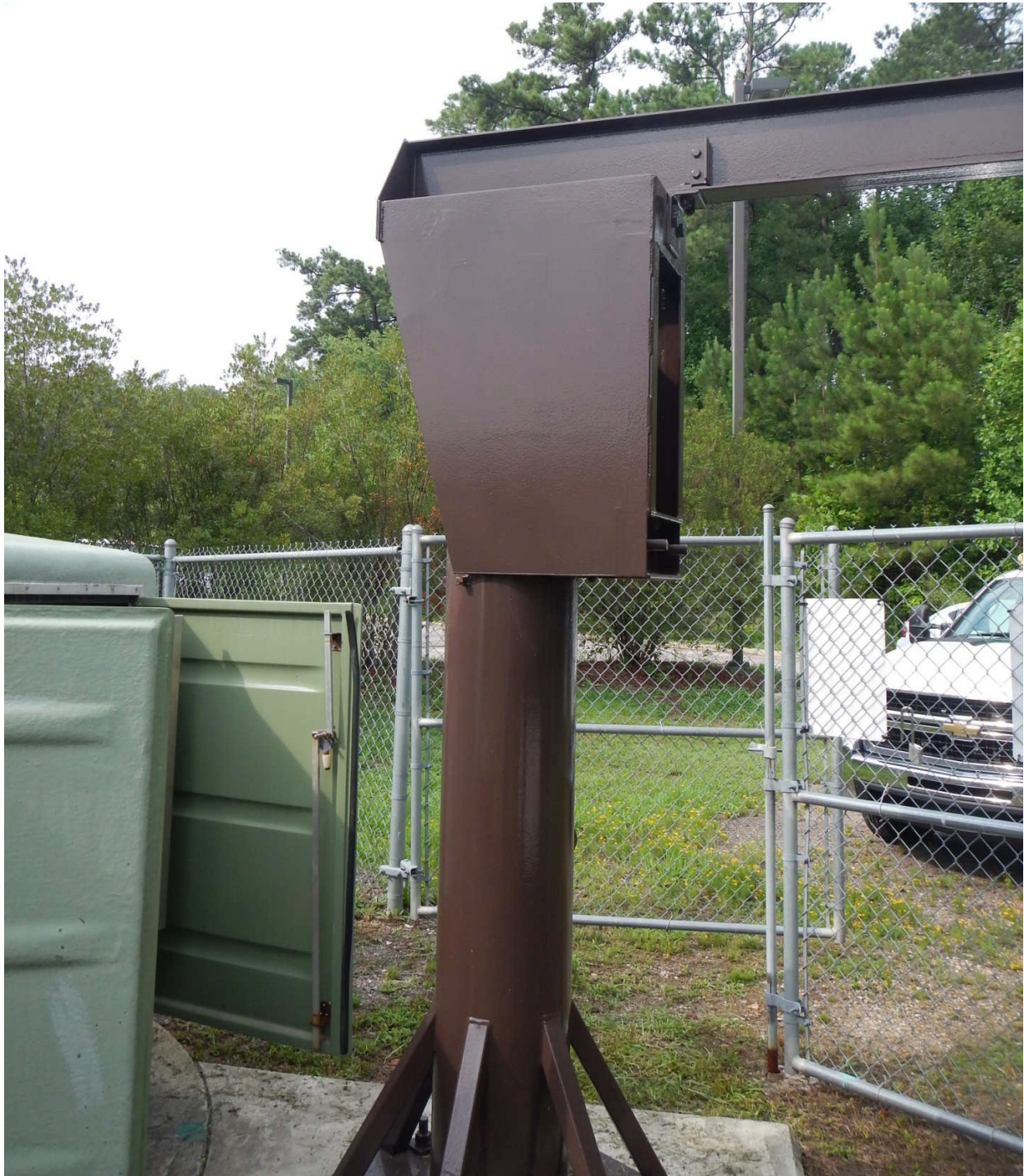
Figure B10. Lift Station 11 jib crane after 12 months of exposure.
