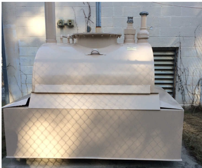
Figure A8. Lift Station C2517 fuel tank after 6 months of exposure.
