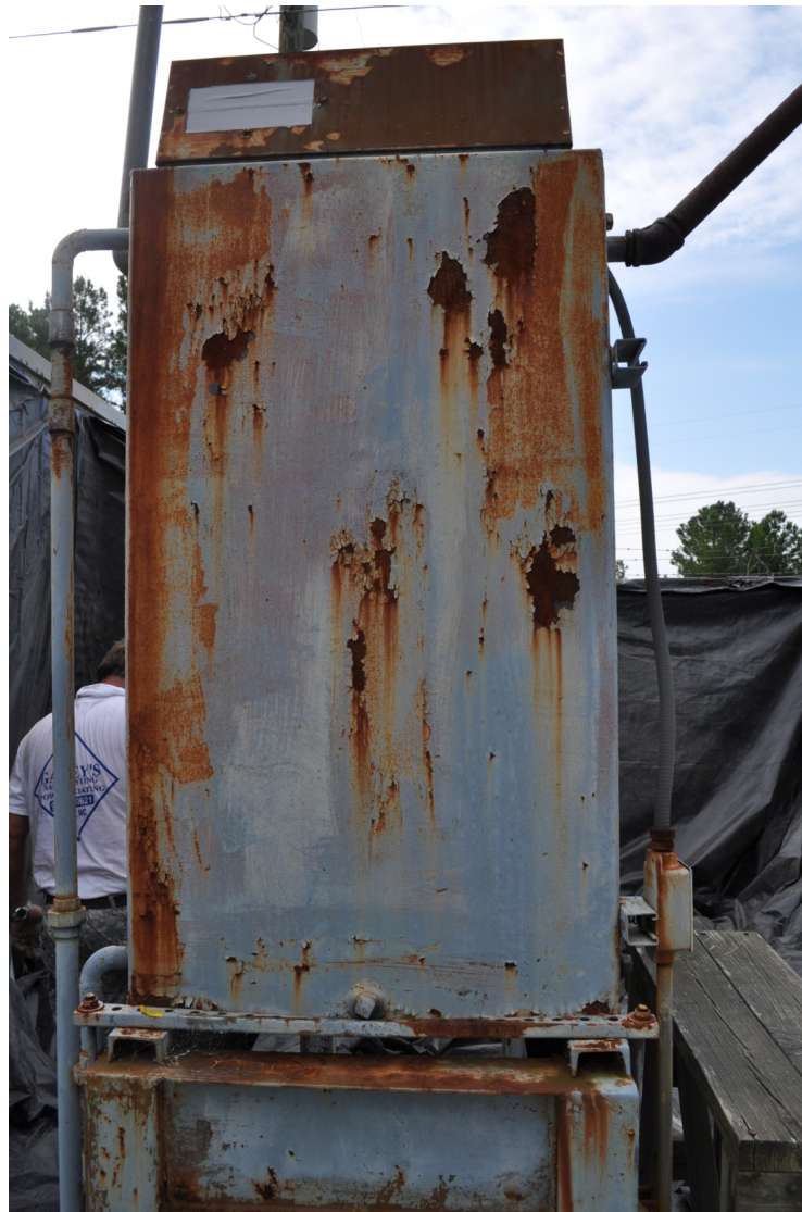
Figure 1. Corroded fuel storage tank.
