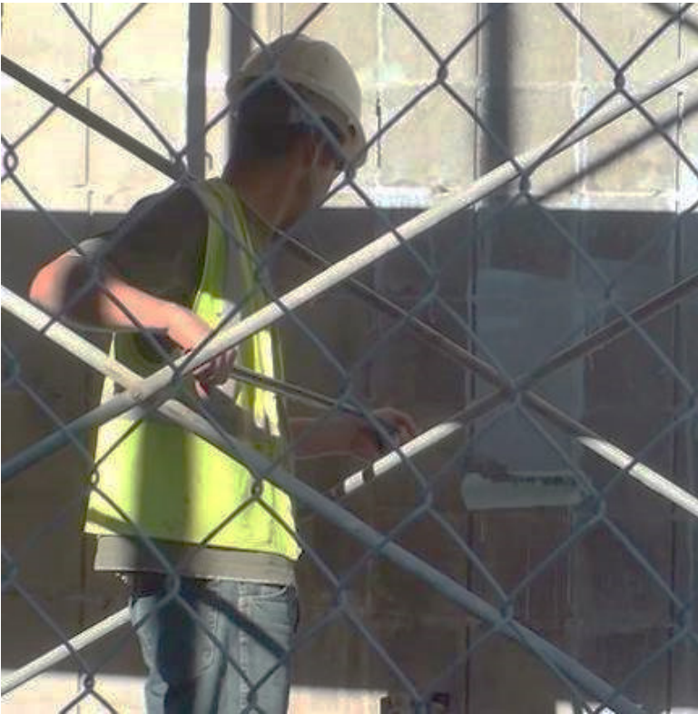
Figure 6. Application of adhesive.
