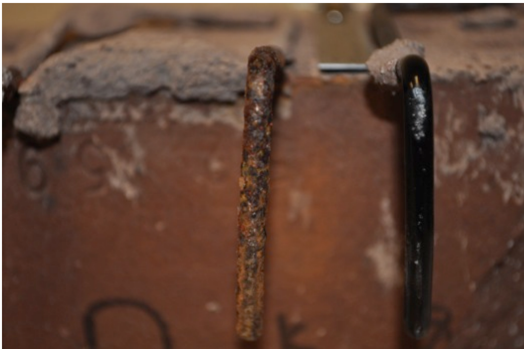
Figure 35. Inspection of the exterior part of the galvanized (left) and vitreous coated (right) pintle after 18 months of exposure at Duck, NC.
