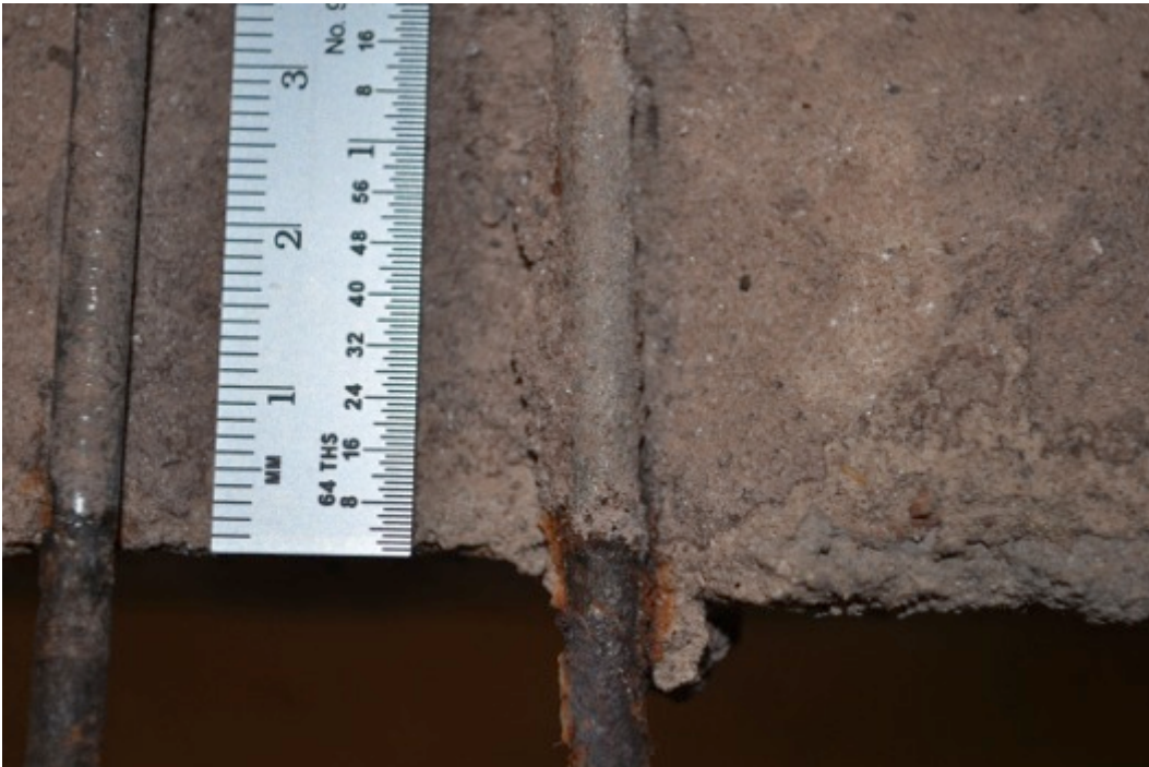
Figure 36. Destructive inspection of the interior of a standard steel (left) and galvanized (right) pintle after 18 months of exposure at Duck, NC.
