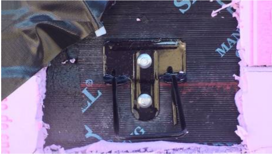
Figure 13. Installed pintles protruding through foam insulation.
