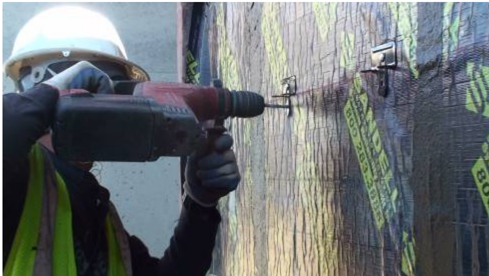
Figure 9. Drilling a pilot hole for a double-eye wall tie component.
