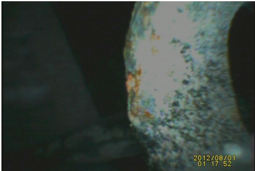
Figure 20. Borescope inspection of a vitreous coated wall tie after 18 months of exposure in Building 635 location 2-2.
