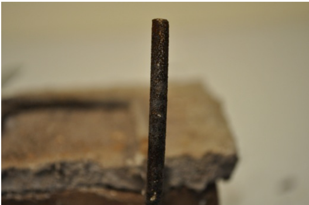
Figure 29. Inspection of the exterior part of the galvanized pintle after 18 months of exposure at Fort Stewart, GA.
