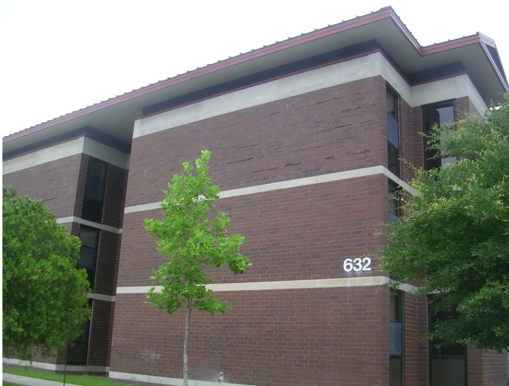
Figure 1. Exterior view of Building 632 brick veneer construction.
