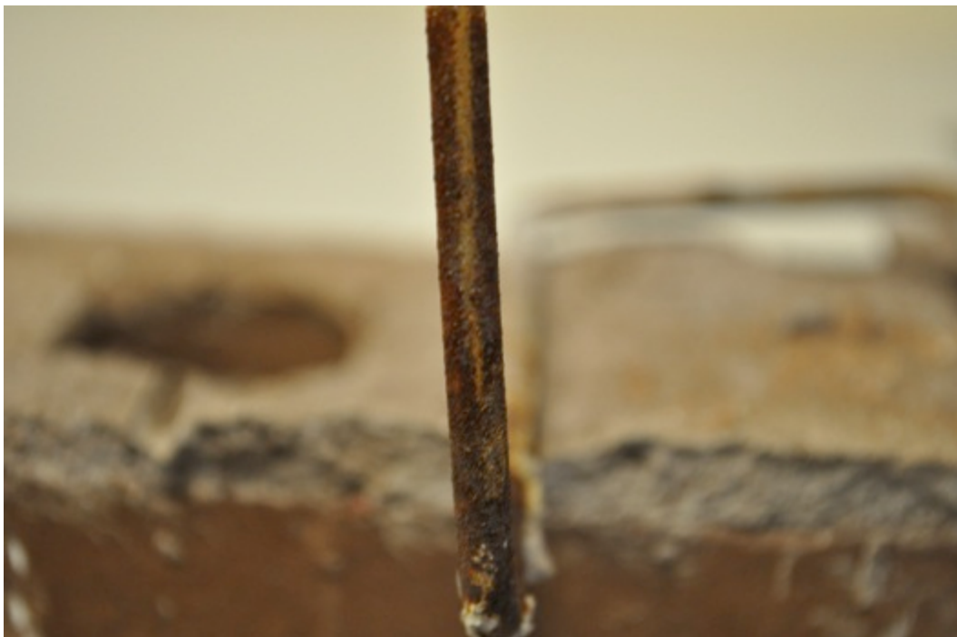
Figure 33. Inspection of the exterior part of the standard steel pintle after 18 months of exposure at Duck, NC.
