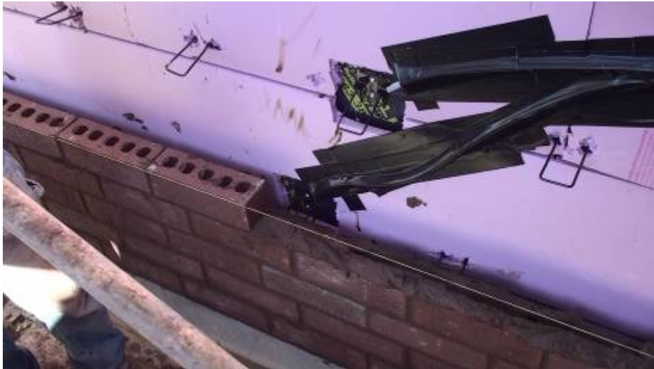
Figure 15. View showing brickwork and mortar adjacent to tubes and tie.
