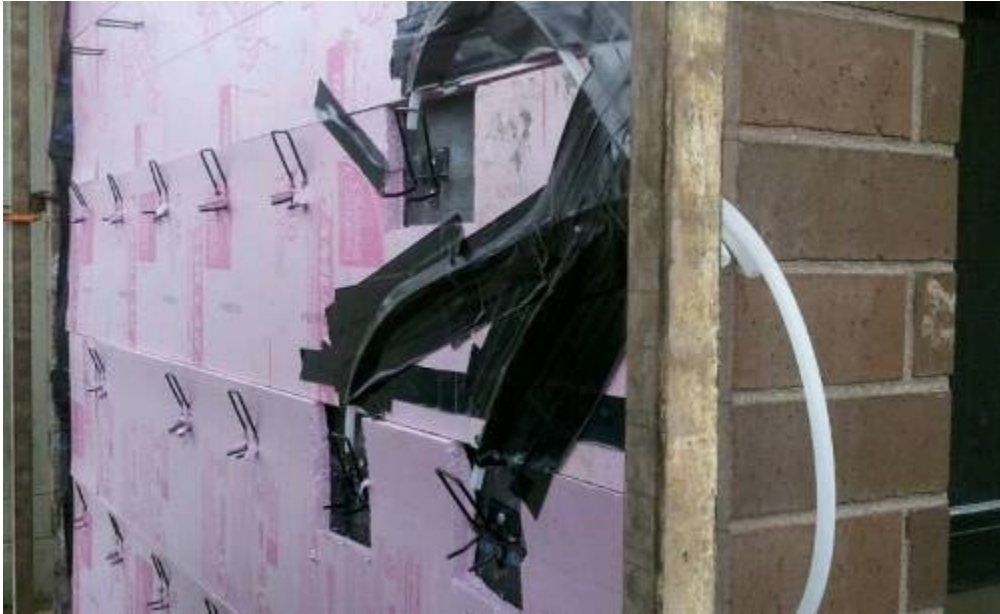
Figure 14. Plastic tubing for borescope inspection.
