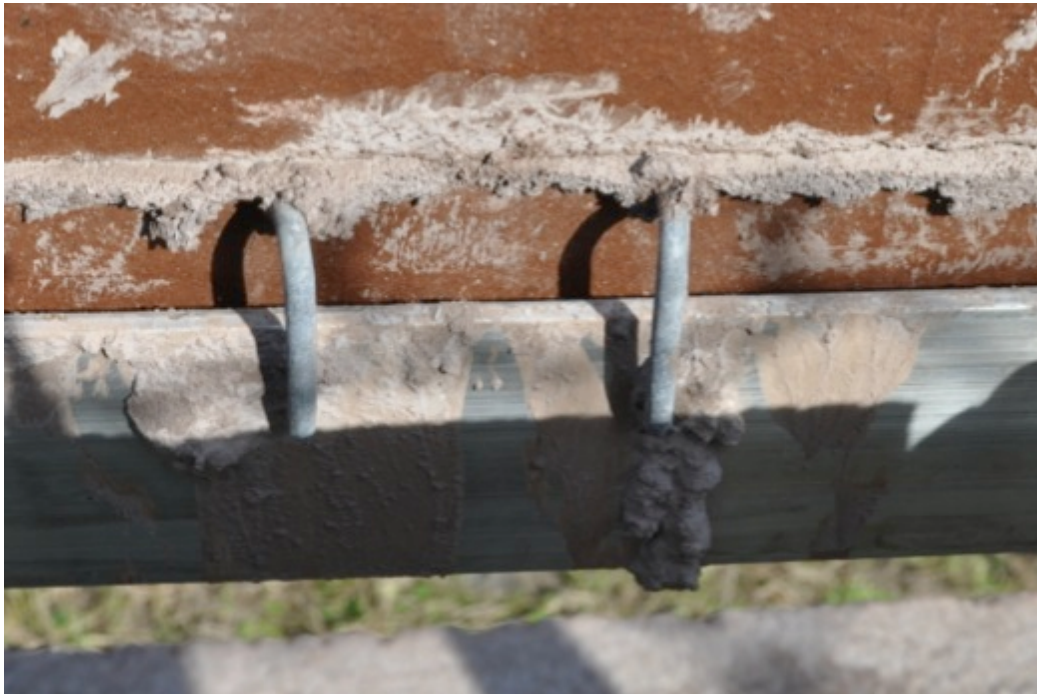
Figure 38. Solo galvanized pintle in an ASTM E754 brick coupon at Fort Stewart, GA.
