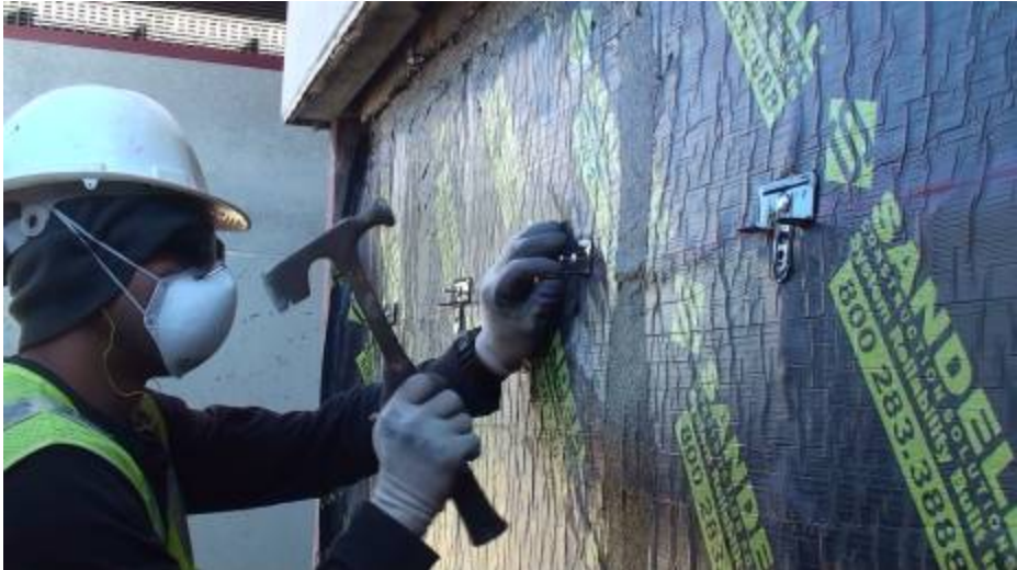
Figure 10. Installation of a double-eye wall tie component.
