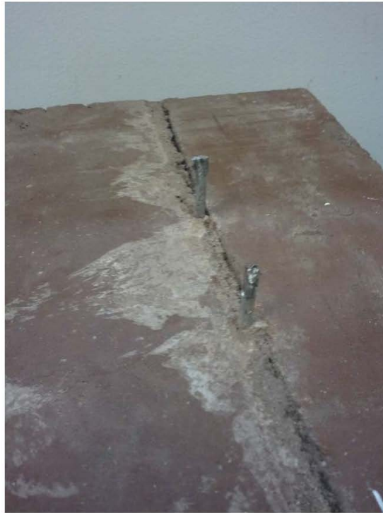
Photo 4 – Metal Tensile Failure
