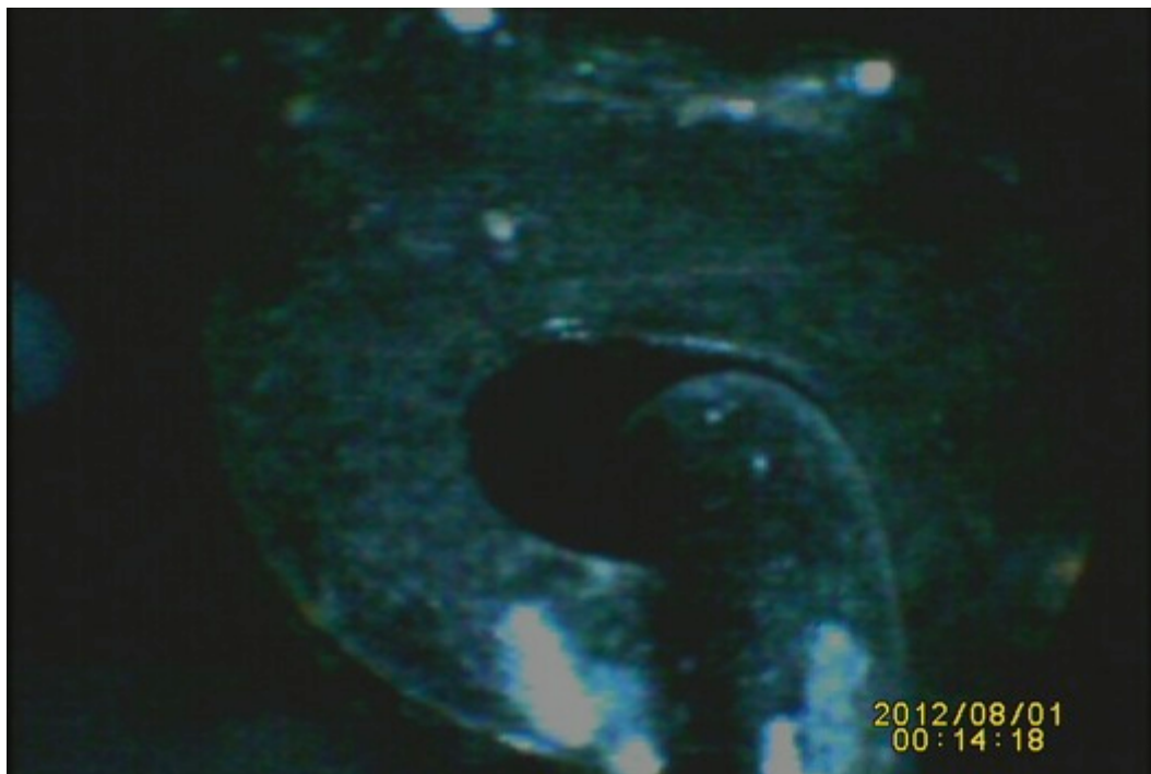
Figure 25. Borescope inspection of a vitreous coated wall tie after 18 months of exposure in Building 632 location 3-1.
