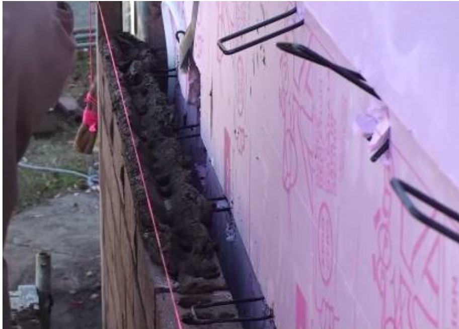
Figure 13. Installed pintles protruding through foam insulation.
