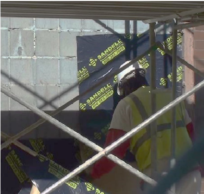
Figure 7. Application of the rubber sheathing.
