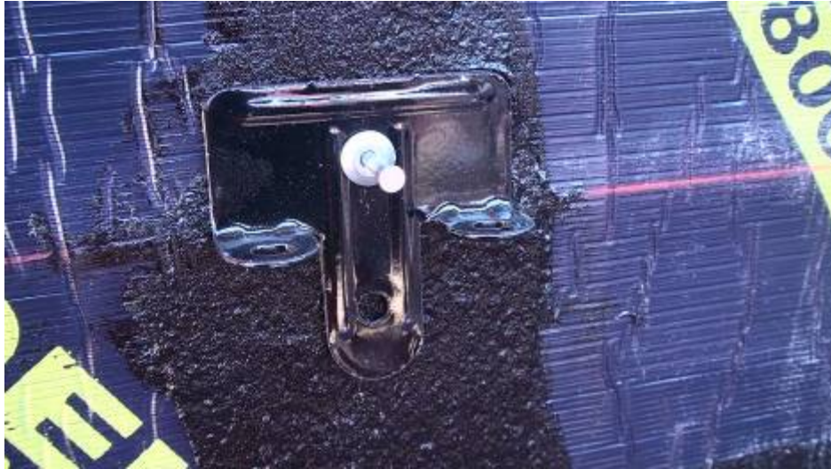
Figure 8. Installed double-eye component with chalk line for alignment.
