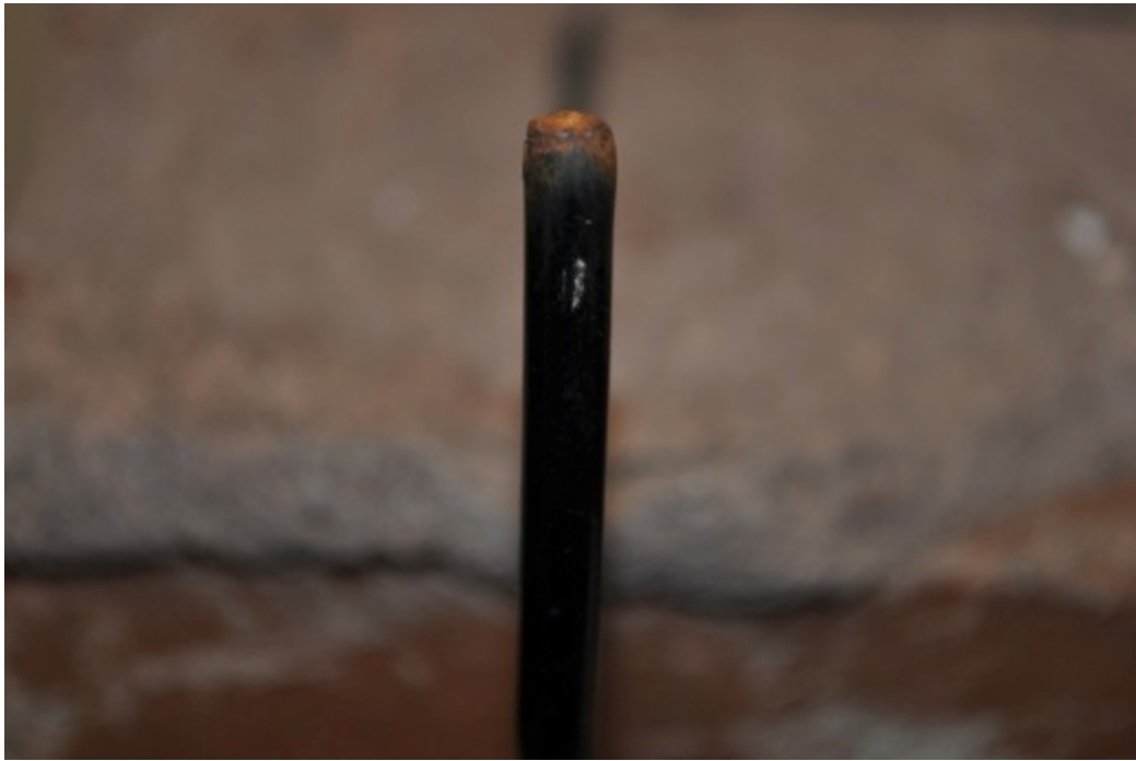
Figure 30. Inspection of the exterior tip of the galvanized pintle after 18 months of exposure at Fort Stewart, GA.
