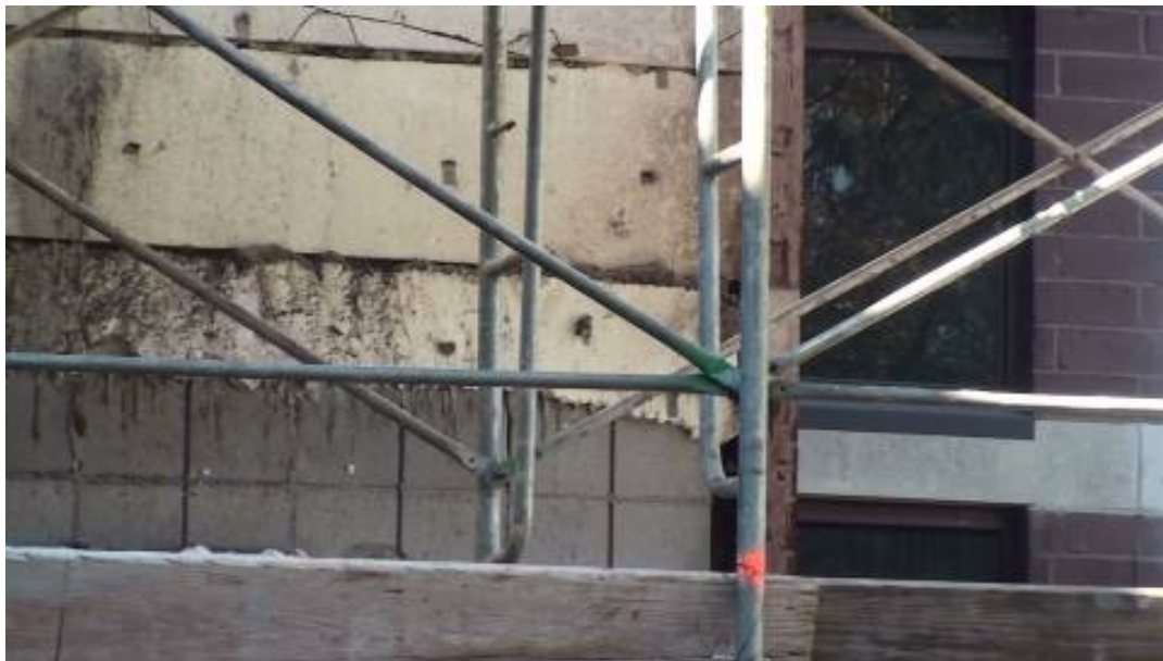
Figure 5. Selected panels stripped to bare walls.
