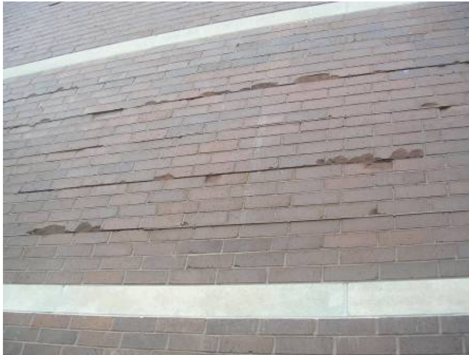
Figure 2. Failed masonry joints, showing spalled bricks.
