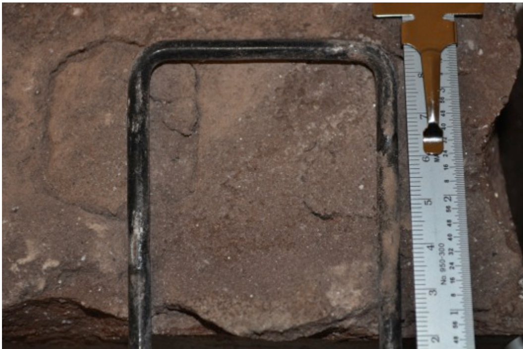
Figure 32. Destructive inspection of the interior of a vitreous coated pintle after 18 months of exposure at Fort Stewart, GA.
