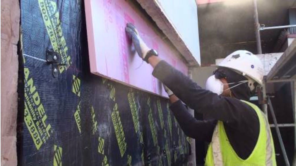
Figure 11. Installation of foam board insulation.
