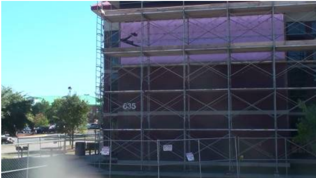
Figure 4. Scaffolding erected for project.
