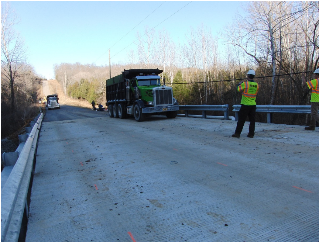
Figure 12. Finished bridge deck with the Gridform section in the foreground, and the conventional deck in the background (break is at the guardrail gap).
