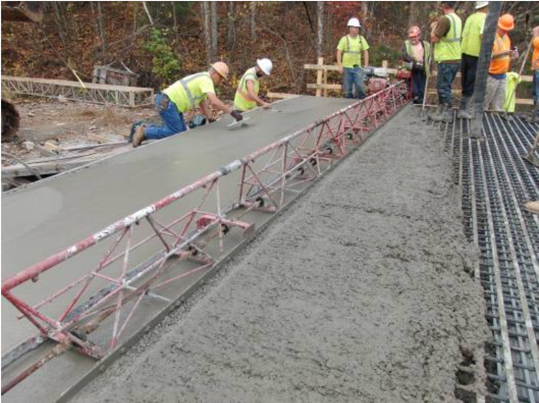
Figure 11. Spreading of concrete over the FRP reinforcement.
