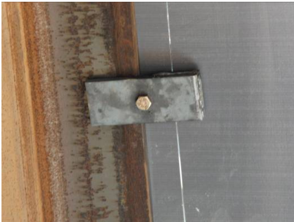
Figure 9. Fastening the FRP reinforcement panels to the top flange of the steel beam, using FRP blocks and stainless steel bolts (shown from below).
