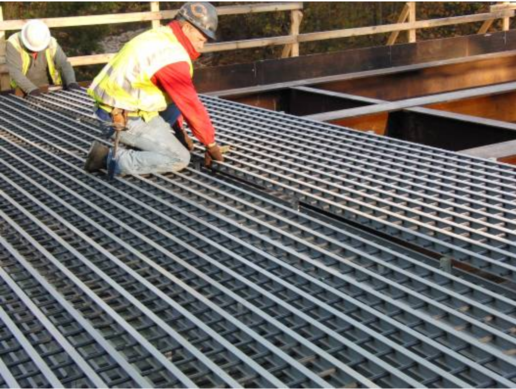
Figure 7. Manipulating the FRP reinforcement panels by hand.
