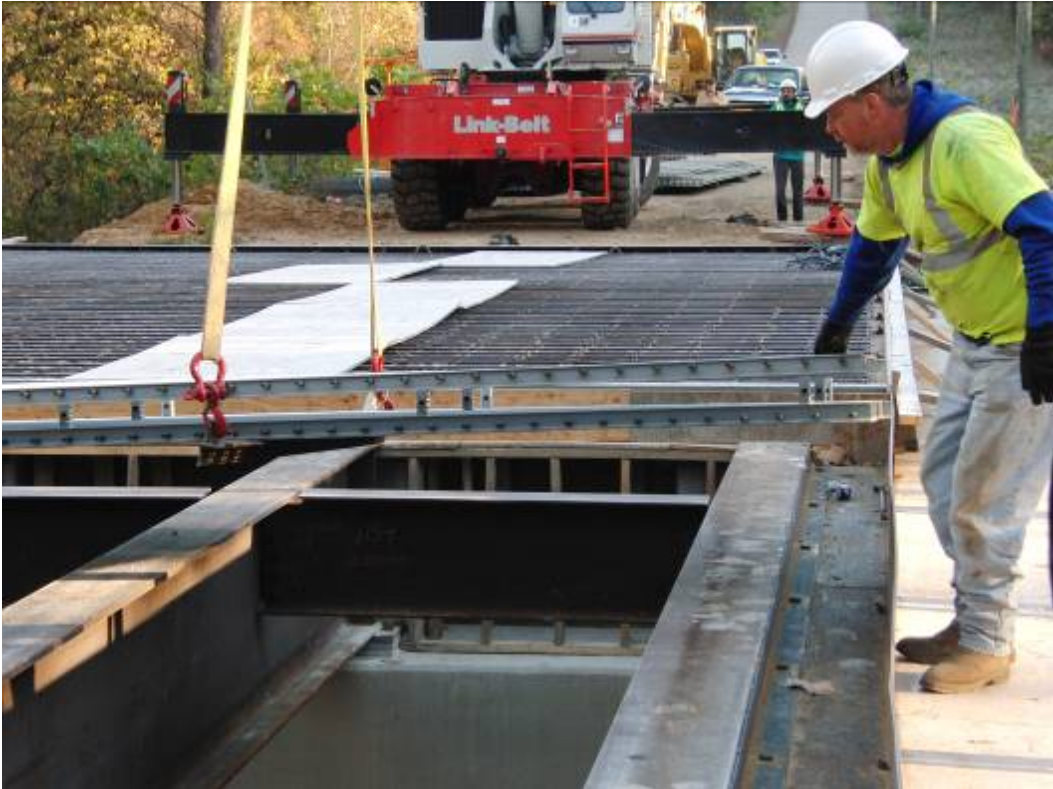
Figure 6. Guiding the FRP reinforcement panel installation.
