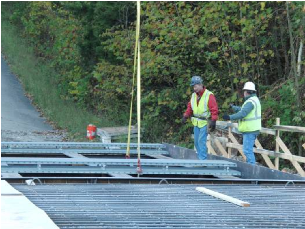
Figure 5. Placing FRP reinforcement panels by crane.
