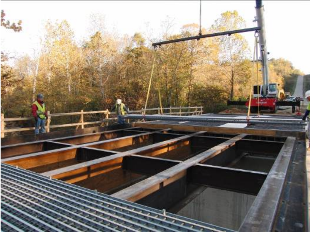
Figure 4. Crane lift of FRP reinforcement panels.
