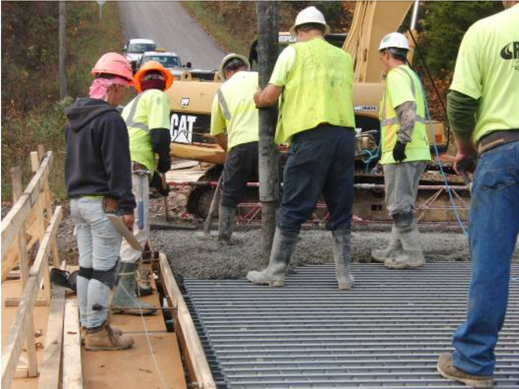
Figure 10. Concrete pouring and vibrating.
