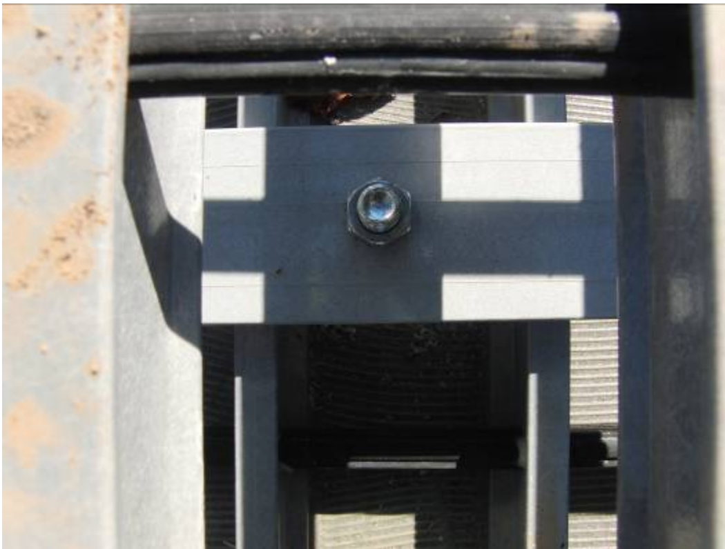
Figure 8. Fastening the bottom layer of FRP I-bars to the steel beam using FRP blocks and stainless steel bolts, shown from above.
