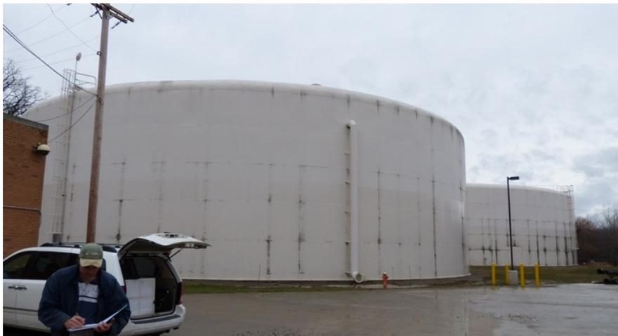
Figure B4. Polarization decay measurements in progress at the rectifier for the 5-million gallon water storage tank.
