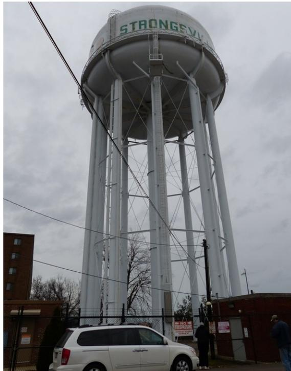
Figure B2. Polarization-decay measurements in progress at the CP rectifier for the 1-million gallon elevated water storage tank.
