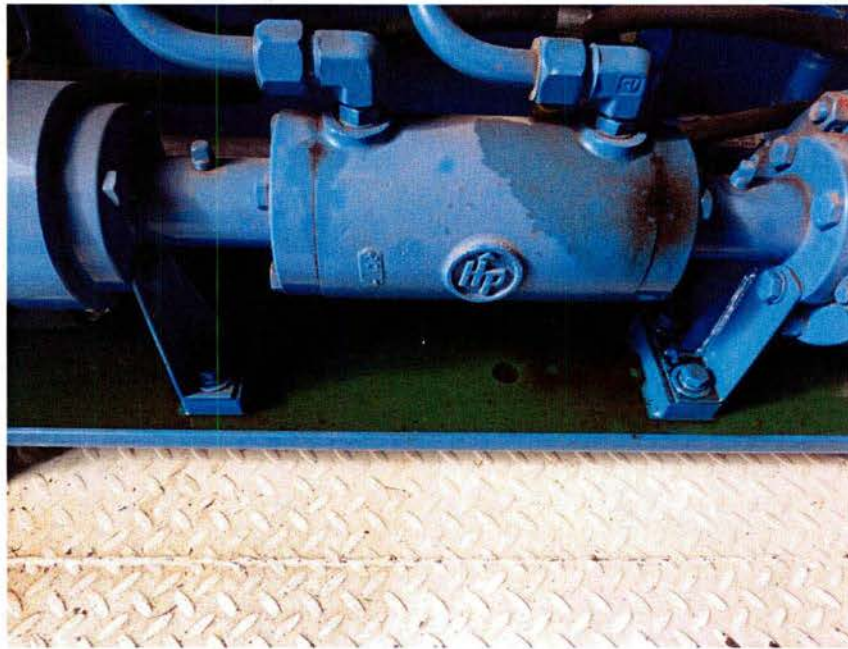
Figure 7.1.9: 350 bar Compressor Oil Leak
