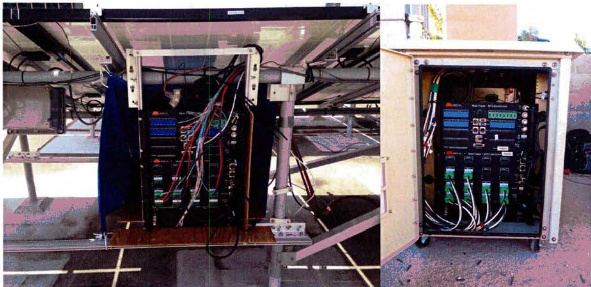
Figure 6.2: IV tracer installed on the rooftop of GHHI (left) and at the Maui test site in a weather-tight outdoor cabinet (right).
