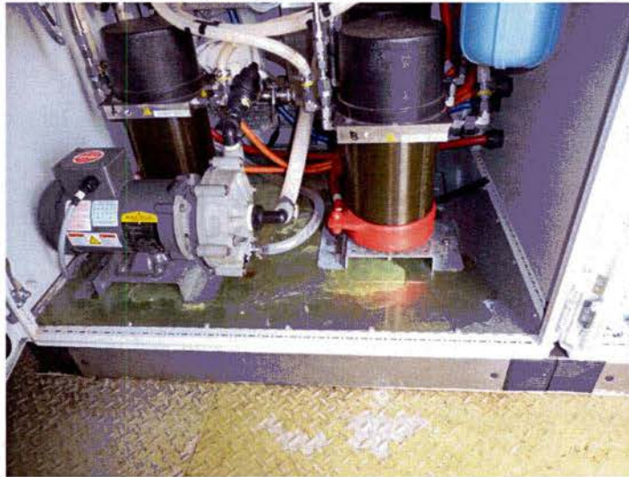
Figure 7.1.7: Heat Exchanger Coolant Leak Heat
