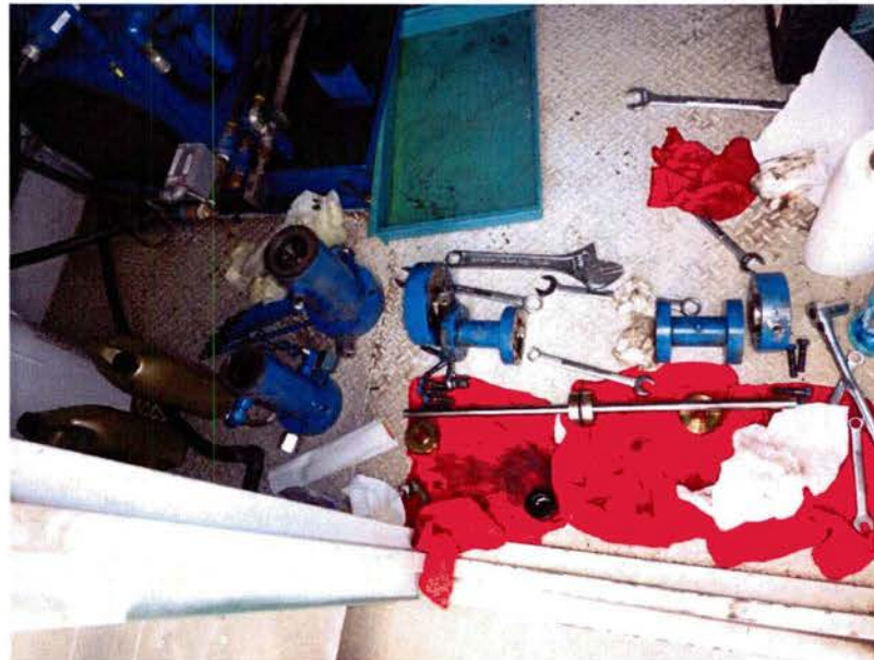
Figure 7.1.10: Repair of 350 bar Compressor in Progress
