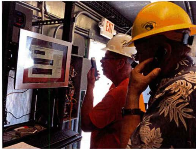
Figure 5.2.1: Hawaiian Electric Company (HECO)/Campbell Industrial Park (CIP) Site Acceptance Test.
