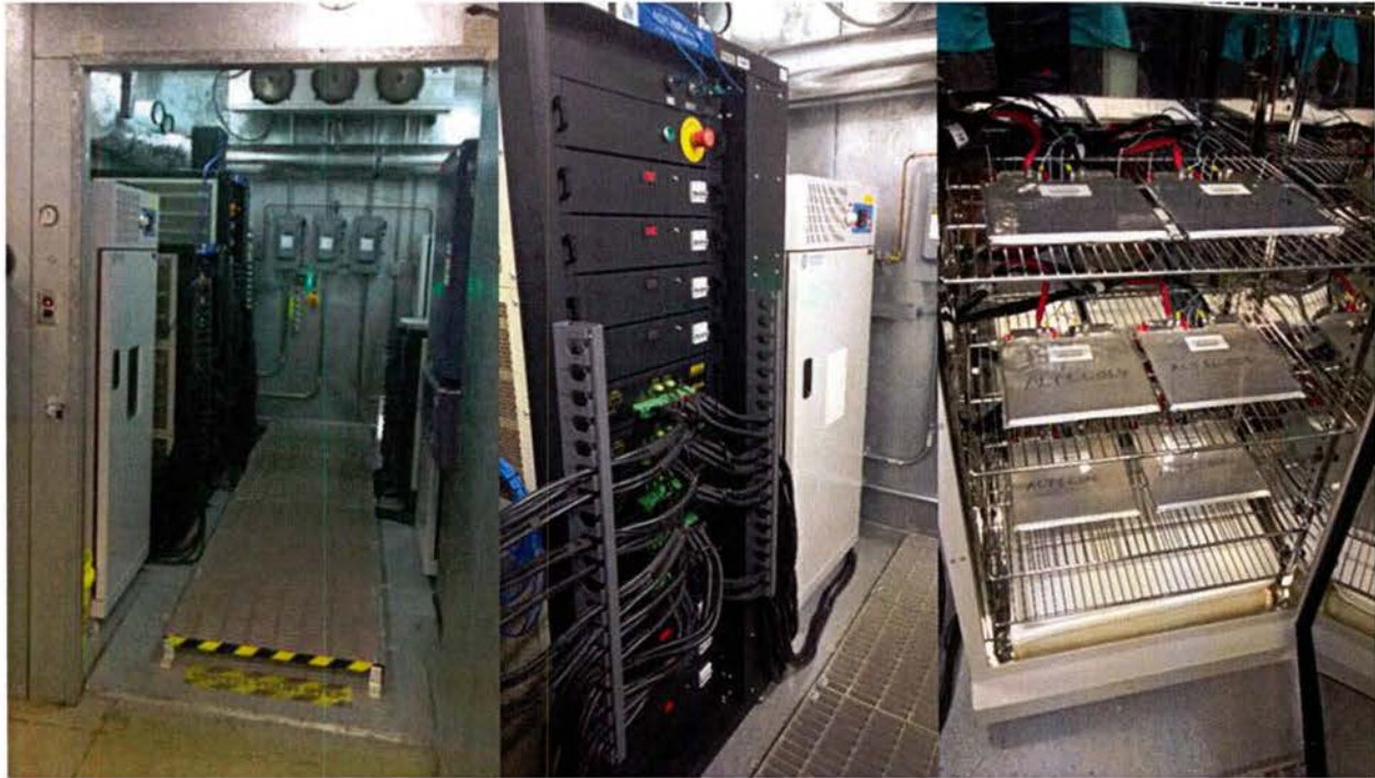
Figure 5.1.2: (Left) Entrance to the battery laboratory, a self-contained converted refrigerator unit. (Center) 20-channel Arbin battery tester and climate chamber by its side. (Right) large format Altairnano cells in the climate chamber.
