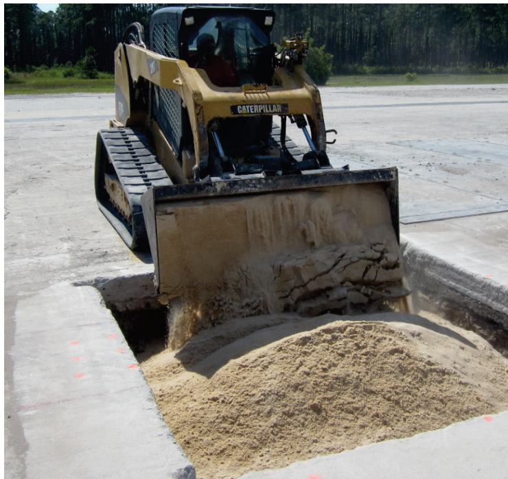
Figure 8. Masonry sand backfill.
