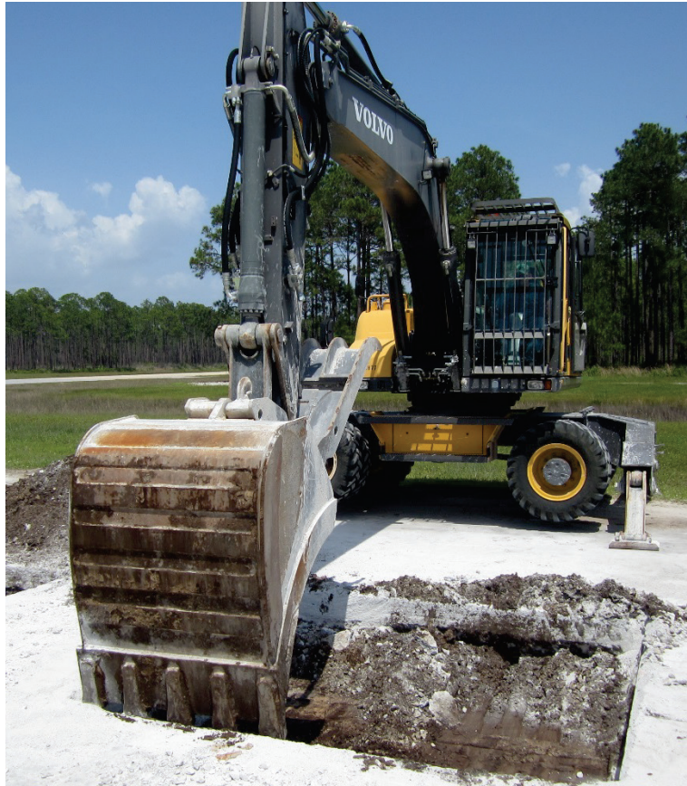
Figure 11. Excavation using the Volvo EW 180C wheeled excavator.
