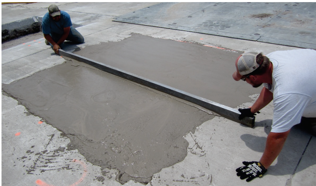
Figure 17. Screeding of rapid-setting flowable fill cap.
