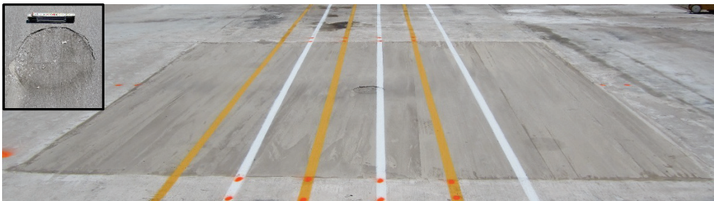
Figure 27. Crater 8 before trafficking.
