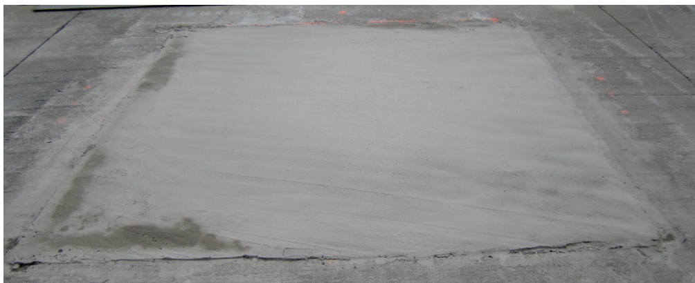
Figure 23. Crater 2 before trafficking.
