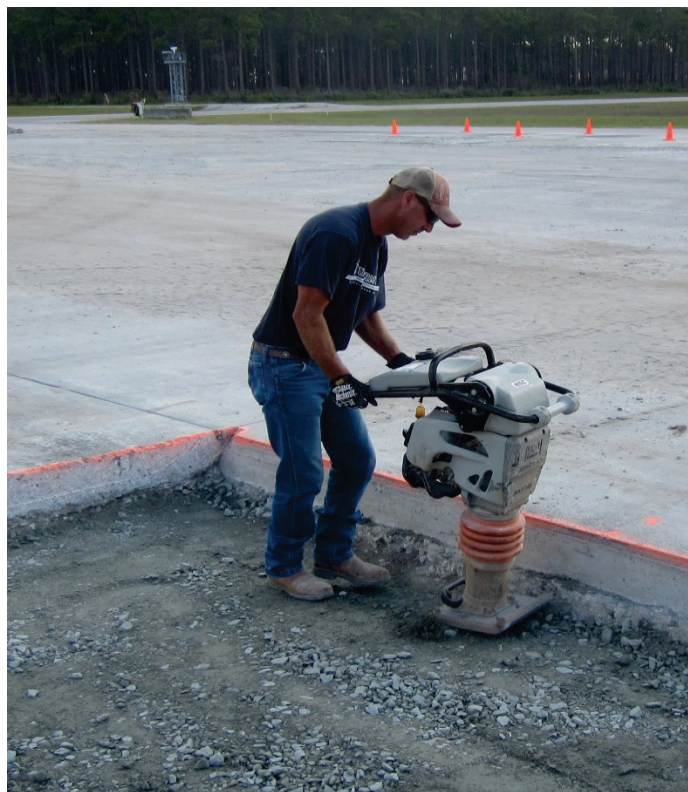
Figure 4. Multiquip Mikasa MTX-70 rammer-style compactor.
