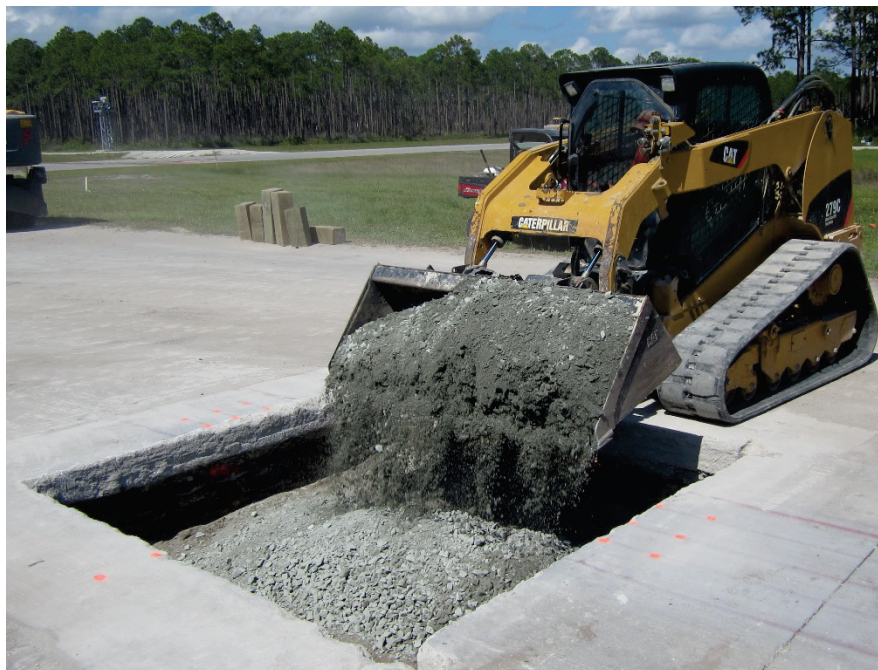
Figure 7. Crushed stone limestone backfill.
