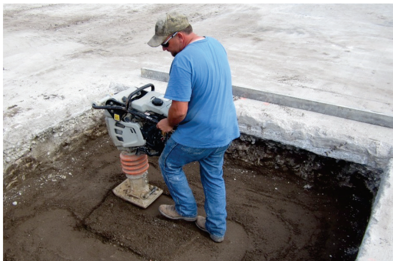
Figure 14. Compaction of natural subgrade.
