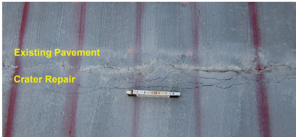
Figure 34. Crater 1, 512 passes, medium-severity joint spalling.
