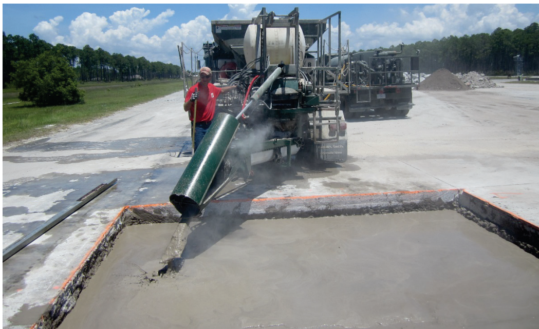
Figure 16. Rapid-setting flowable fill placement during a large crater repair.
