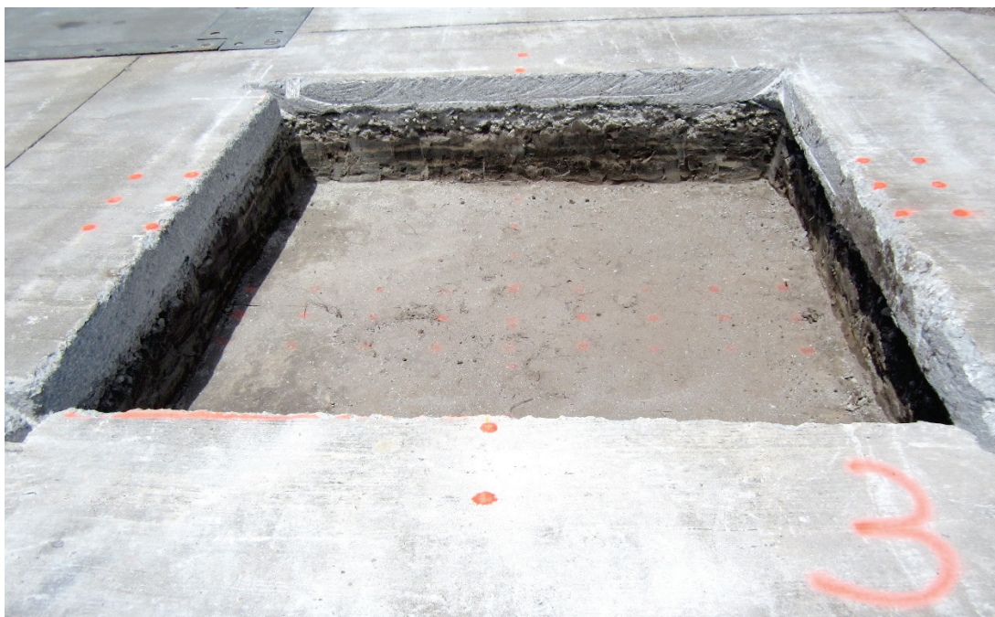
Figure 12. Excavated 8.5-ft by 8.5-ft crater
