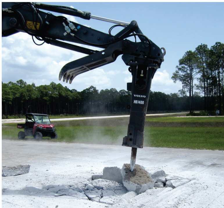
Figure 10. Breaking using Volvo HB 1400 breaker attachment.
