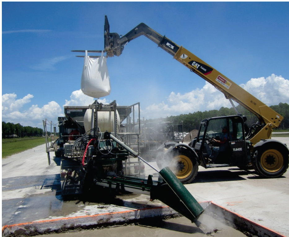
Figure 5. Extendable-boom forklift loading supersack into volumetric mixer.
