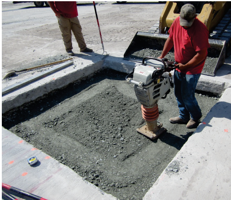
Figure 15. Compaction of crushed stone backfill material.
