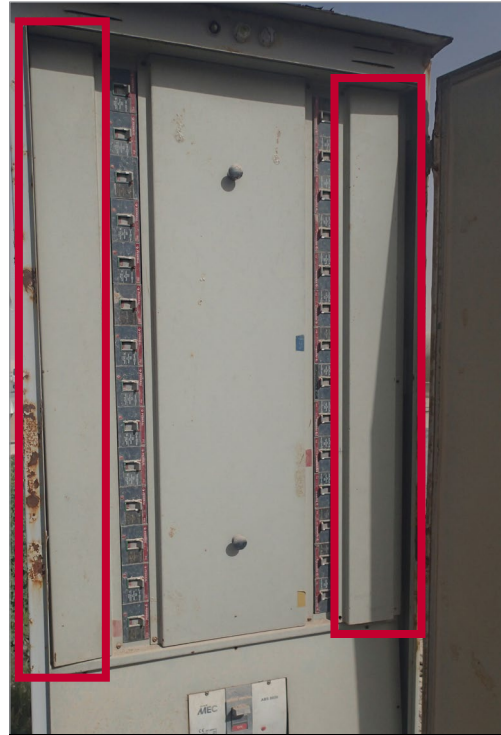
Figure 6. Unlabeled electrical distribution panel (Deficiency No. BUH-EL-160226-054) Source: DoD OIG
