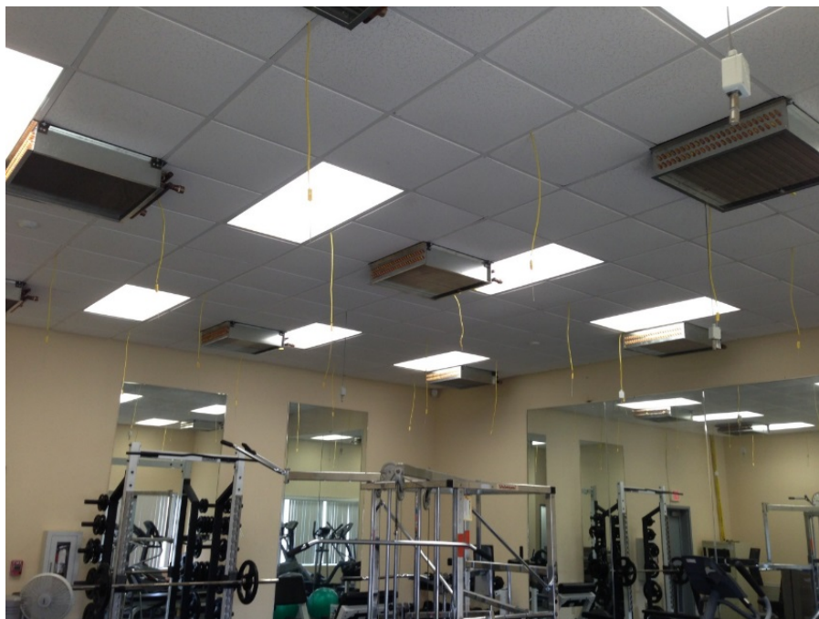
Figure 20: Exercise room complete ceiling coil installation
