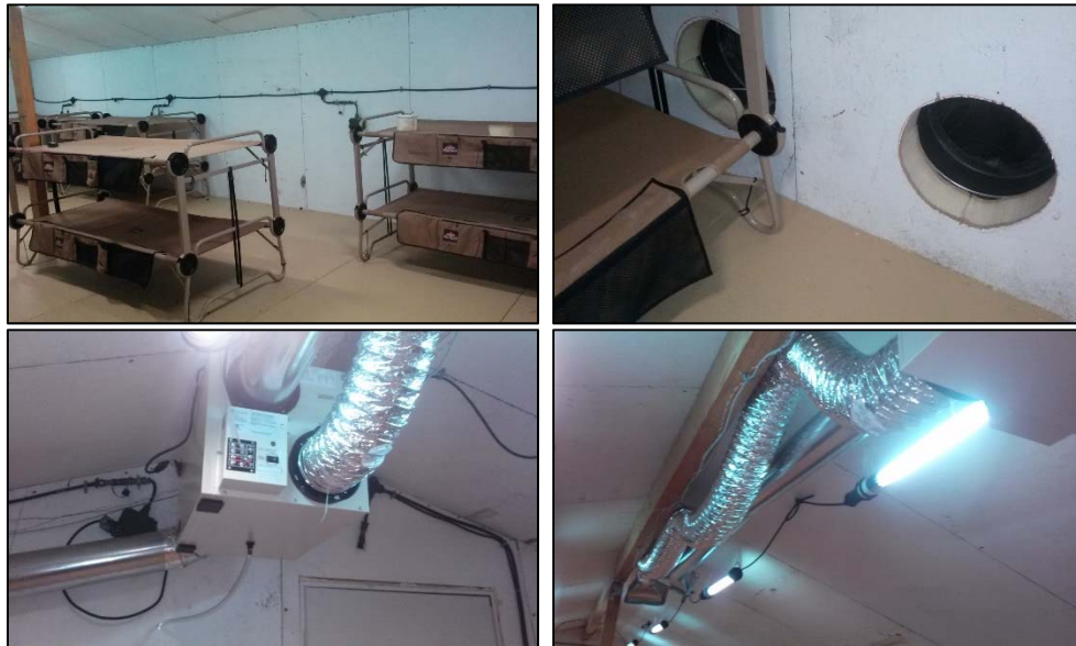
Figure B-2: Interior of SIP-Hut 2, Bunks Installed in Hut, ECU Ducts, Air Exchanger and Air Exchanger Ducts
