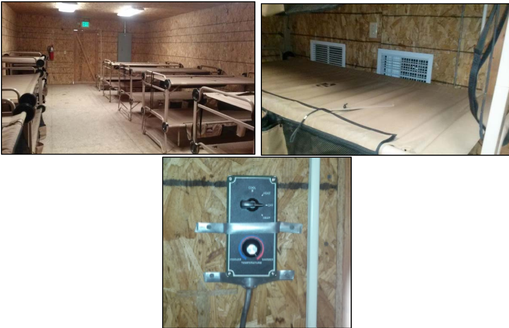
Figure B-6: Interior of B-Hut 1H, Bunks Installed, Ducts Installed and ECU
