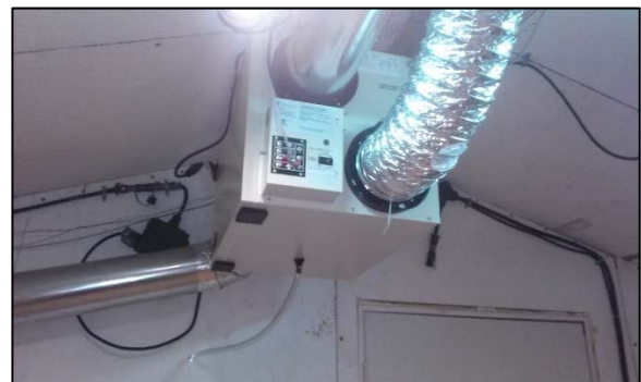
Figure 92: Air Exchanger in SIP-Hut
