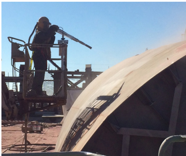
NMC and Ingalls developed and implemented an easy-to-use prototype mechanical arm to perform hull exterior abrasive blasting from a man lift during ship construction. Ingalls photo
