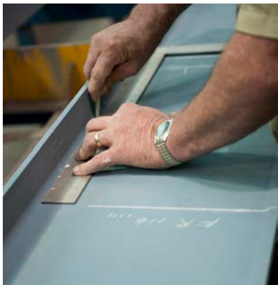
Automating the cutting and welding of stiffeners will reduce shipbuilding costs and improve the schedule due to reduced labor and improved efficiency and quality. Ingalls photo
