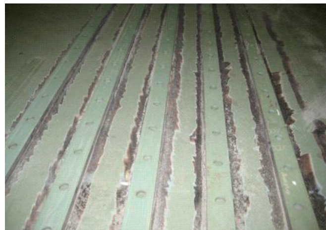
Improving the manufacturability and installation of weapons magazine C-channels will reduce labor and costs. Ingalls photo
