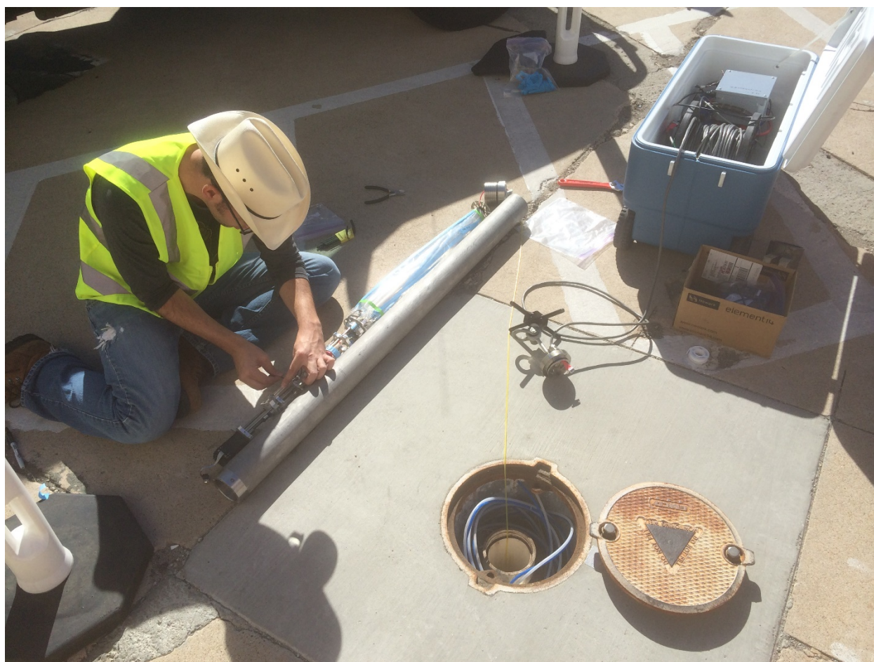
Figure 5-23. Field assembly and installation of the IS2 at NASNI.
