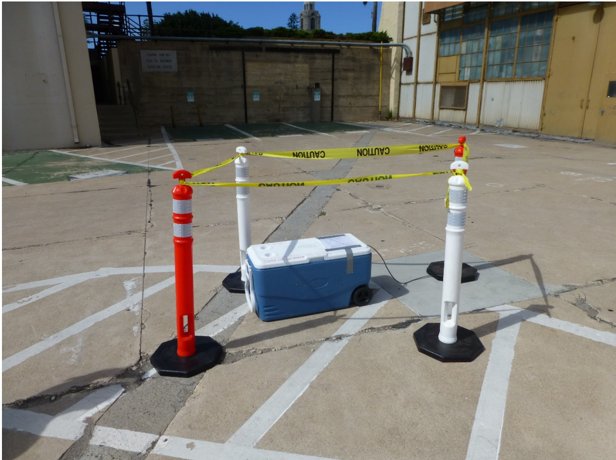
Figure 5-6. IS2 surface package at an installation. Batteries and communication are stored in the waterproof container, and an electrical control cable extends into the well. The surface package location is determined by site safety considerations; here it is located at a restricted-access site, in a low-traffic location.
