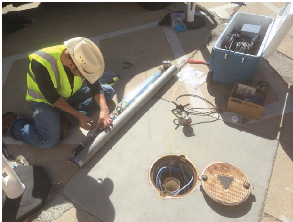
Figure 29. Field assembly and installation of the IS2 at NASNI.
