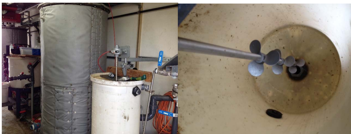
Figure 20. Phase IV feed tank and mixer assembly adjacent to the digester.
