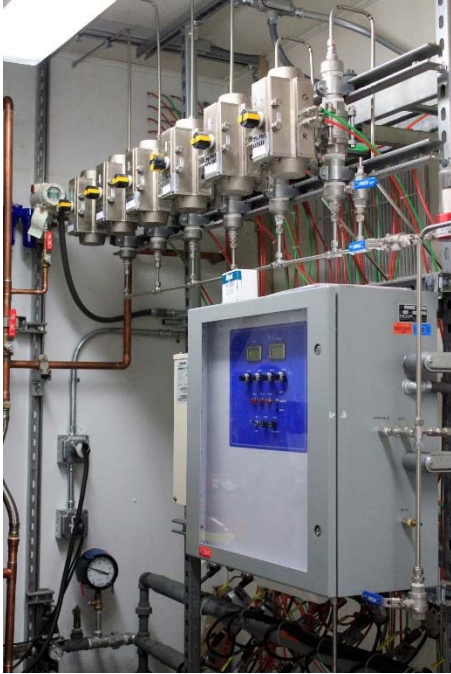
Figure 24. Nova gas analyzer with stream switching valves.
