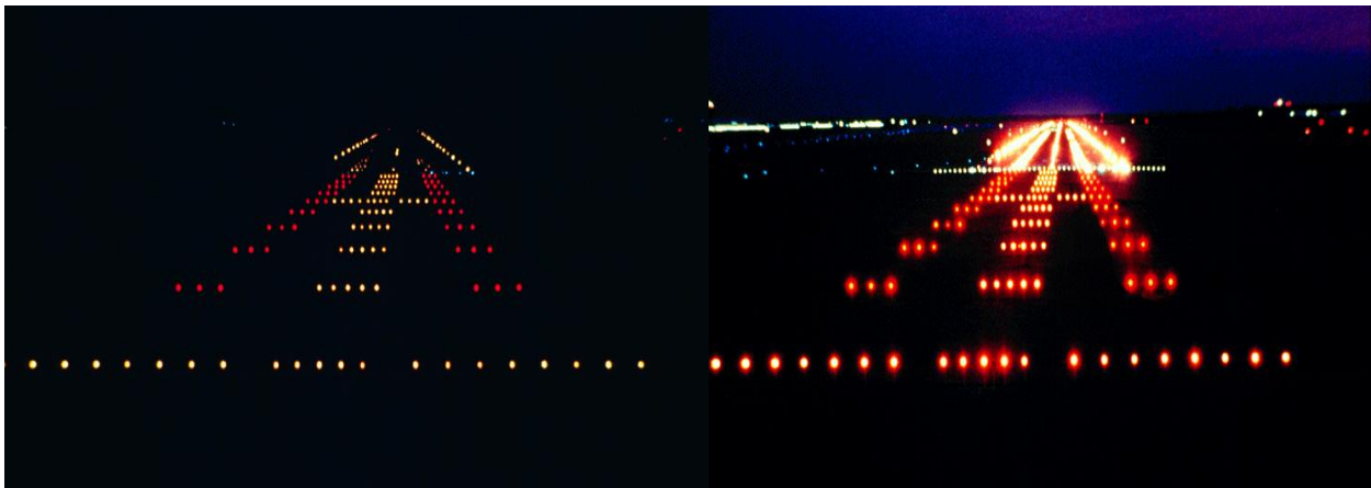
Figure 7.3.6.1-1. Comparison between a Dimly Lit Runway and a Bright Runway with the Same Lighting Configuration
