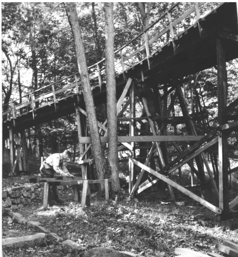
Figure 16. Repair of narrow-gauge railway trestle near Building 559, circa 1940s (PICA History Office).
