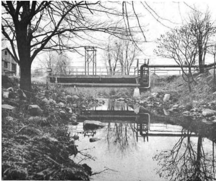
Figure 34. Steam piping and air piping across creek at Whittmore Ave, circa 1958 (PICA Cultural Resources).
