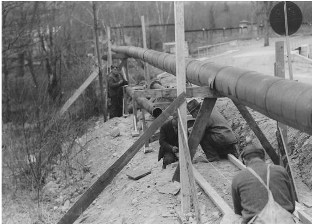
Figure 35. Relocating outside steam lines, date unknown (PICA Cultural Resources).
