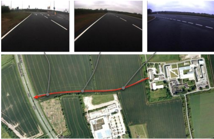
Figure 4.36: Featureless road section. A relatively featureless section near the Begbroke Science Park. The lack of informative structure in this region requires us to utilise the reflective properties of the LIDAR data.
