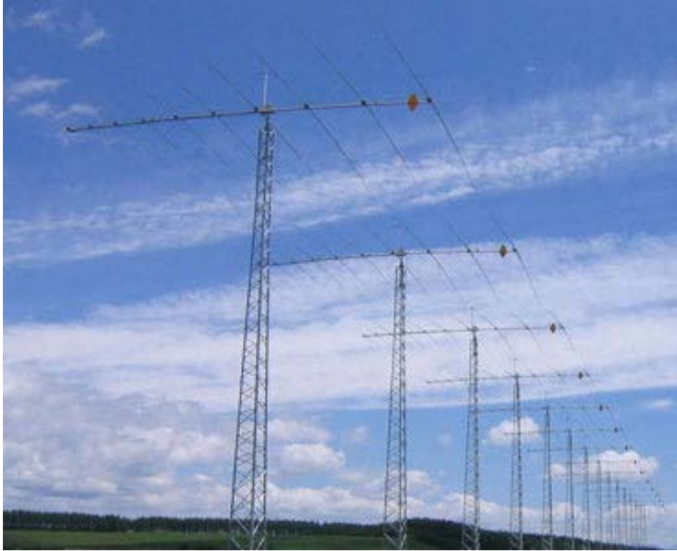
Figure 7: SuperDARN Antenna (Nagano Website)
