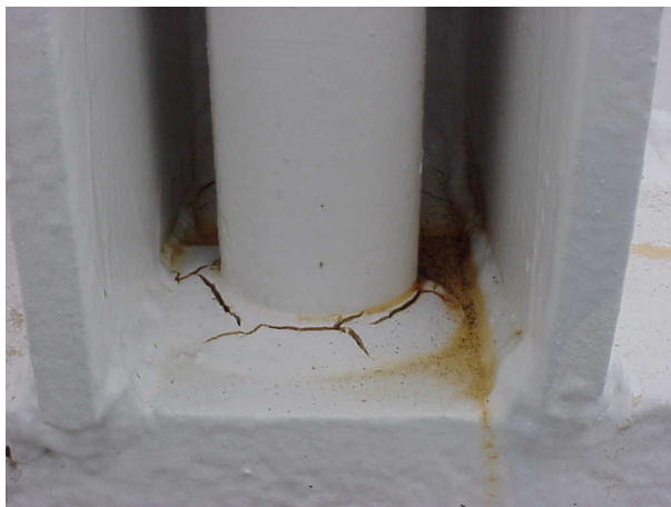
Figure 1. Example of failure due to excessive thickness.
