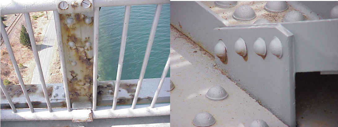
Figure 3. Examples of failure near bolts, rivets, and welds.
