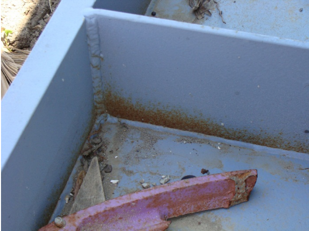
Figure 2. Example of failure from too thin of a coating.
