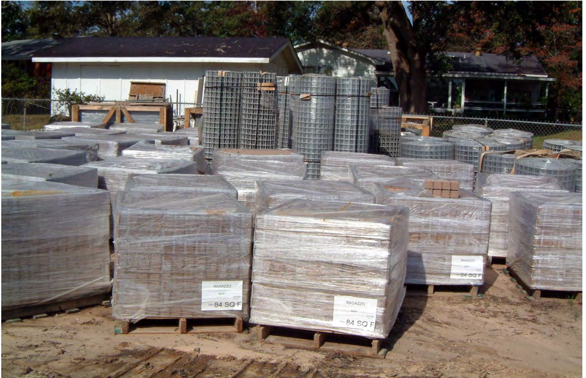
CONCRETE “RAGAZZO” BLOCKS AND GABION “ROLL-STOCK” MATERIAL AT JOBSITE
