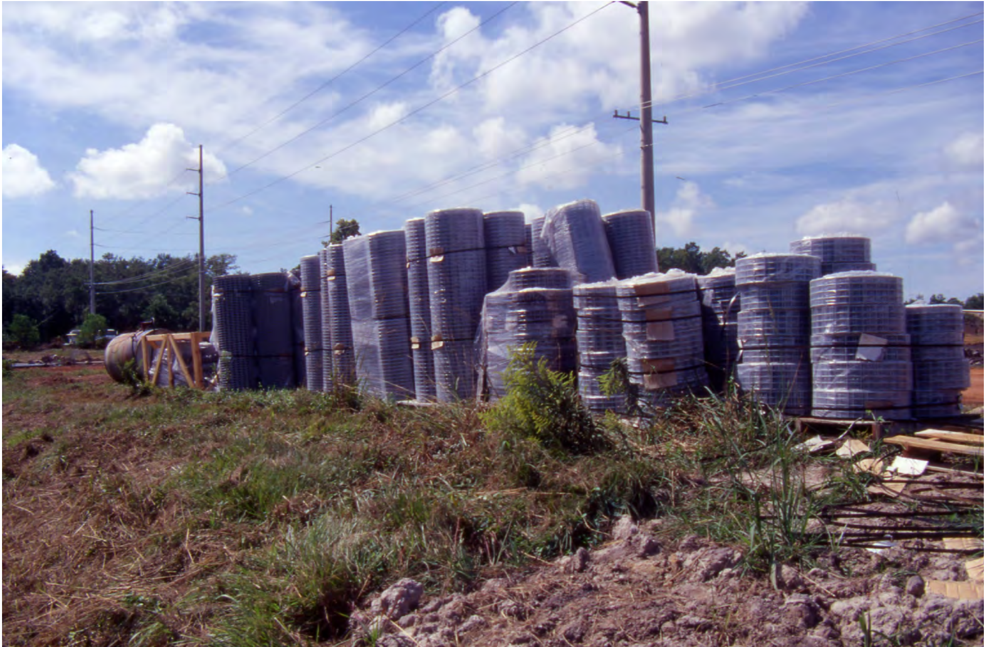
“ROLL-STOCK” GABION MATERIAL DELIVERED TO JOBSITE
