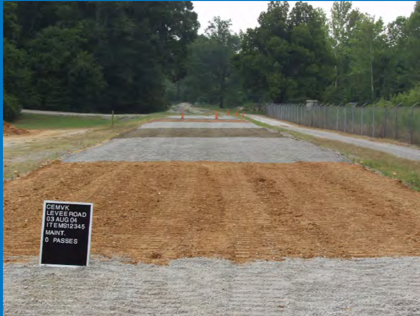
Maintenance Test Section
