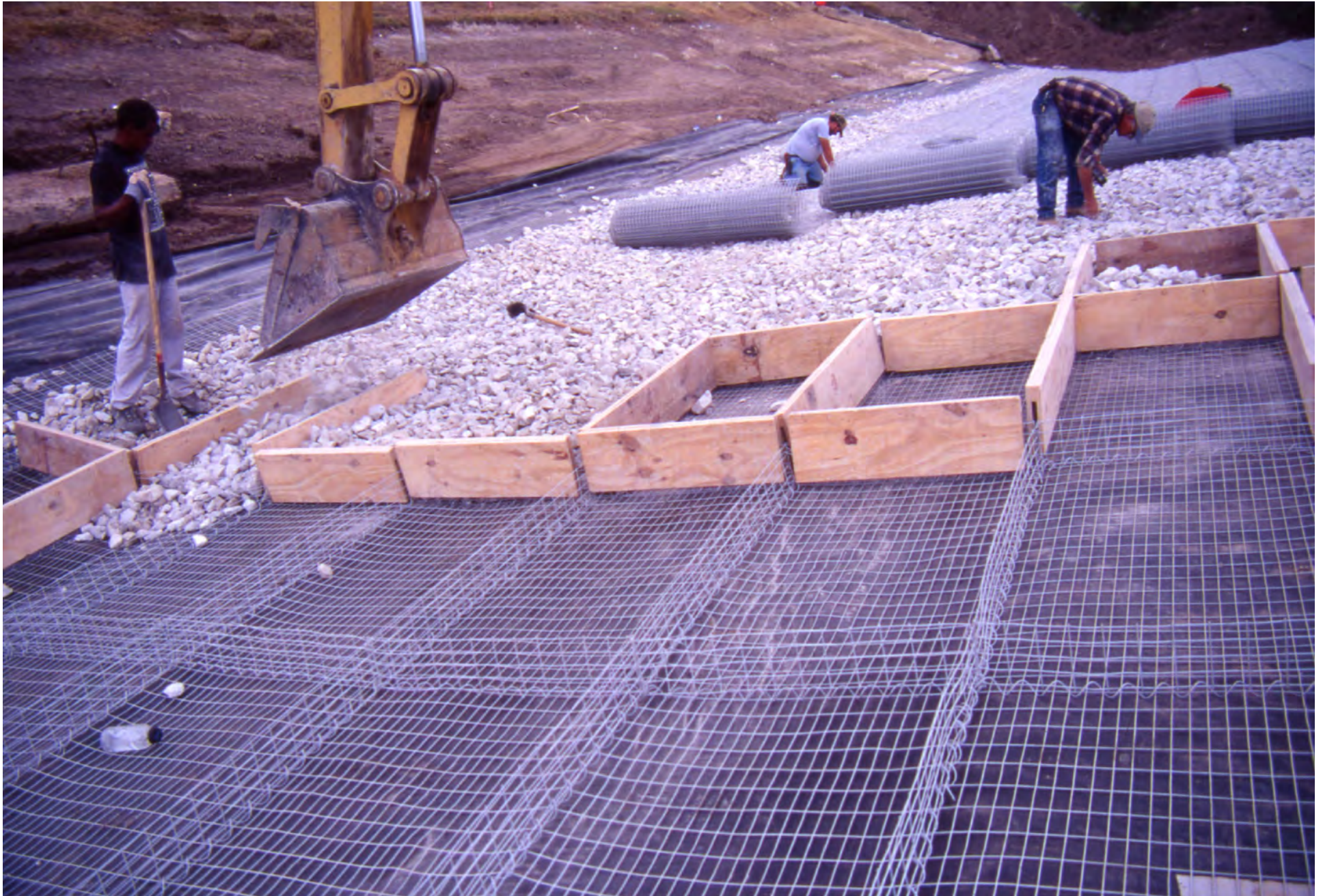
ROCK-FILLING THE GABION MATTRESS
