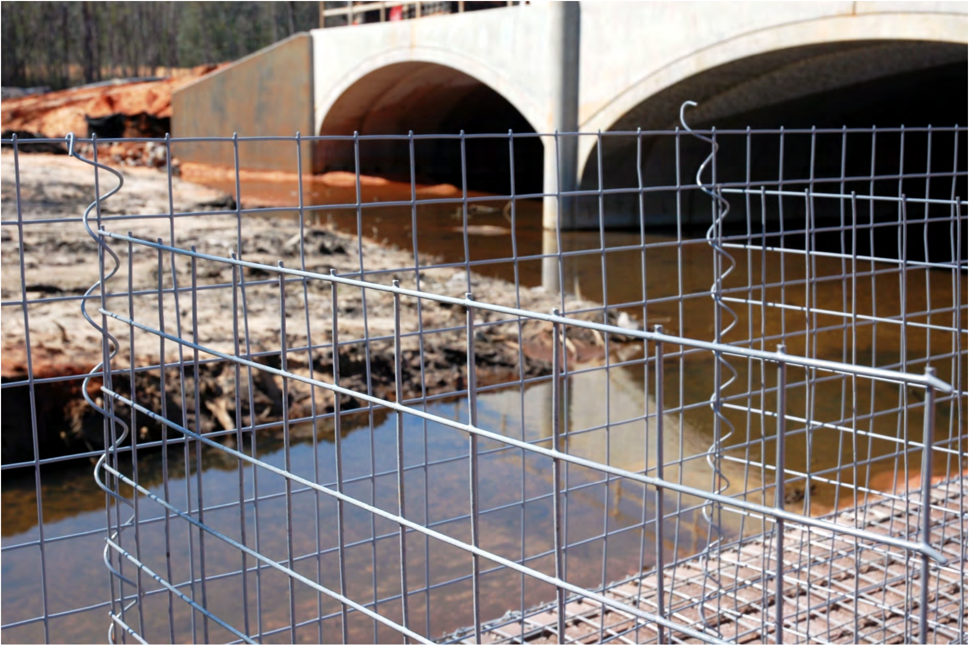
SPIRAL BINDERS – VERTICAL JOINTS
