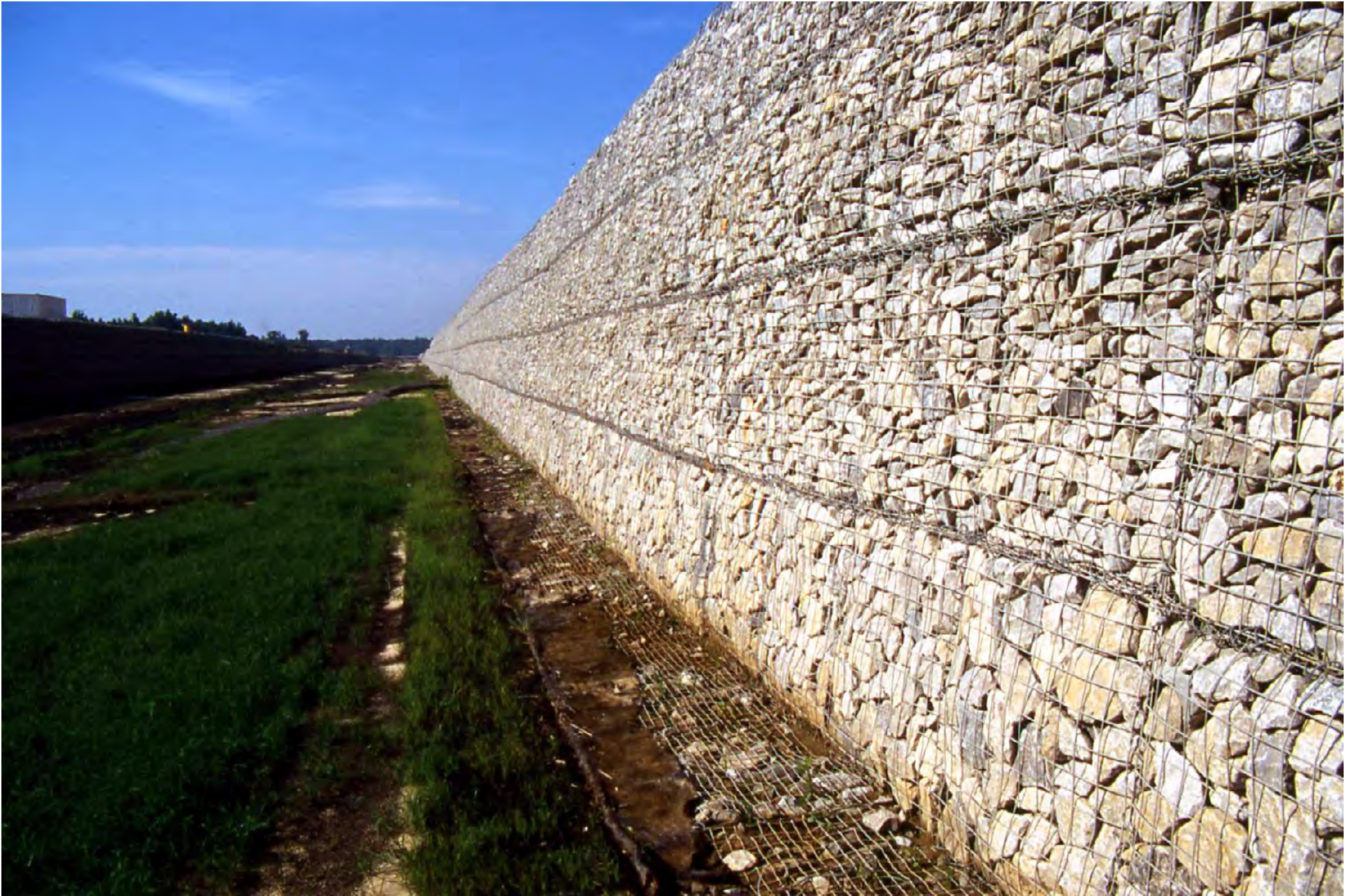
TYPICAL GABION WALL
