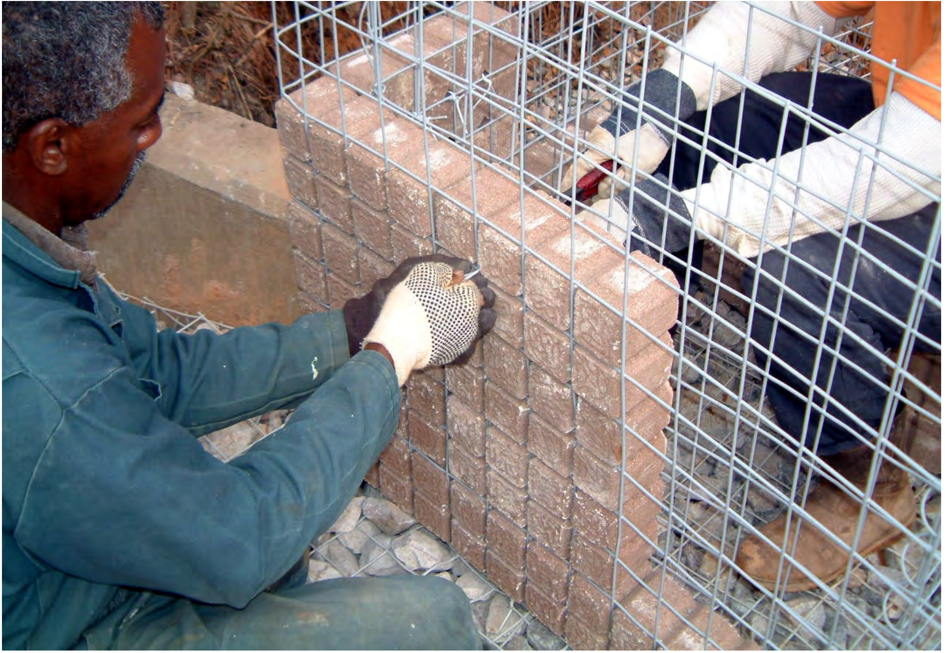
TWO MAN CREW SECURES BLOCKS IN PLACE
