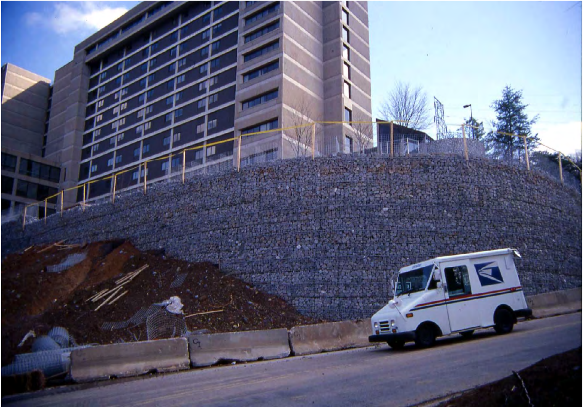
MSE GABION WALL ABOUT 1/2 COMPLETED
