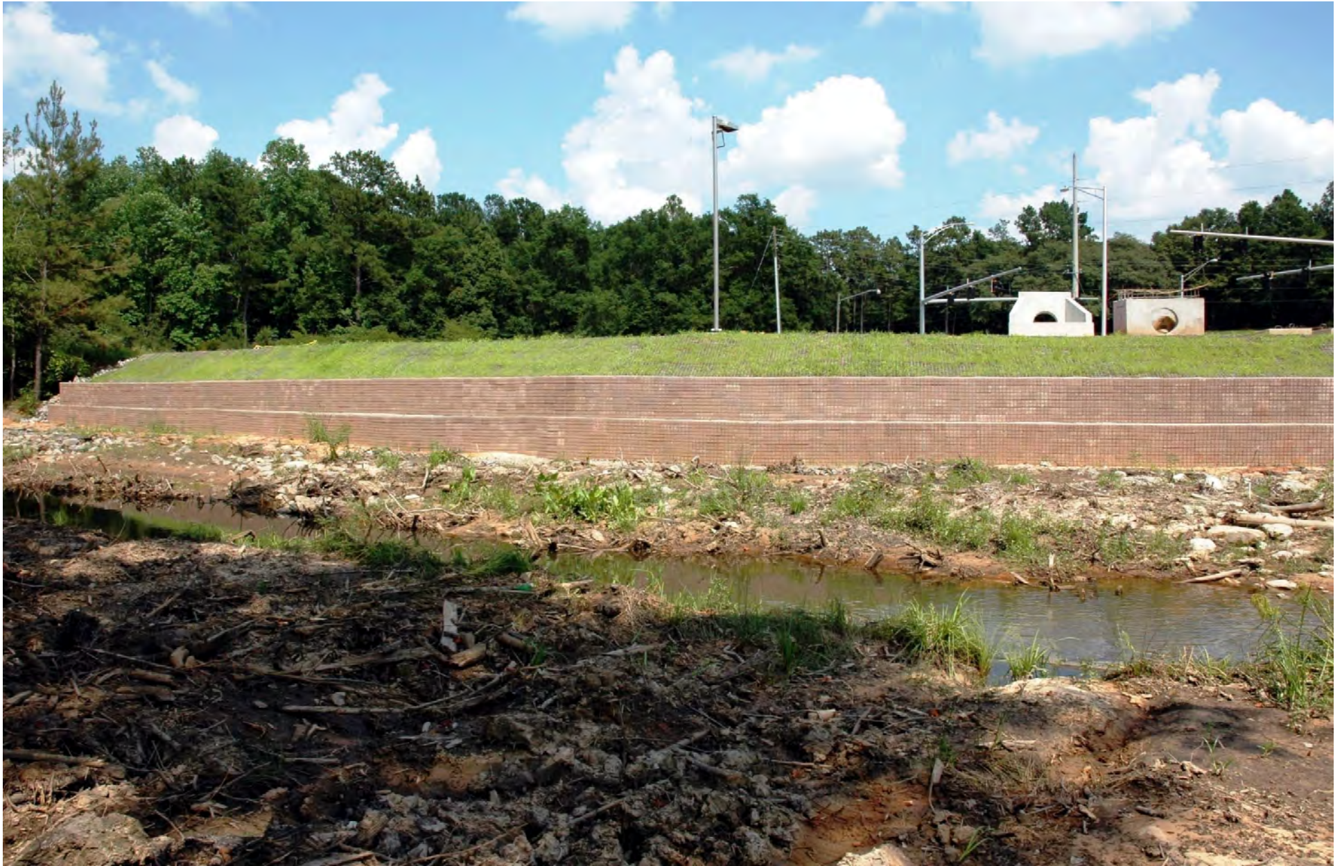
SECTION OF CONCRETE “RAGAZZO” BLOCKS FACED GABION WALL COMPLETED
