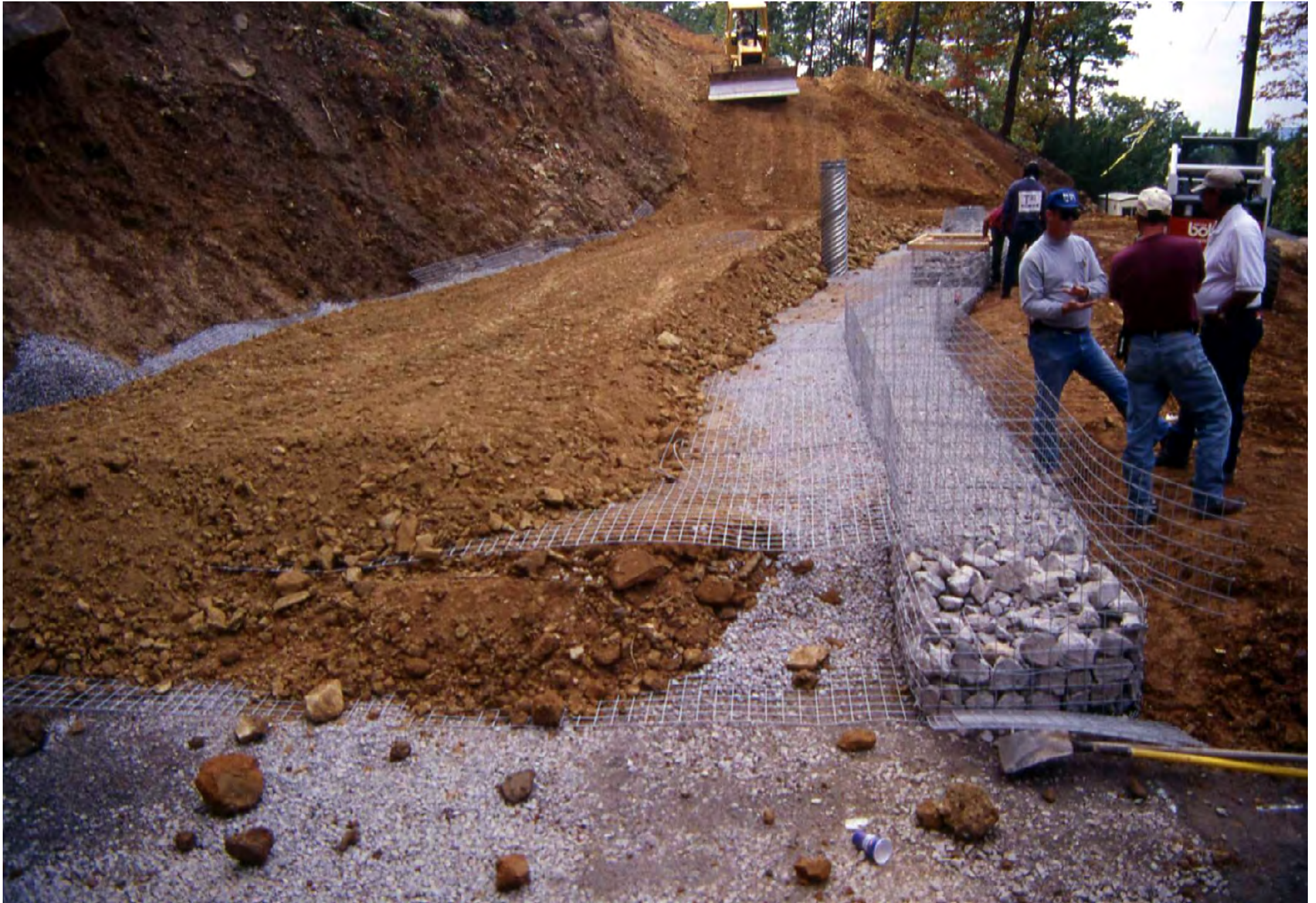
TYPICAL MSE GABION WALL CONSTRUCTION
