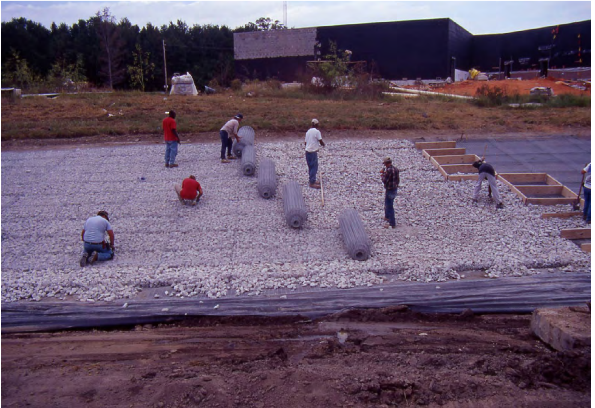
LEVELING ROCK-FILL & LID CLOSING
