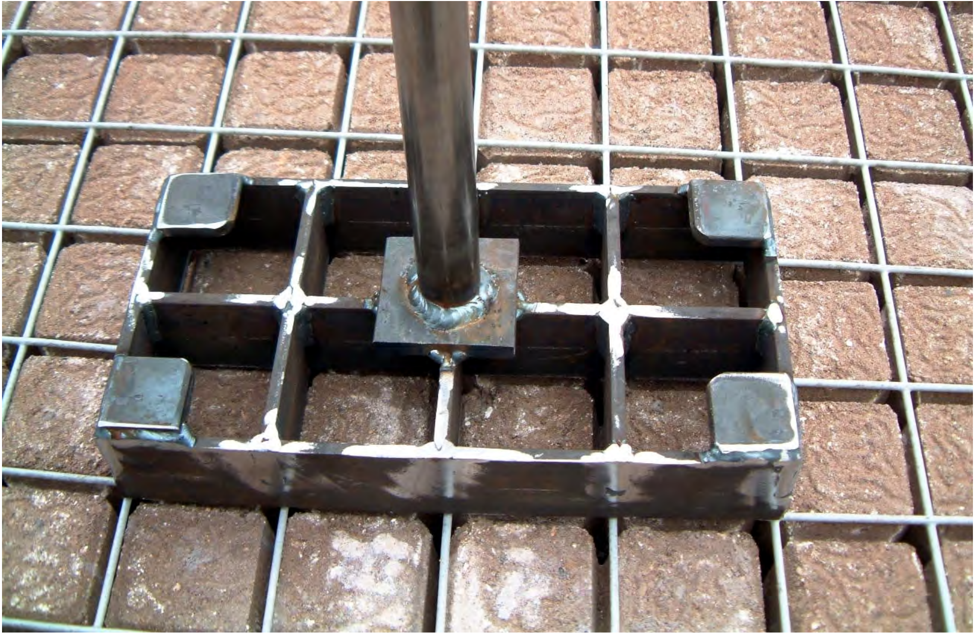
TOOL DESIGNED TO RECESS GABION MESH INTO BLOCK GROOVES
