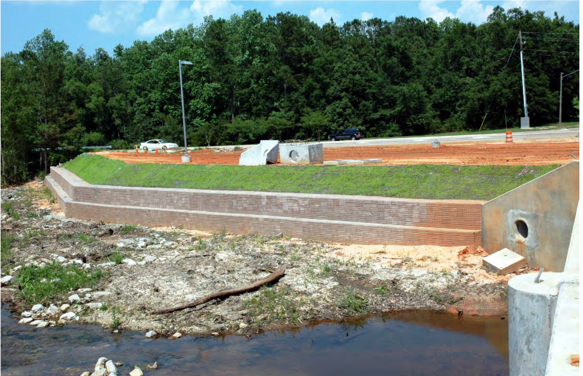
A VIEW OF THE ECOMATTRESS OVER THE CONCRETE BLOCKS FACED GABION WALL
