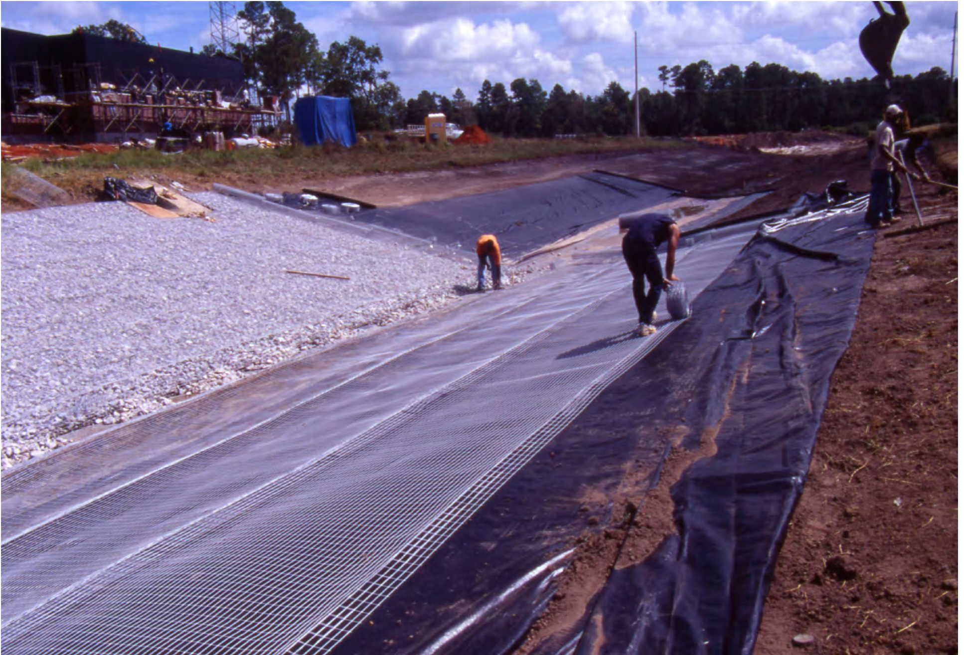
UNROLLING CONTINUOUS EDGE PANEL
