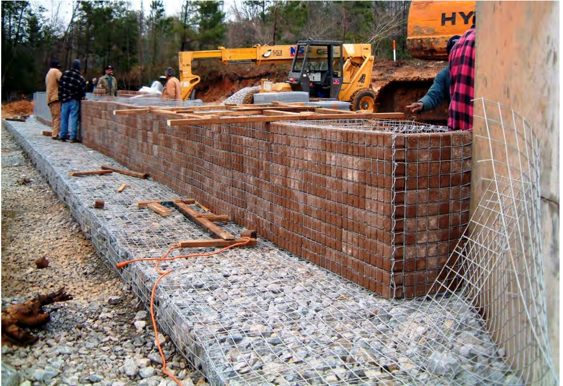
CONCRETE “RAGAZZO” BLOCKS WALL FACING
