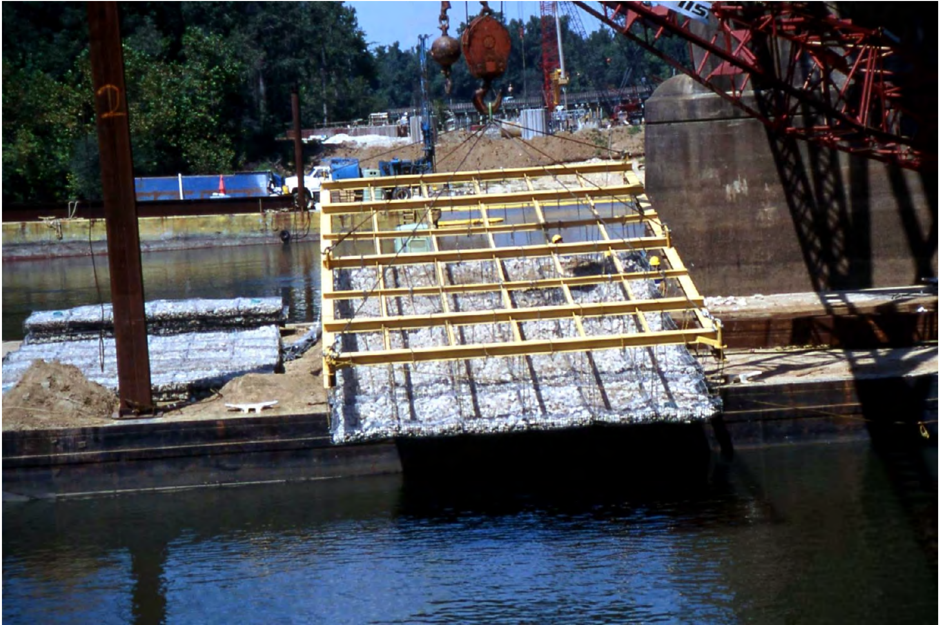
GABION MATTRESS UNDERWATER PLACEMENT
