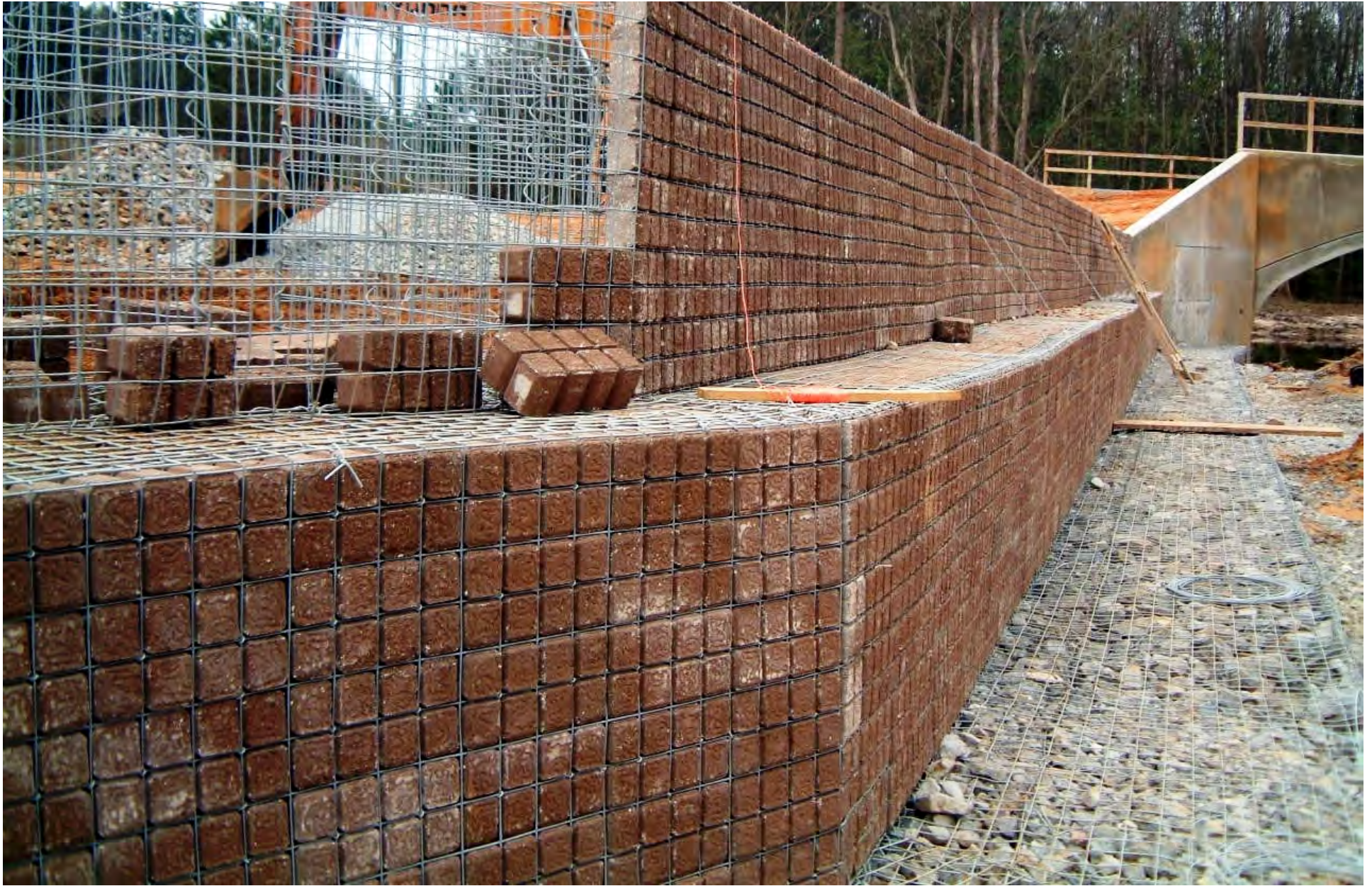
CORNER DETAIL OF CONCRETE “RAGAZZO” BLOCKS FACED GABION WALL
