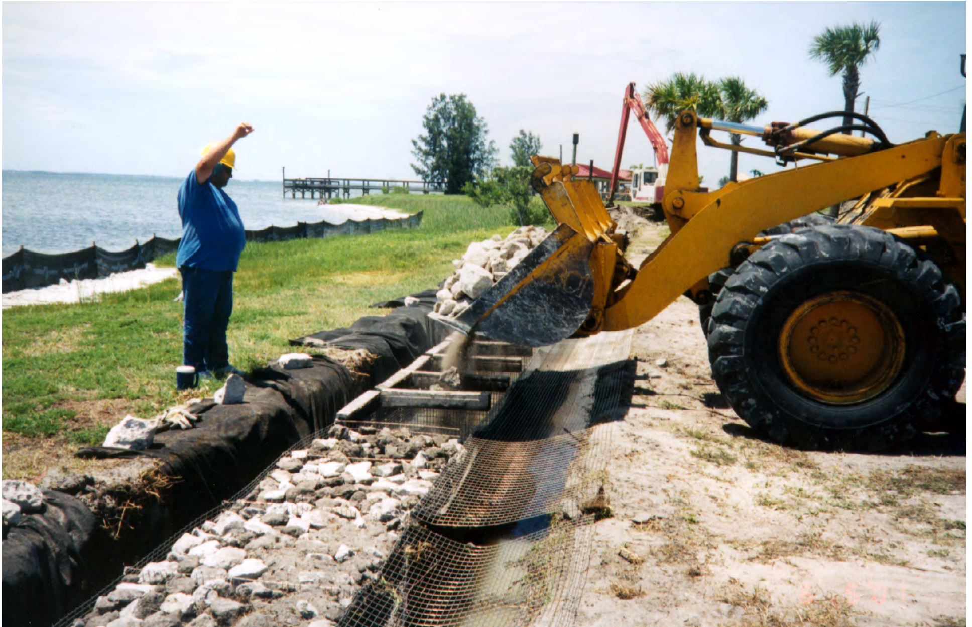
GABION WALL WRAPPED IN GEOTEXTILE AND PLACED BELOW THE BEACH LEVEL
