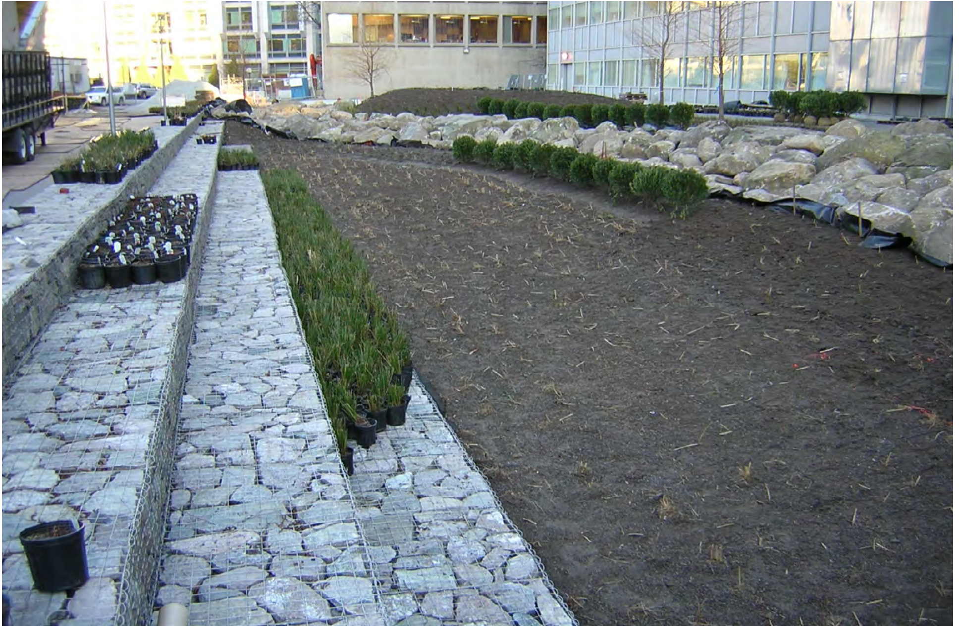
M.I.T. CAMPUS CAMBRIDGE, MA S. S. WIRE GABIONS LANDSCAPING DETAIL
