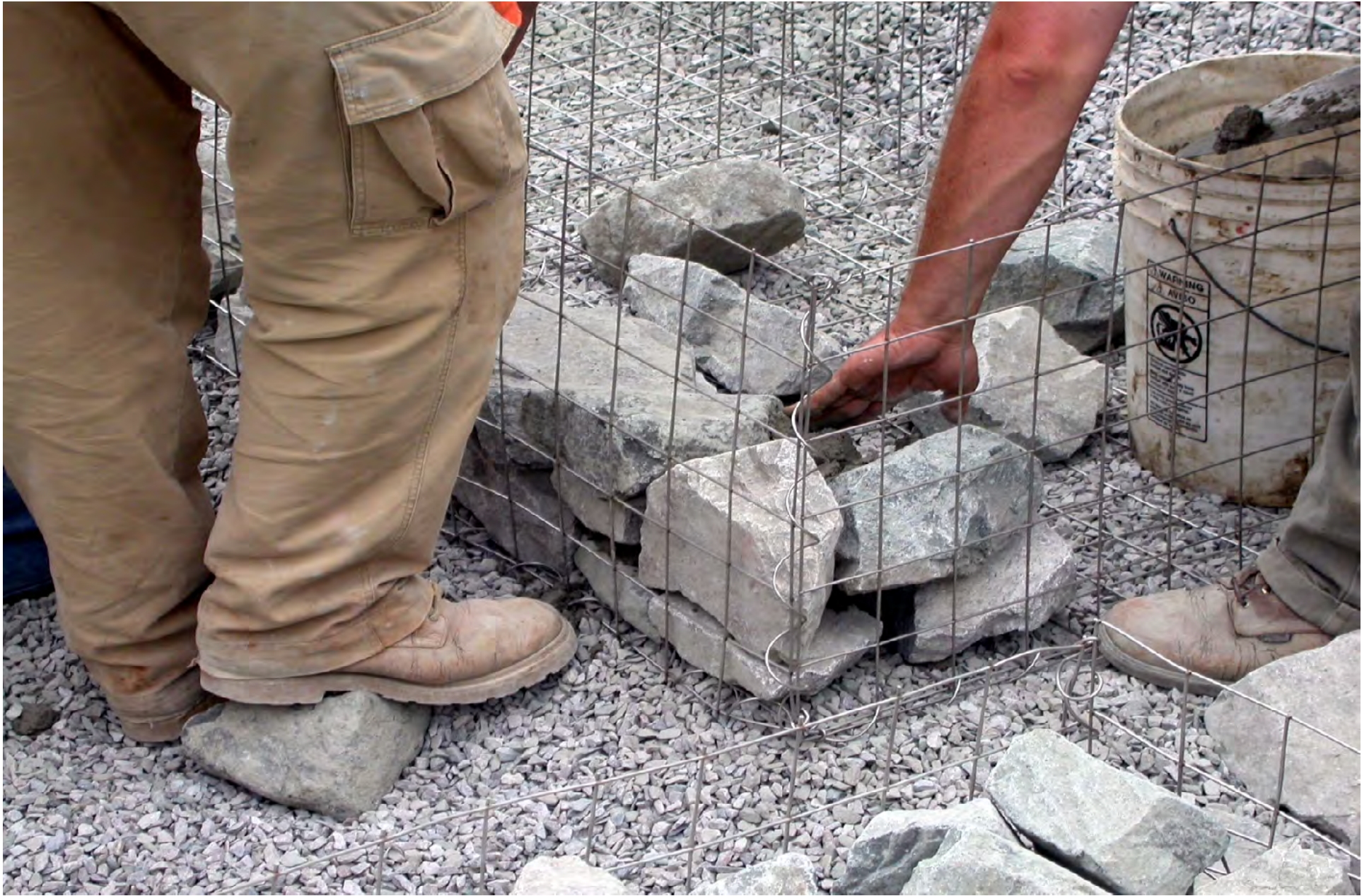
M.I.T. CAMPUS - S. S. GABION WALLS CONSTRUCTION DETAIL
