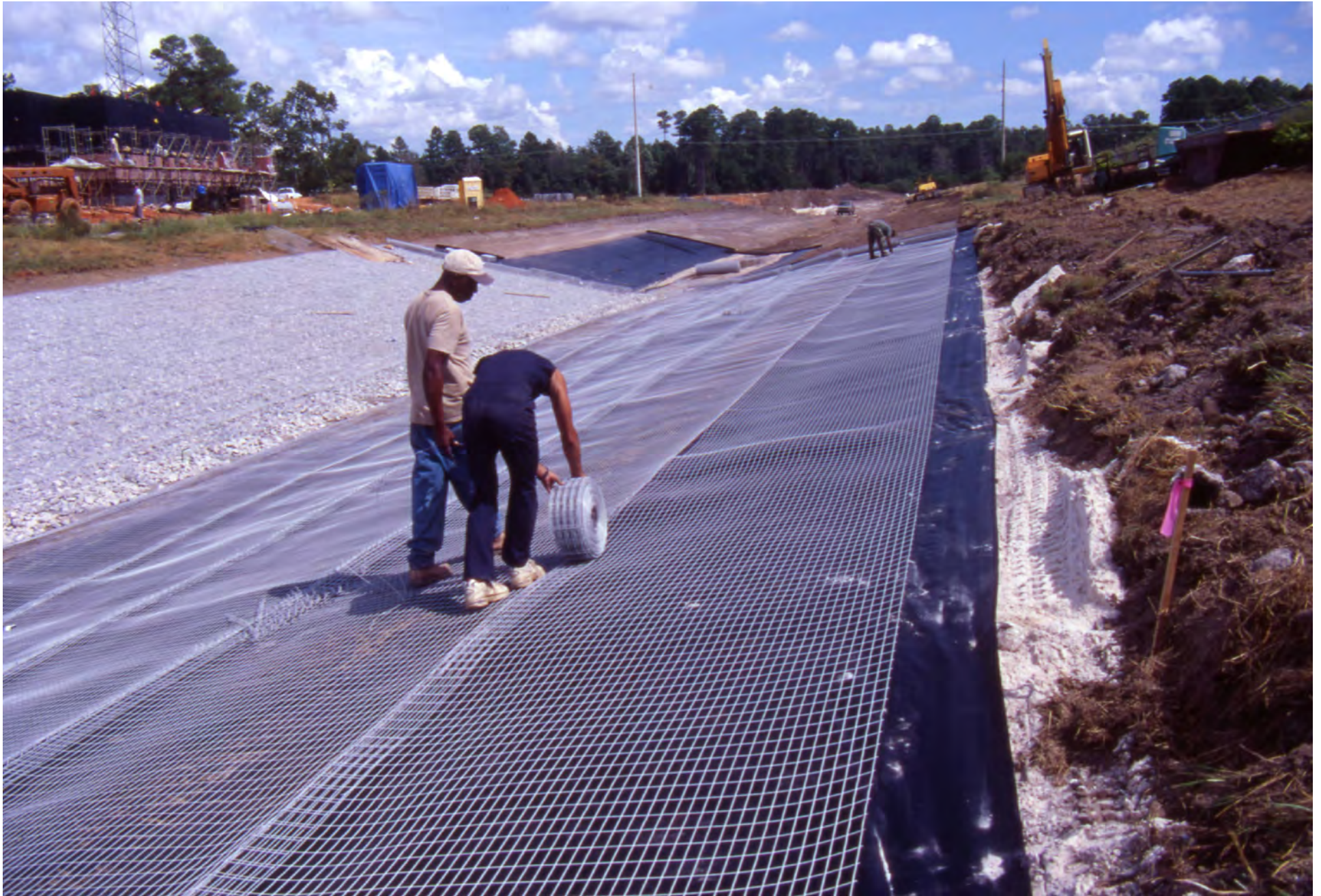
UNROLLING CONTINUOUS DIVIDER PANEL
