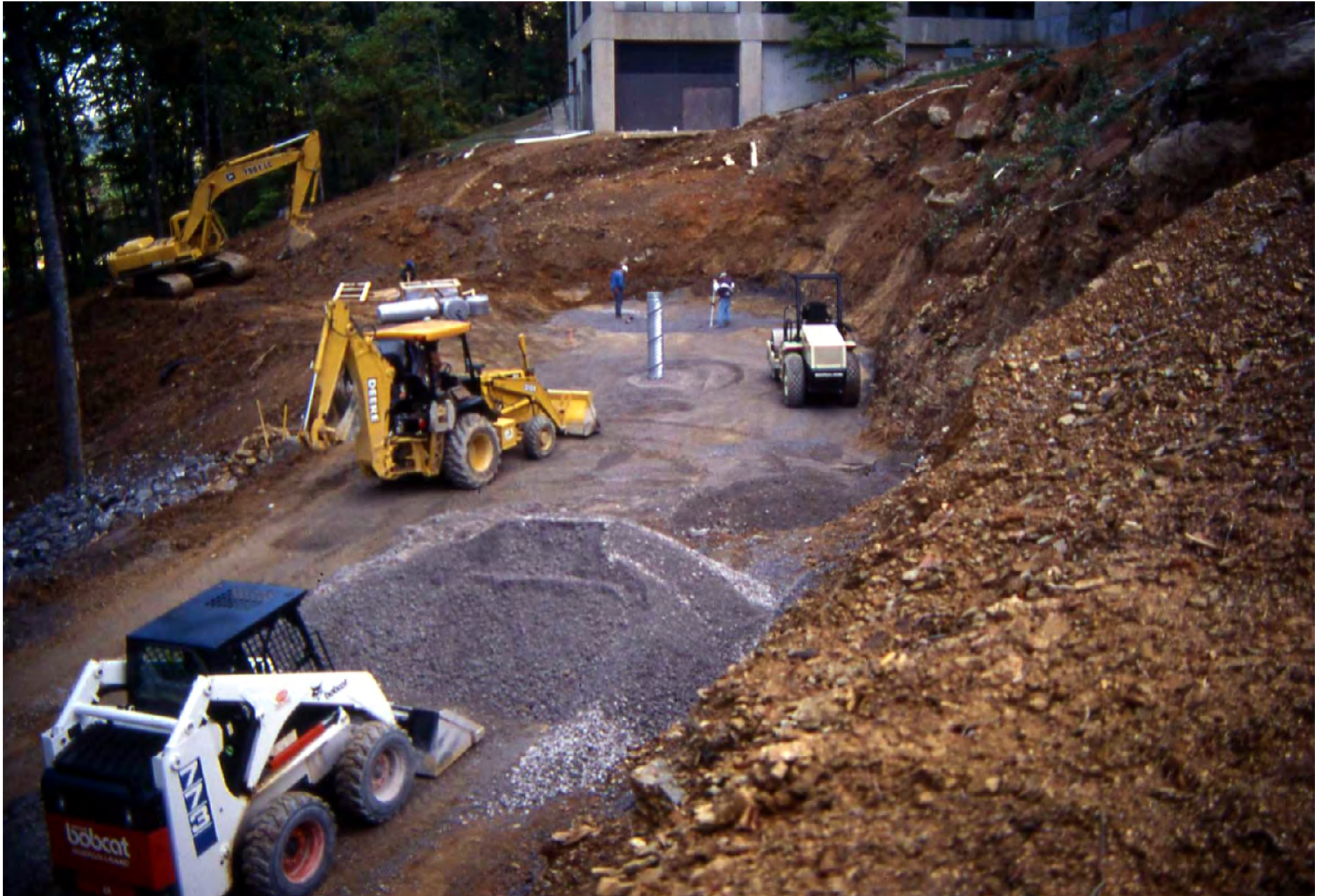
SITE EXCAVATED-DRAIN PIPE-GRAVEL BEDDING
