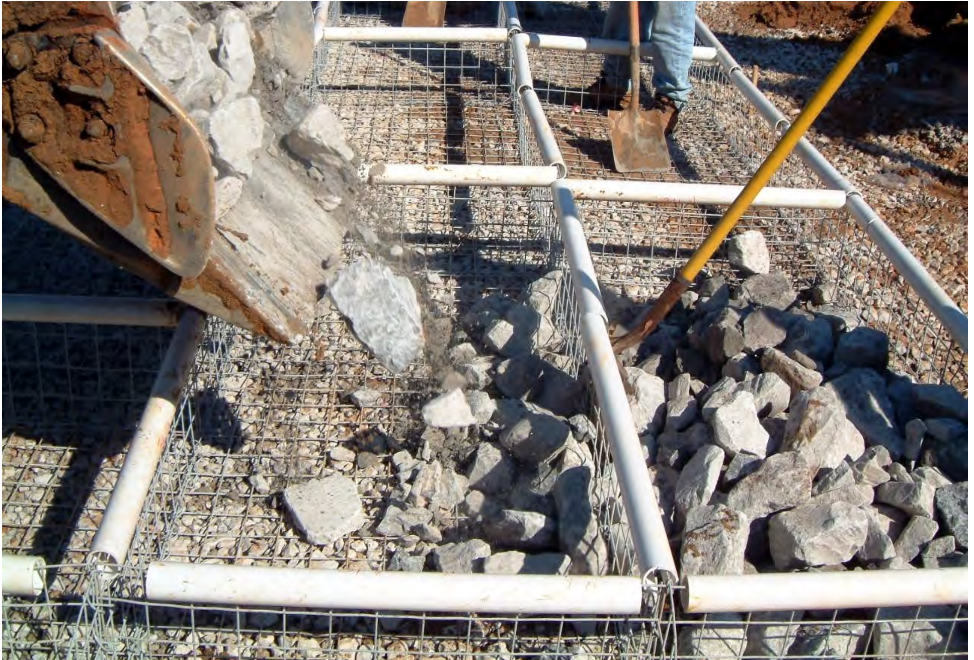
ROCK-FILLING THE 12" GABION MATTRESS
