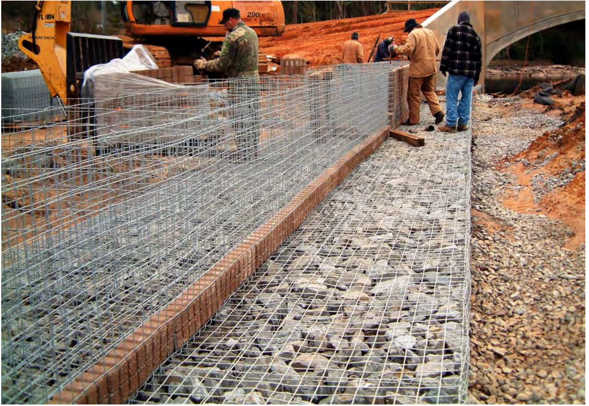
CONCRETE BLOCKS PLACEMENT
