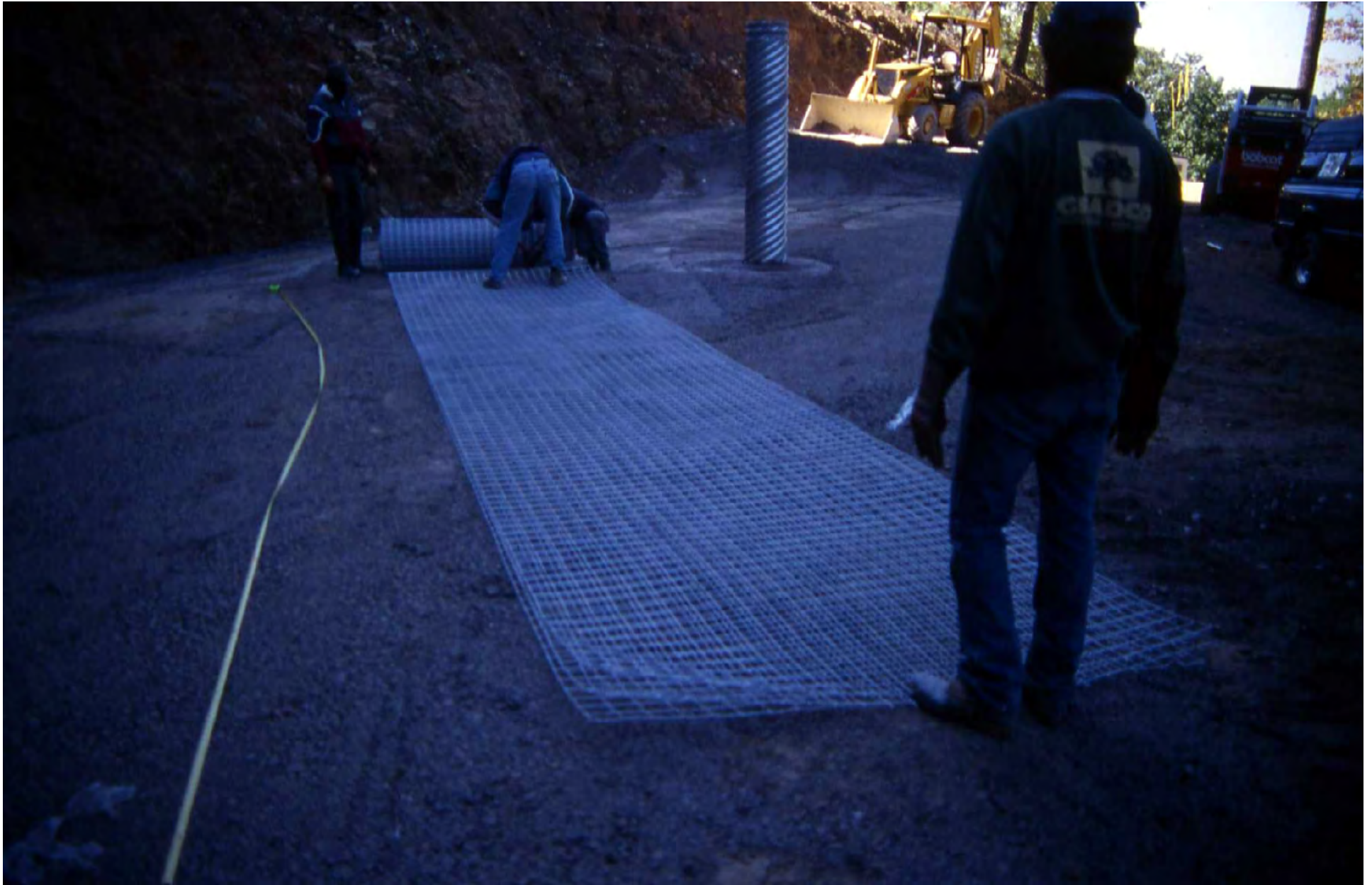
33' LONG X 6' WIDE PANELS CUT FROM "ROLL-STOCK" FOR BASE COURSE SOIL REINFORCING
