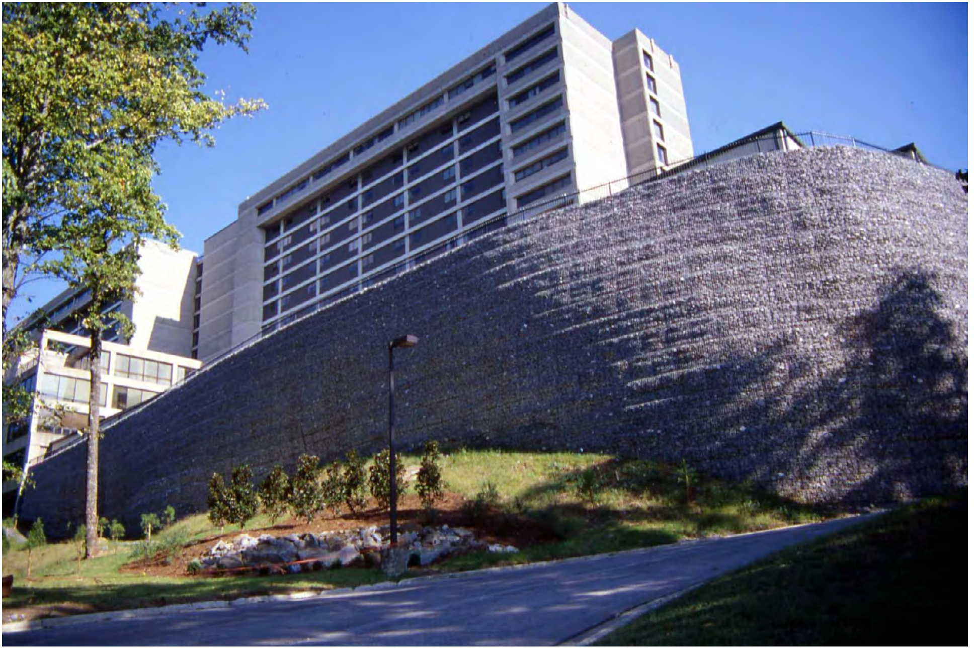
MSE GABION WALL COMPLETED MARCH 1998
