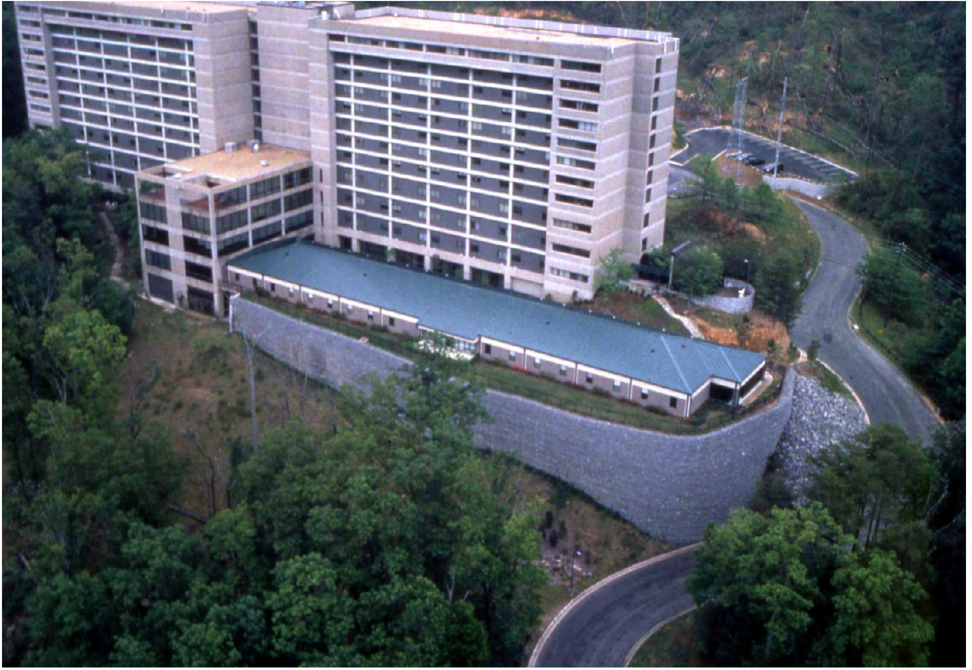
AERIAL VIEW OF MSE GABION WALL & BLDGS.
