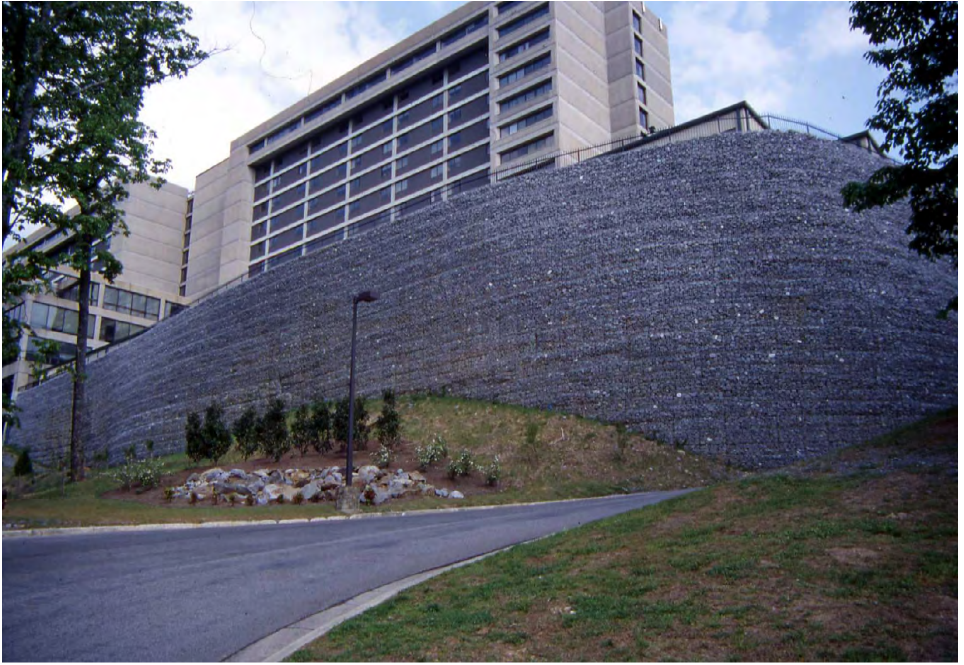
48' HIGH MSE GABION WALL COMPLETED 03/1998
