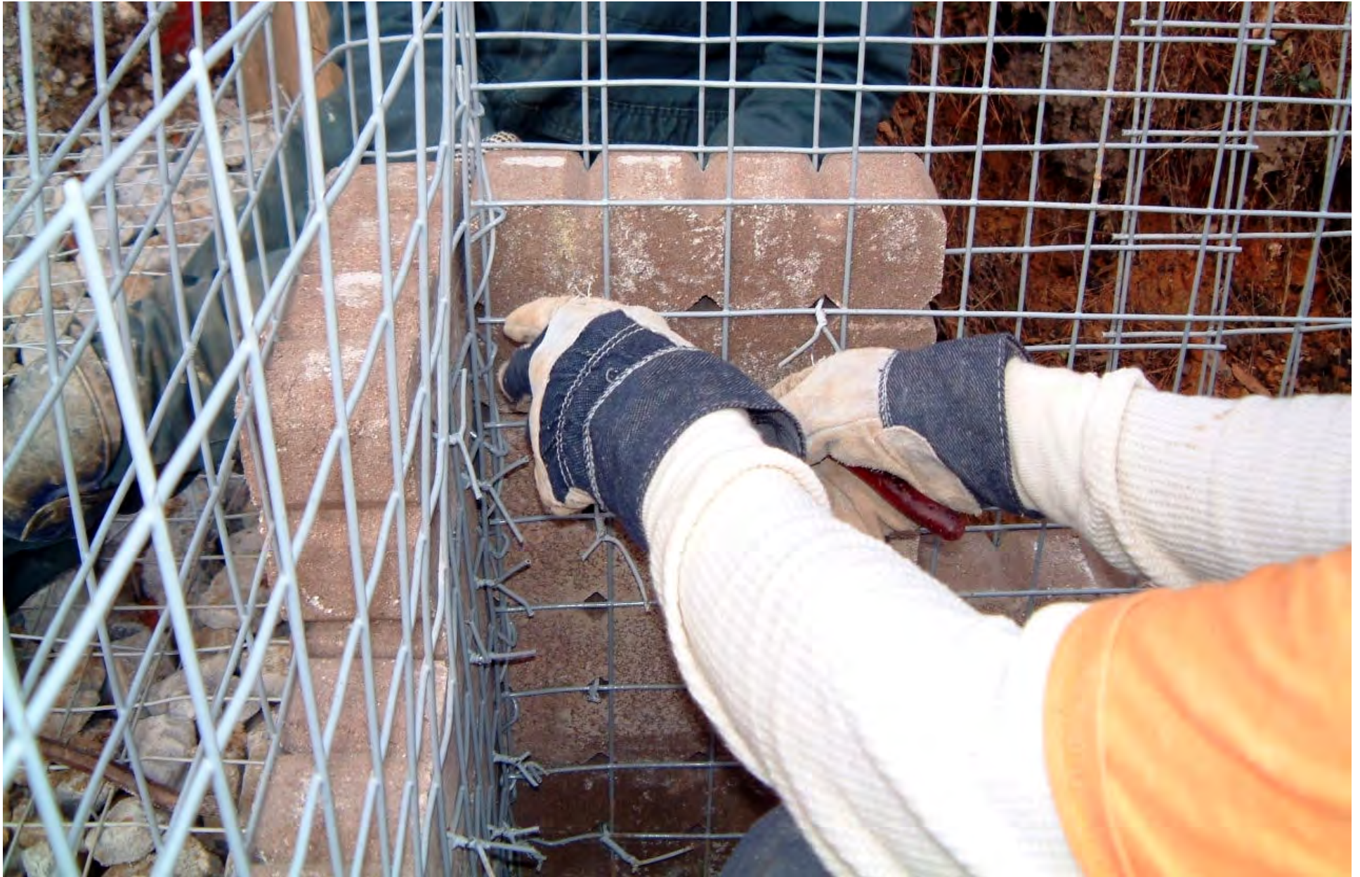
SHAPED WIRE TIES FASTENED TO REAR MESH PANEL
