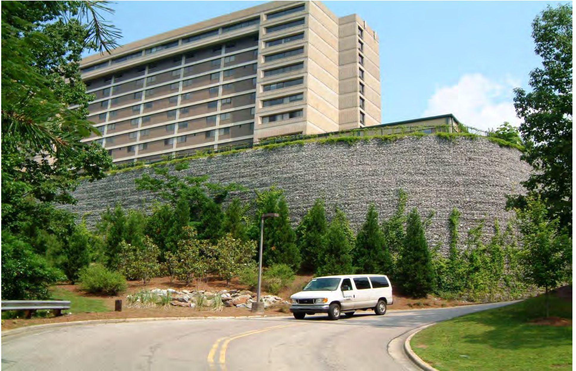
MSE GABION WALL AS SEEN IN JUNE 2005, SEVEN YEARS AFTER COMPLETION
