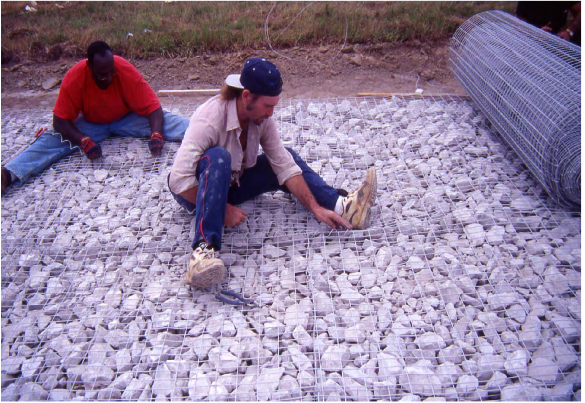
SPIRAL CONNECTING LIDS TO DIAPHRAGMS
