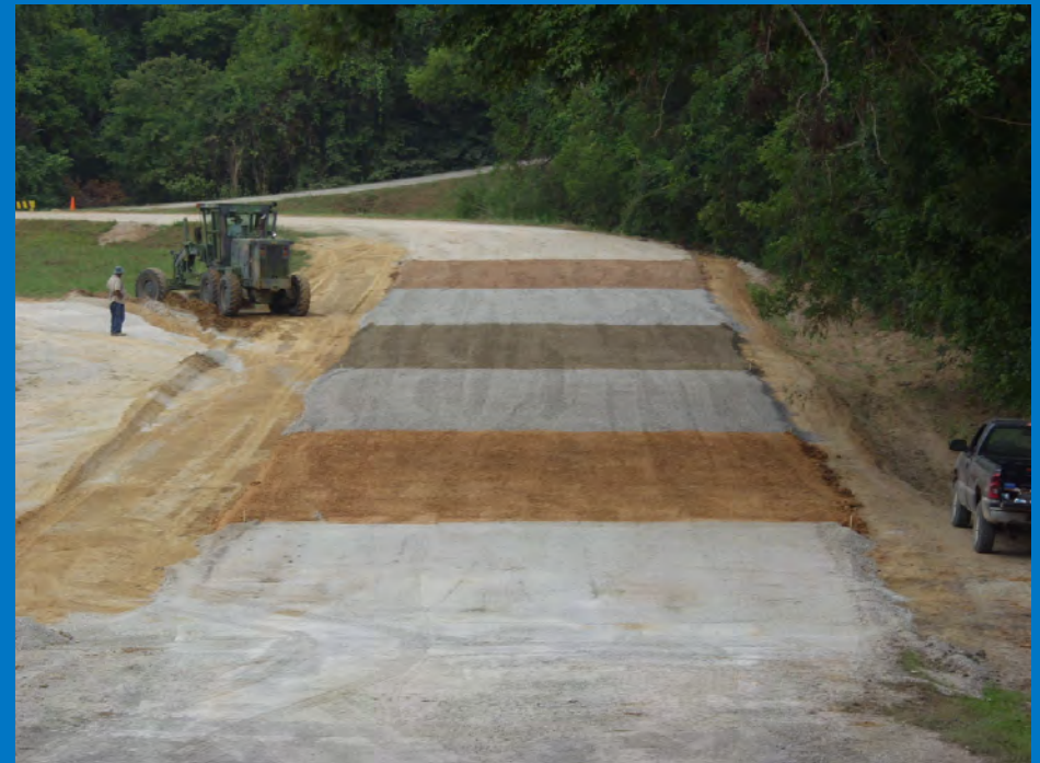
New Construction Test Section
