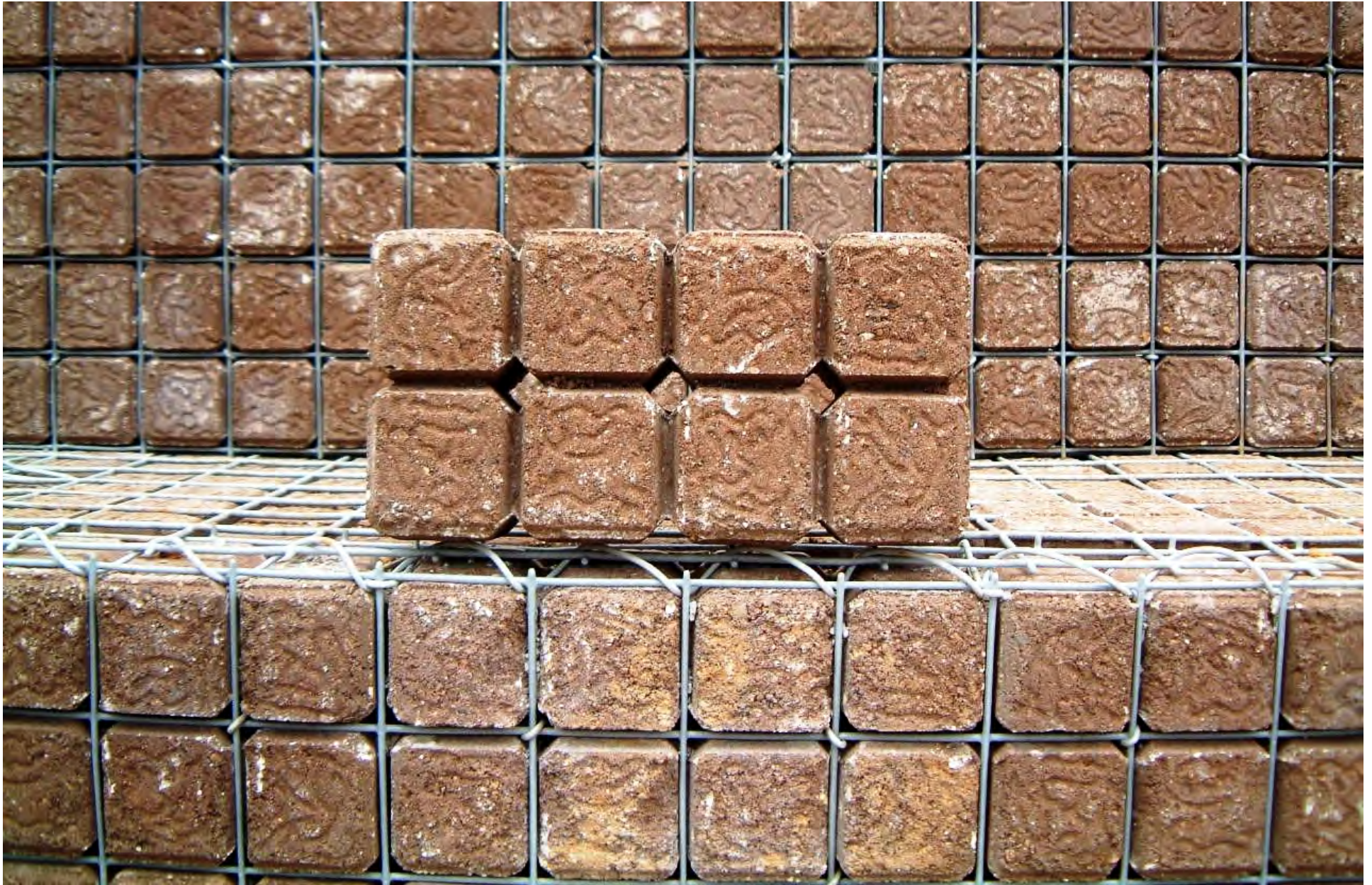
DETAIL OF A CONCRETE BLOCK NOTICE THE DRAINAGE HOLES
