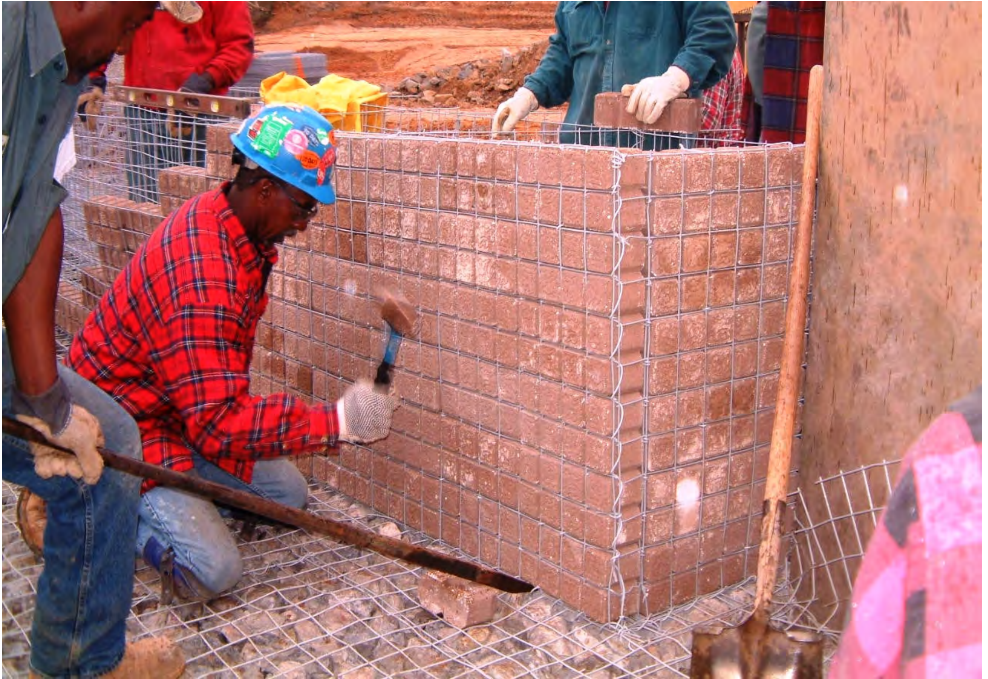
LEVELING THE CONCRETE BLOCKS FACING
