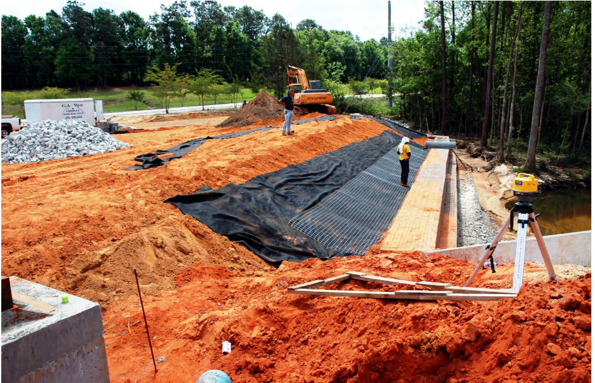
PLACING GEOTEXTILE & “ROLL-STOCK” PVC MESH FOR THE ECOMATTRESS BASE
