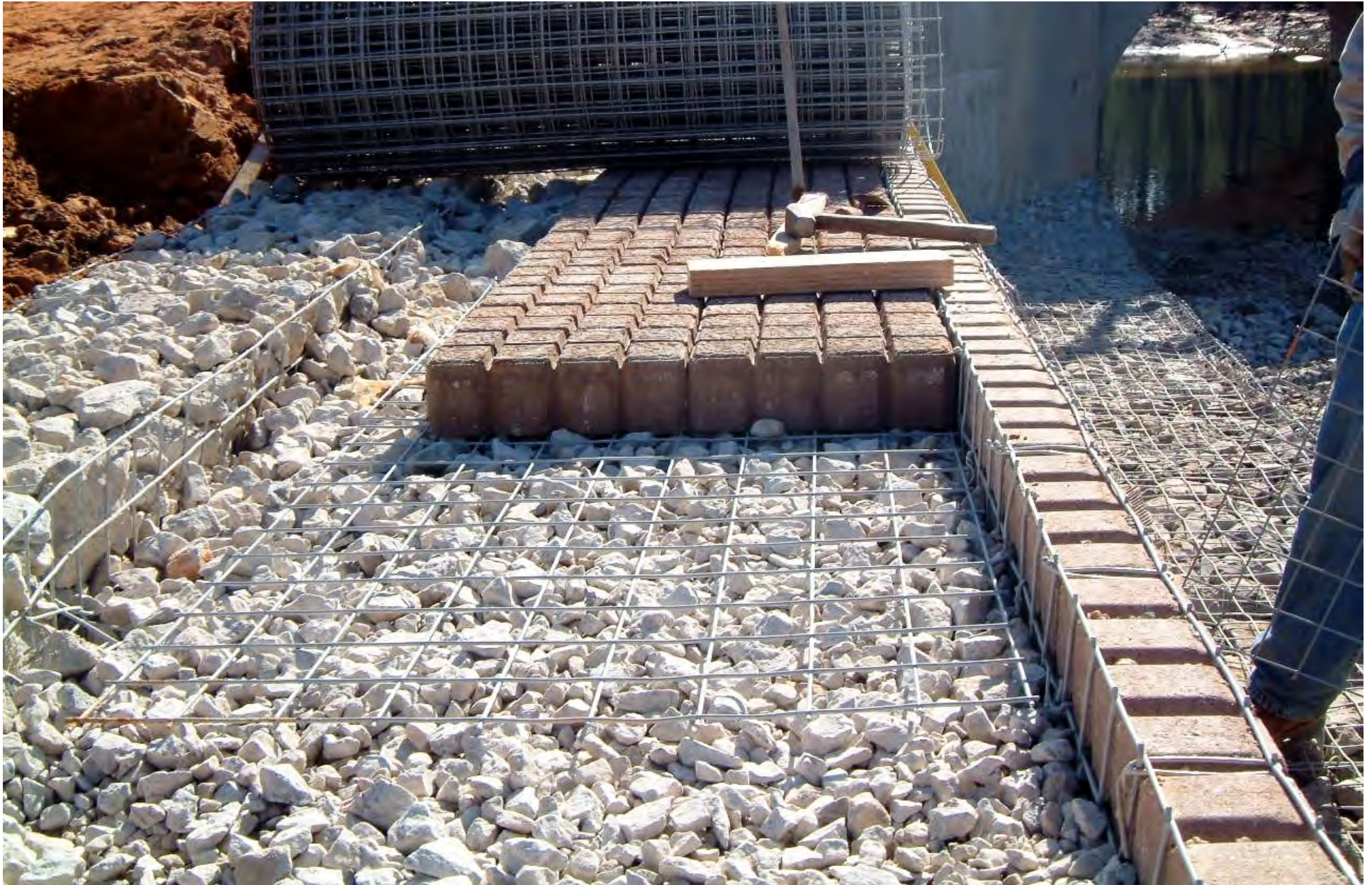
BLOCKS PLACED HORIZONTALLY ON GABION WALL SETBACK
