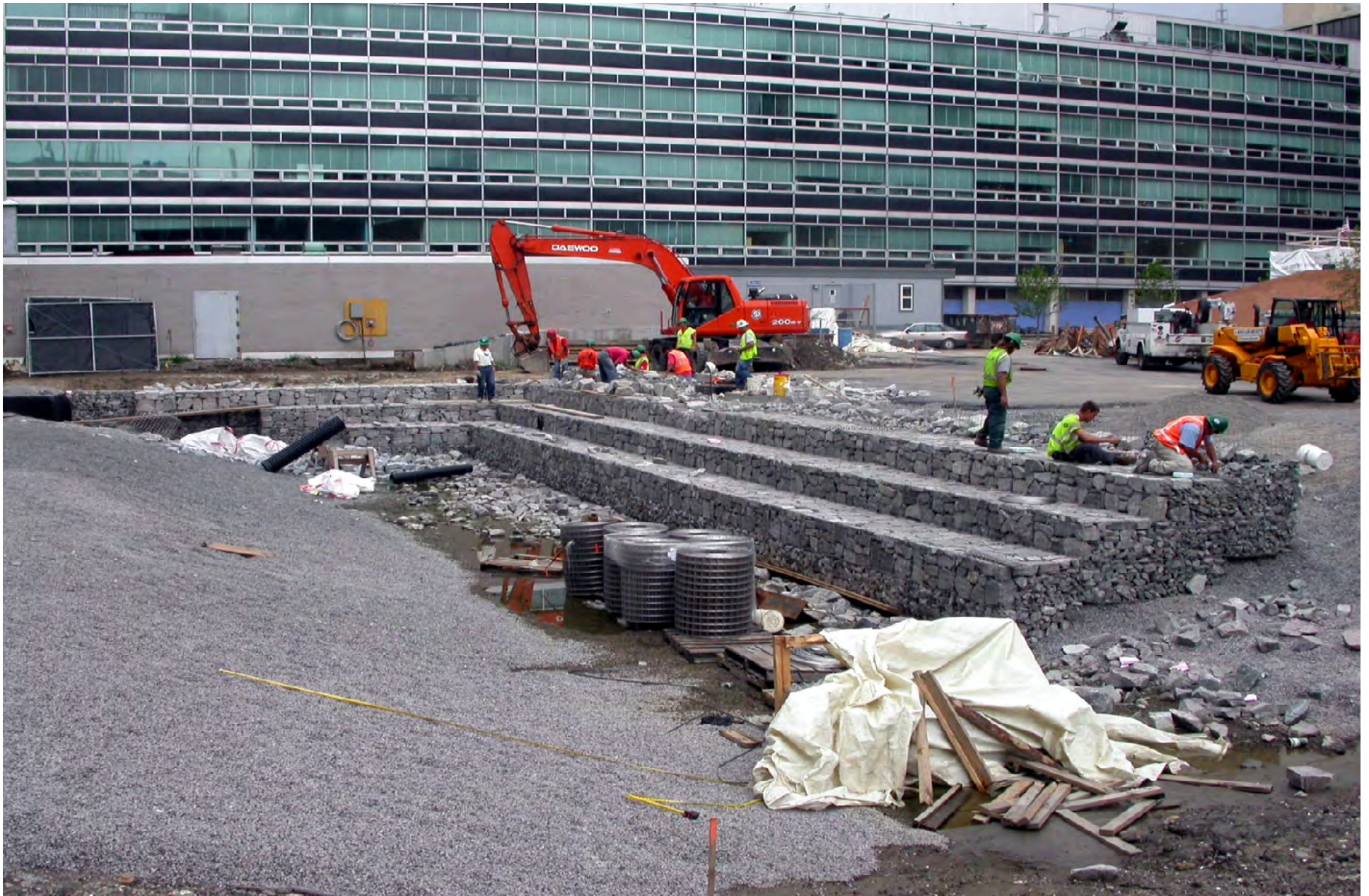
STAINLESS STEEL WIRE GABIONS AT M.I.T. CAMPUS LANDSCAPING STRUCTURES
