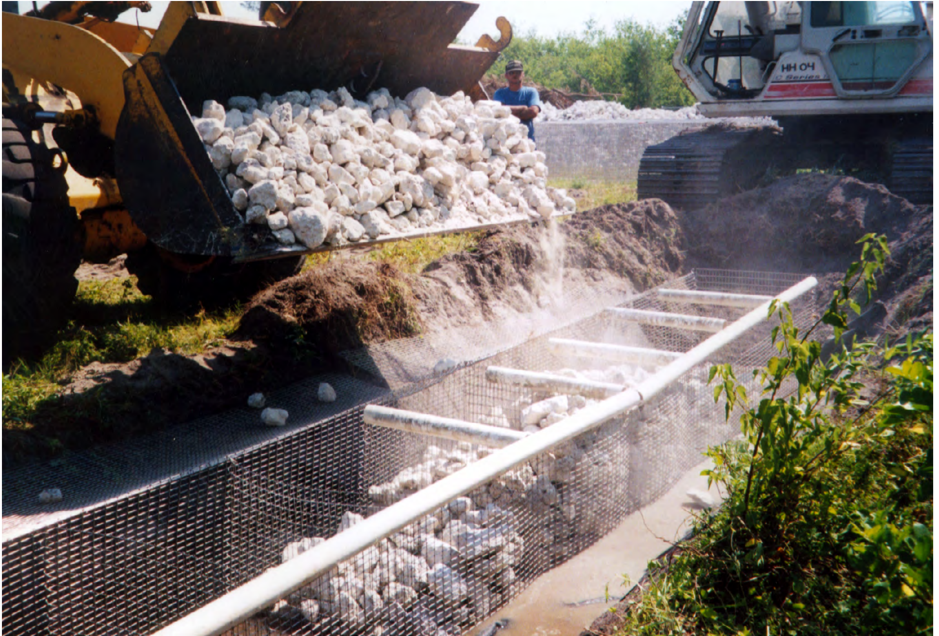
GABION ROCK-FILLING
