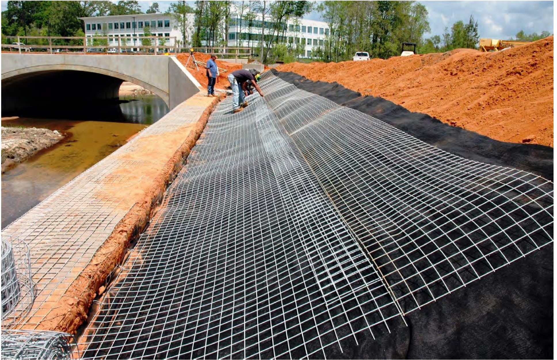
FORMING JOINTLESS ECOMATTRESS WITH BASE & LONGITUDINAL DIVIDER PANELS
