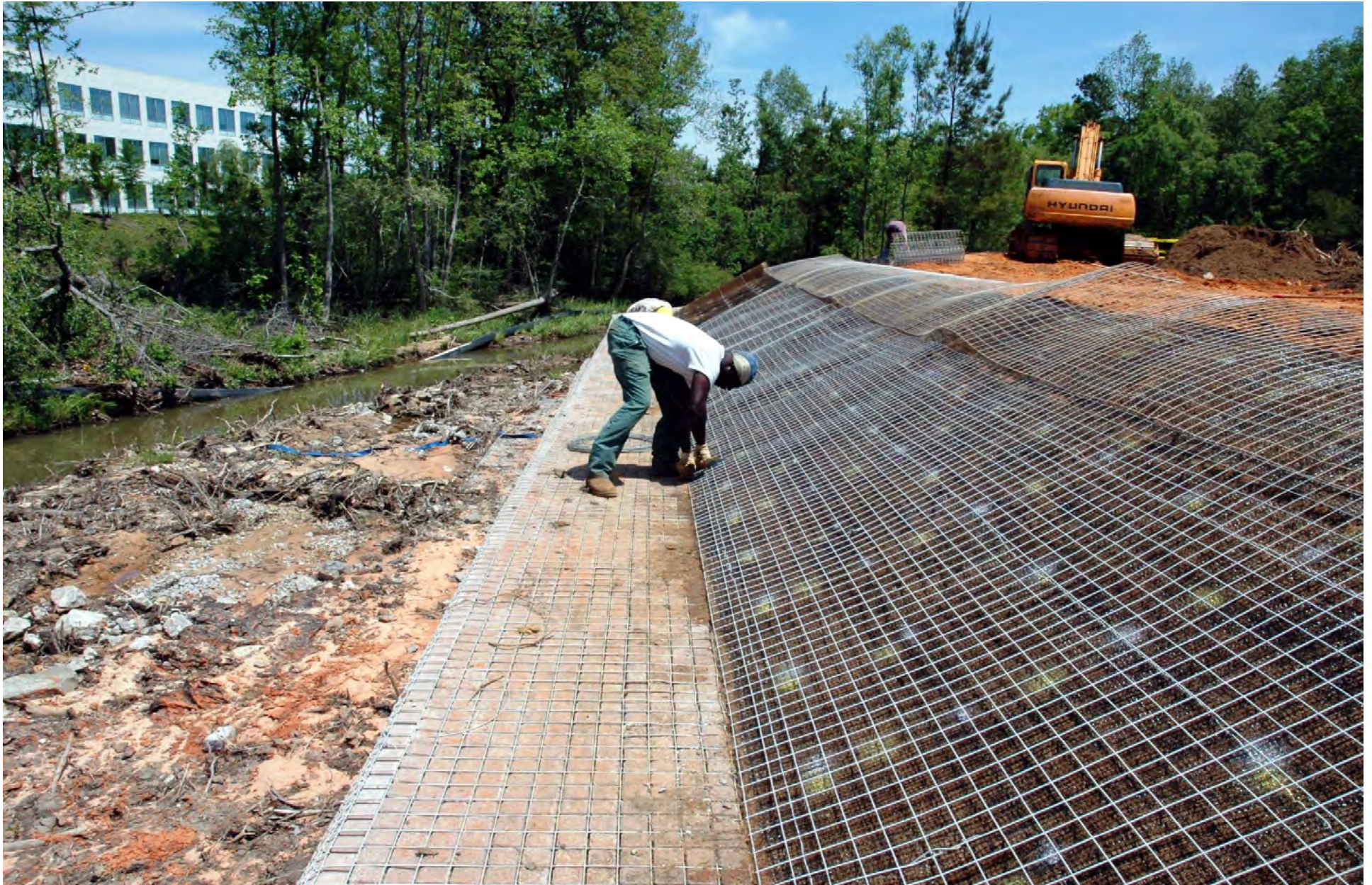
PVC GABION MESH SECURES TOP OF ECOMATTRESS
