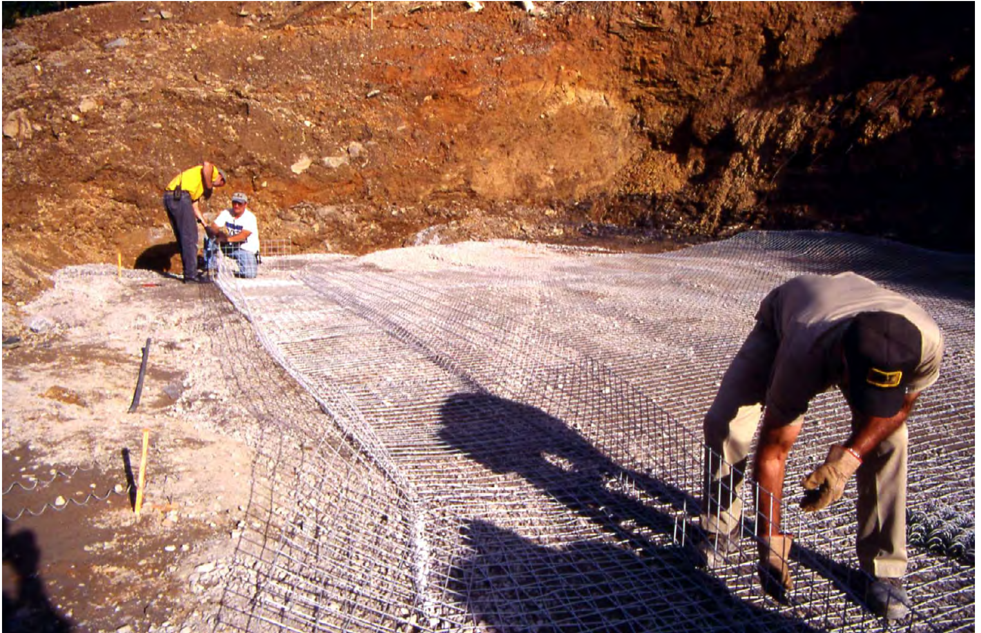
SPIRALS CONNECTING GABION DIAPHRAGMS TO SOIL REINFORCEMENT GRID
