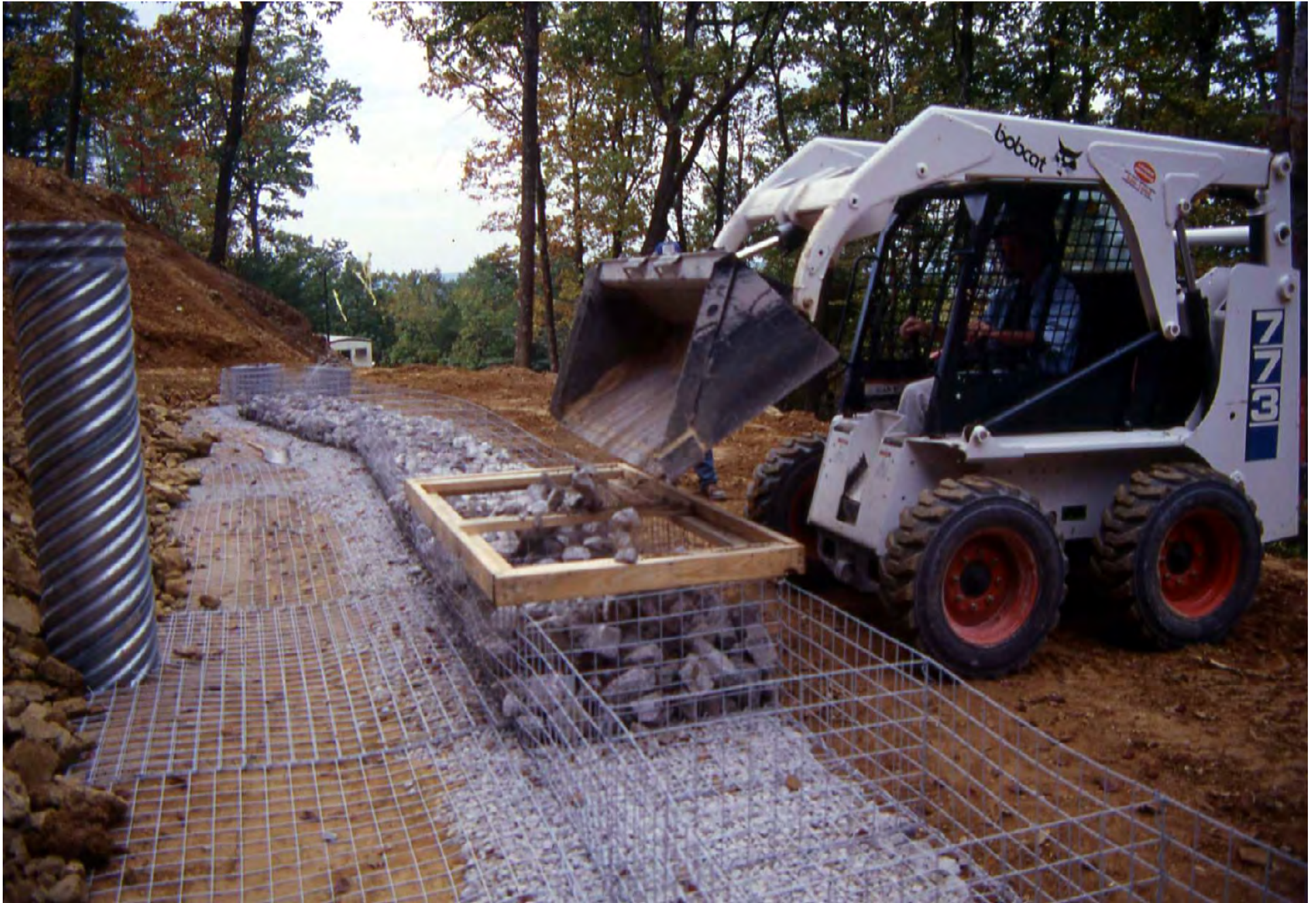
ROCK-FILLING GABIONS WITH 4" TO 8" STONE
