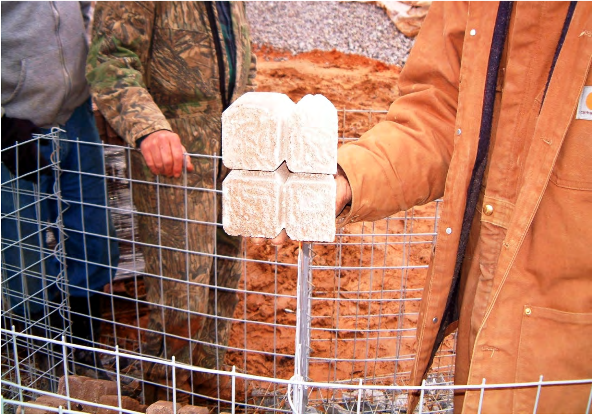
BLOCKS CUT & SHAPED TO FIT CORNERS
