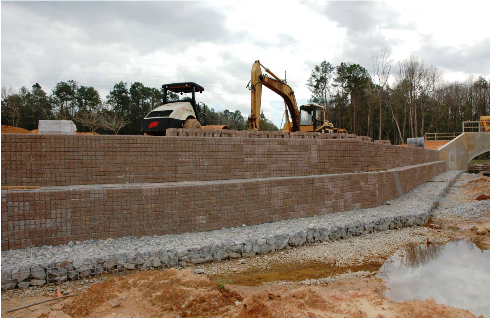
SECTION OF CONCRETE “RAGAZZO” BLOCKS FACED GABION WALL NEAR COMPLETION
