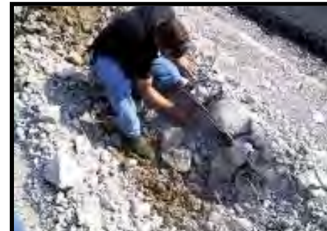
Test Pits – Verify Cracked Pattern
