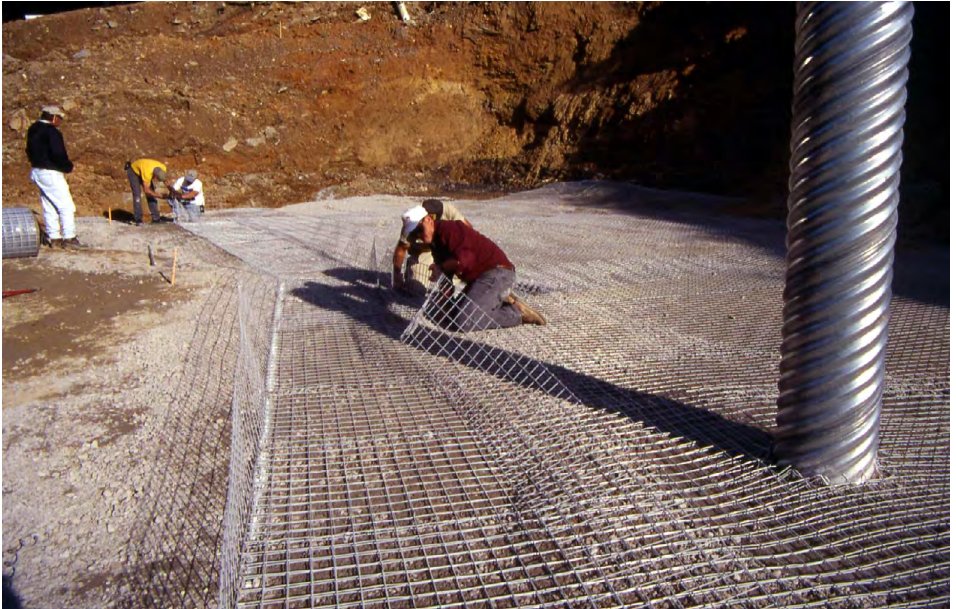
JOINTLESS GABION BASE COURSE ASSEMBLED OVER SOIL REINFORCEMENT PANELS
