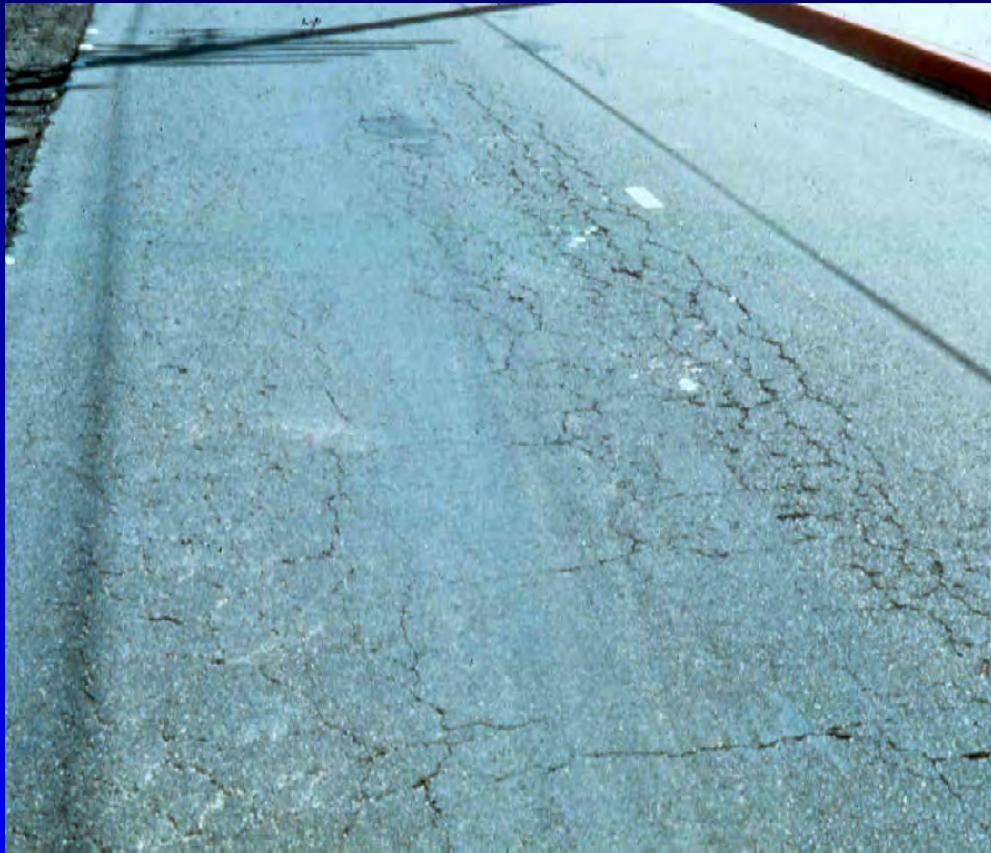
Alligator Cracking
