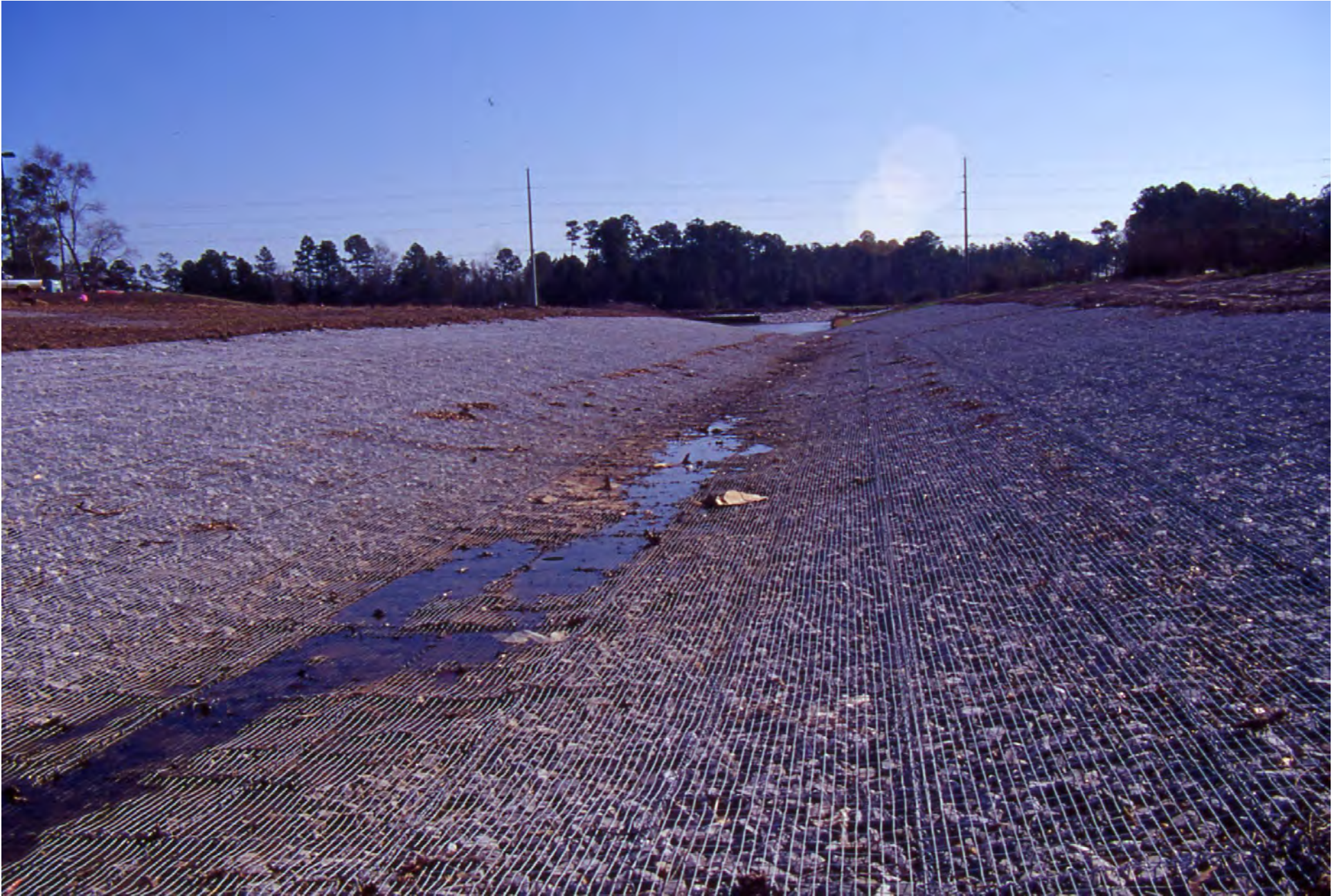
TRAPEZOIDAL CHANNEL REVETMENT - COMPLETED
