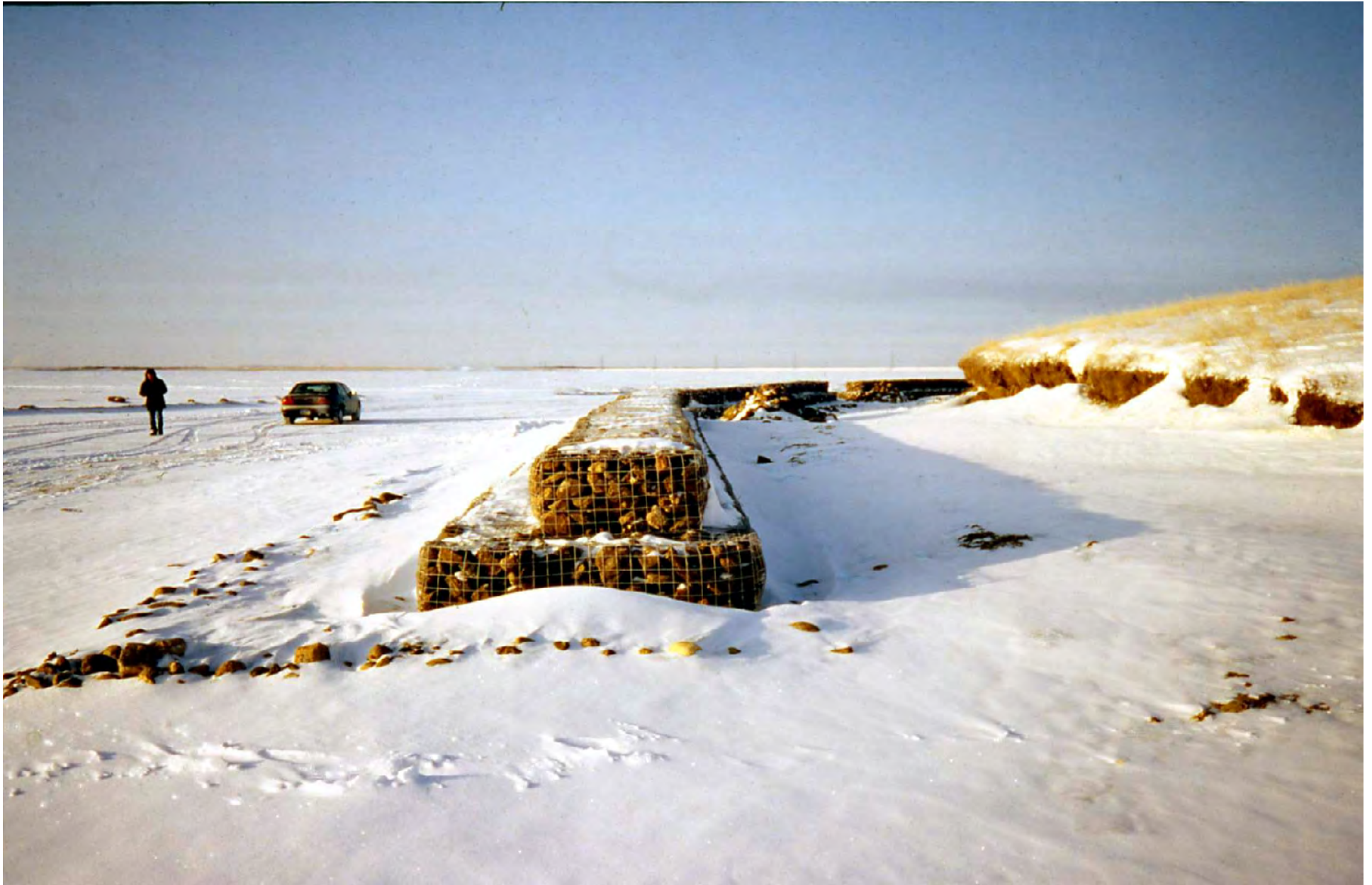
AUDUBON LAKE BIRD SANCTUARY GABION BREAKWATERS BUILT AROUND ISLANDS
