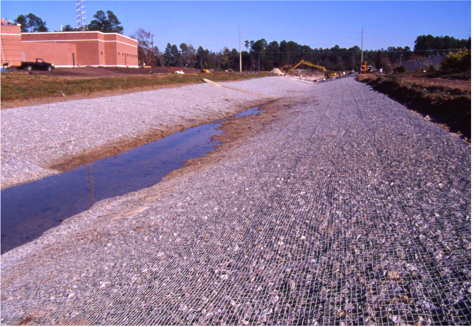
COMPLETED SECTION OF JOINTLESS GABIONS
