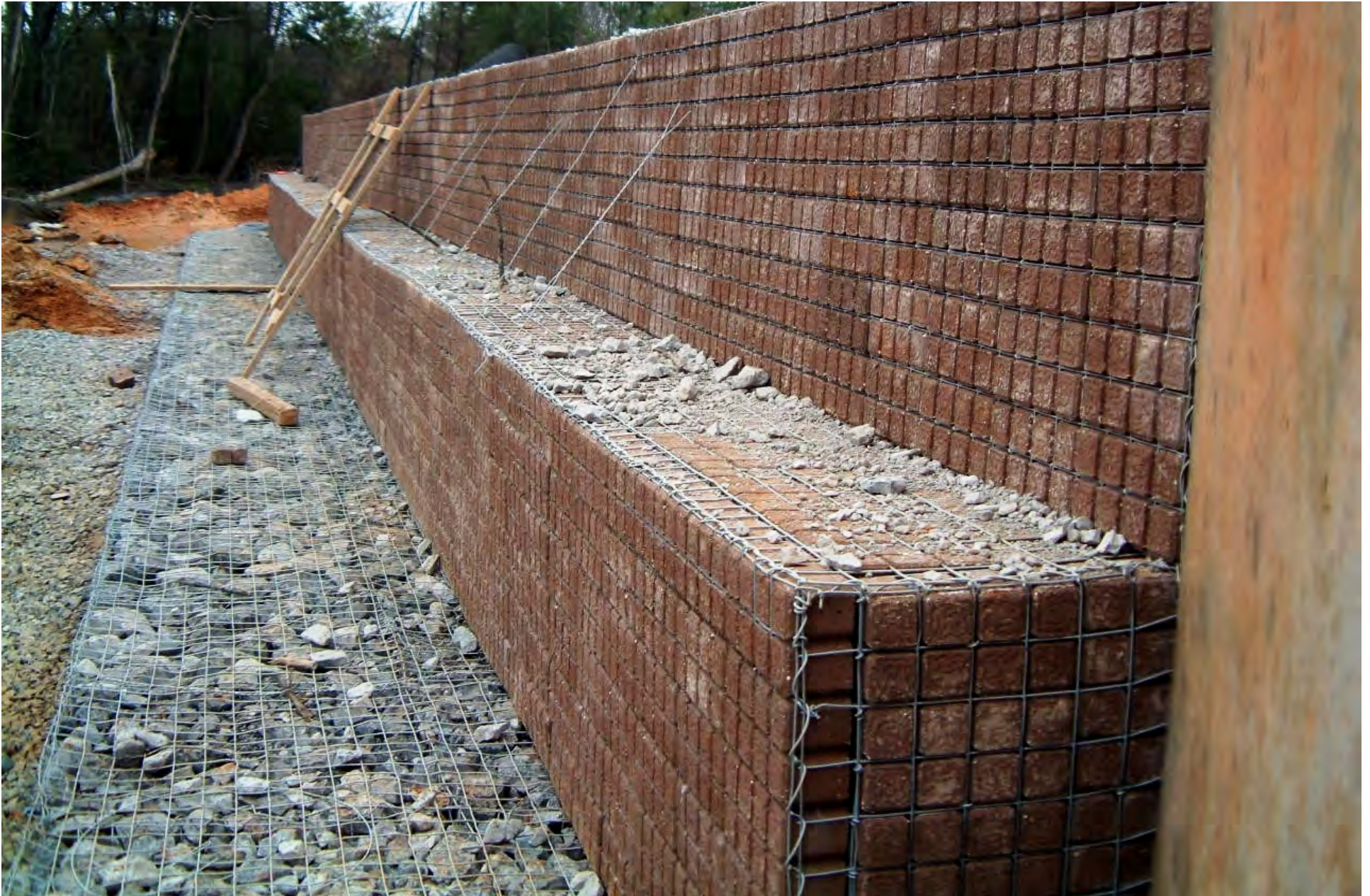
SECOND TIER BLOCKS FACED GABION WALL BEING INSTALLED
