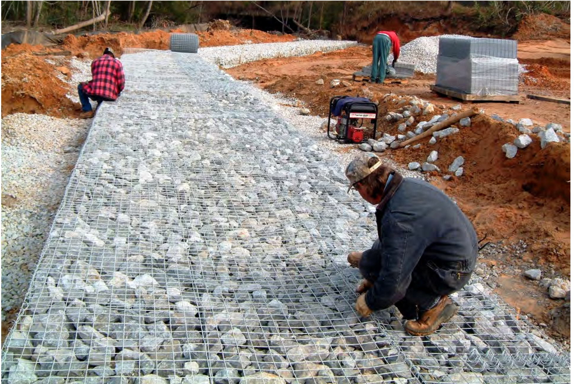
12" THICK MATTRESS READIED FOR WALL BASE
