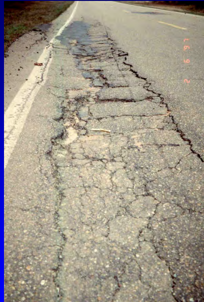
Base Failure
