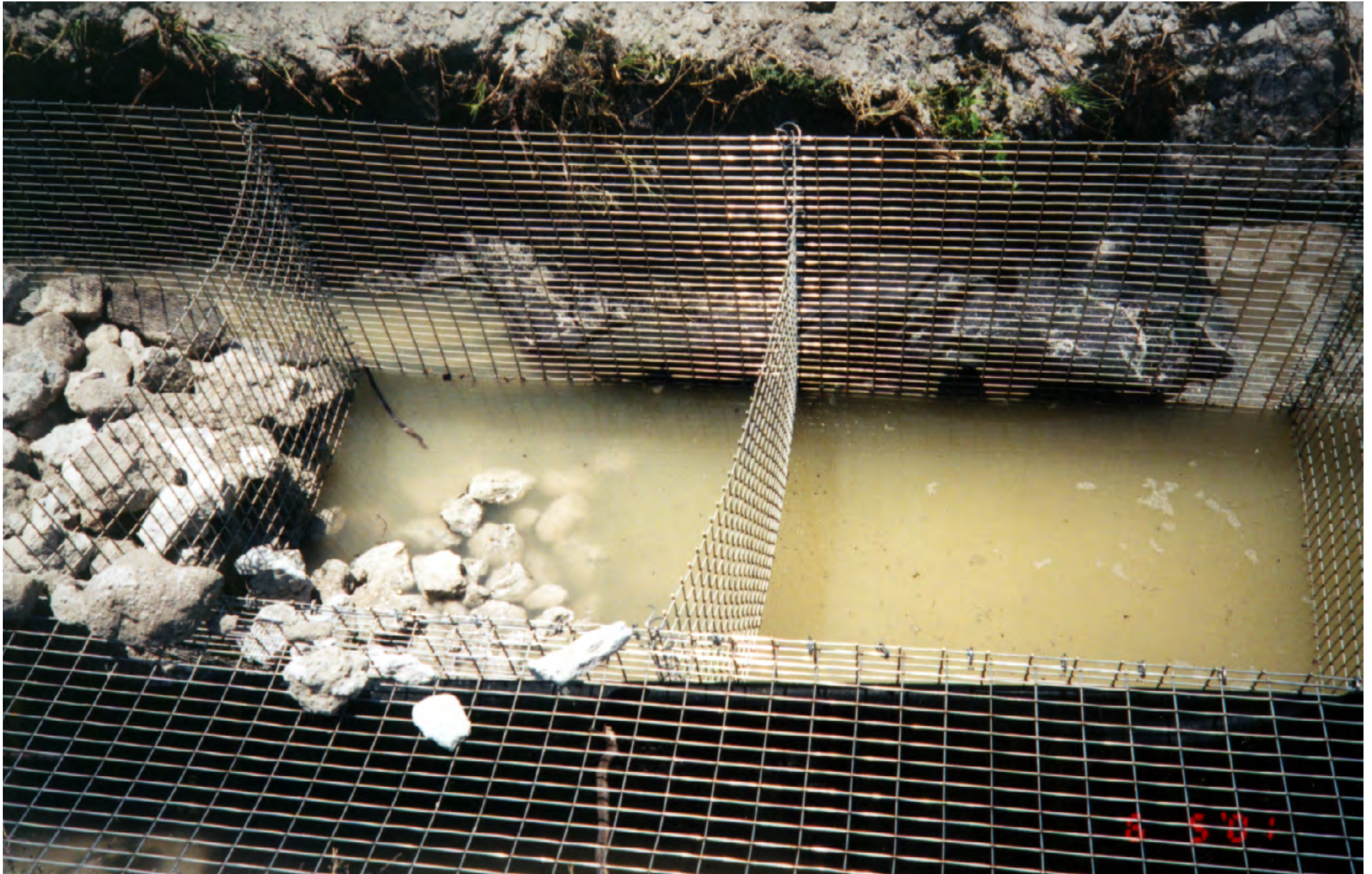
DETAIL OF STAINLESS STEEL GABIONS PLACED BELOW THE WATER TABLE
