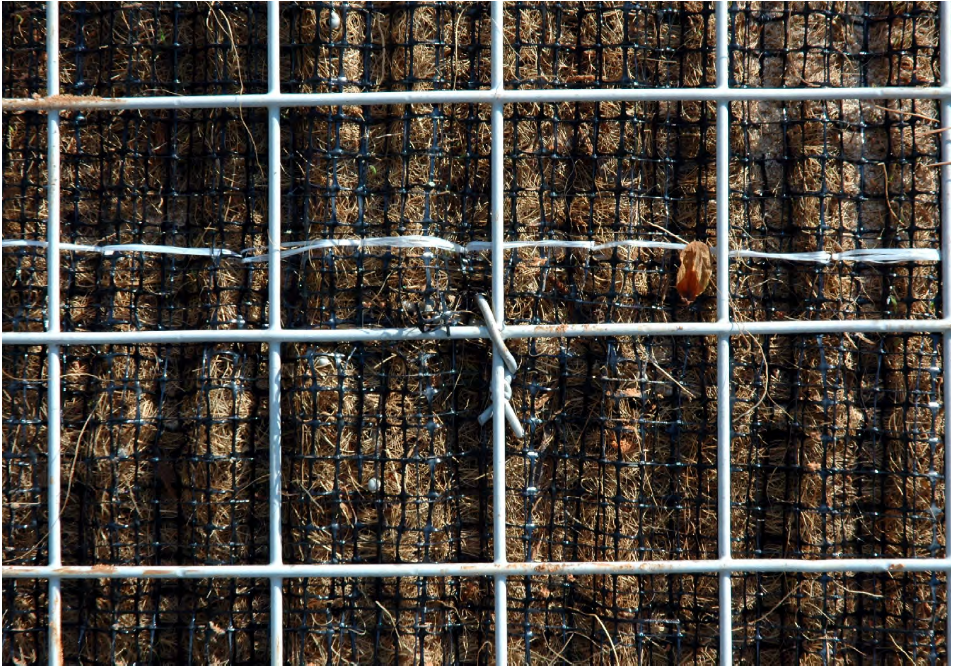
ECOMATTRESS LID FASTENED TO DIVIDER'S TOP
