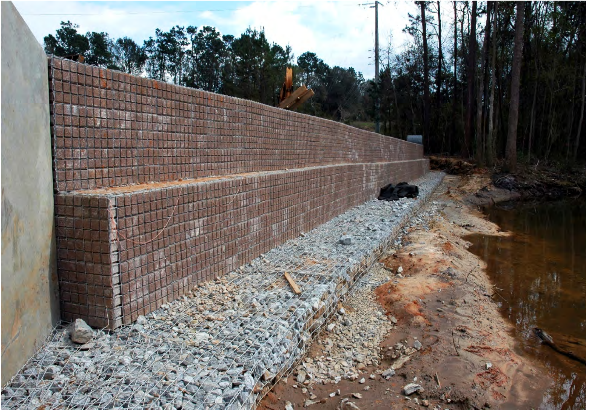
COMPLETED WALL SECTION
