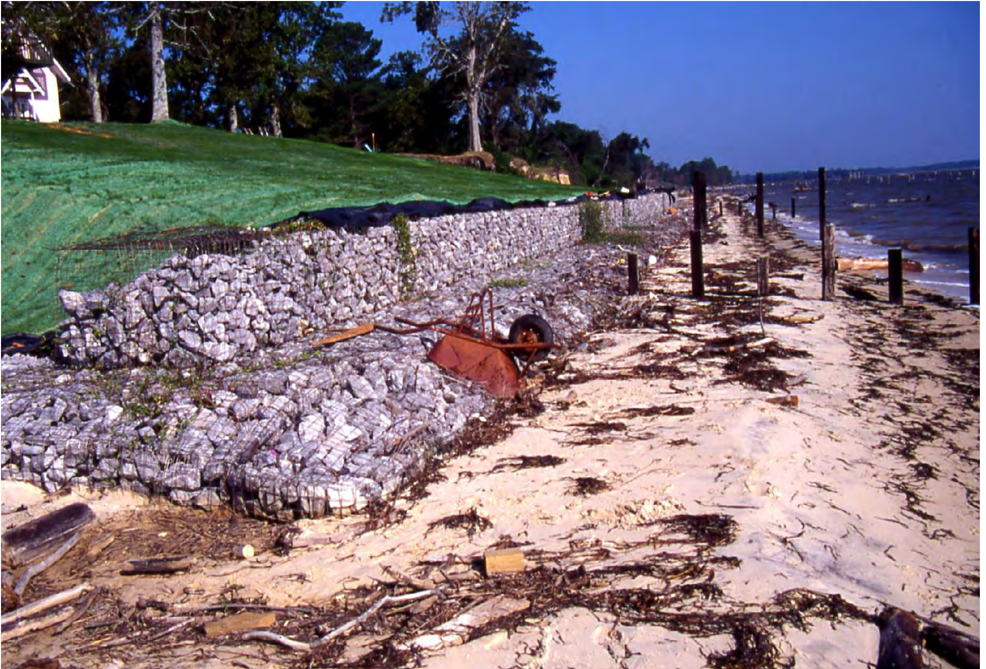
STAINLESS STEEL WIRE GABION SEA WALL
