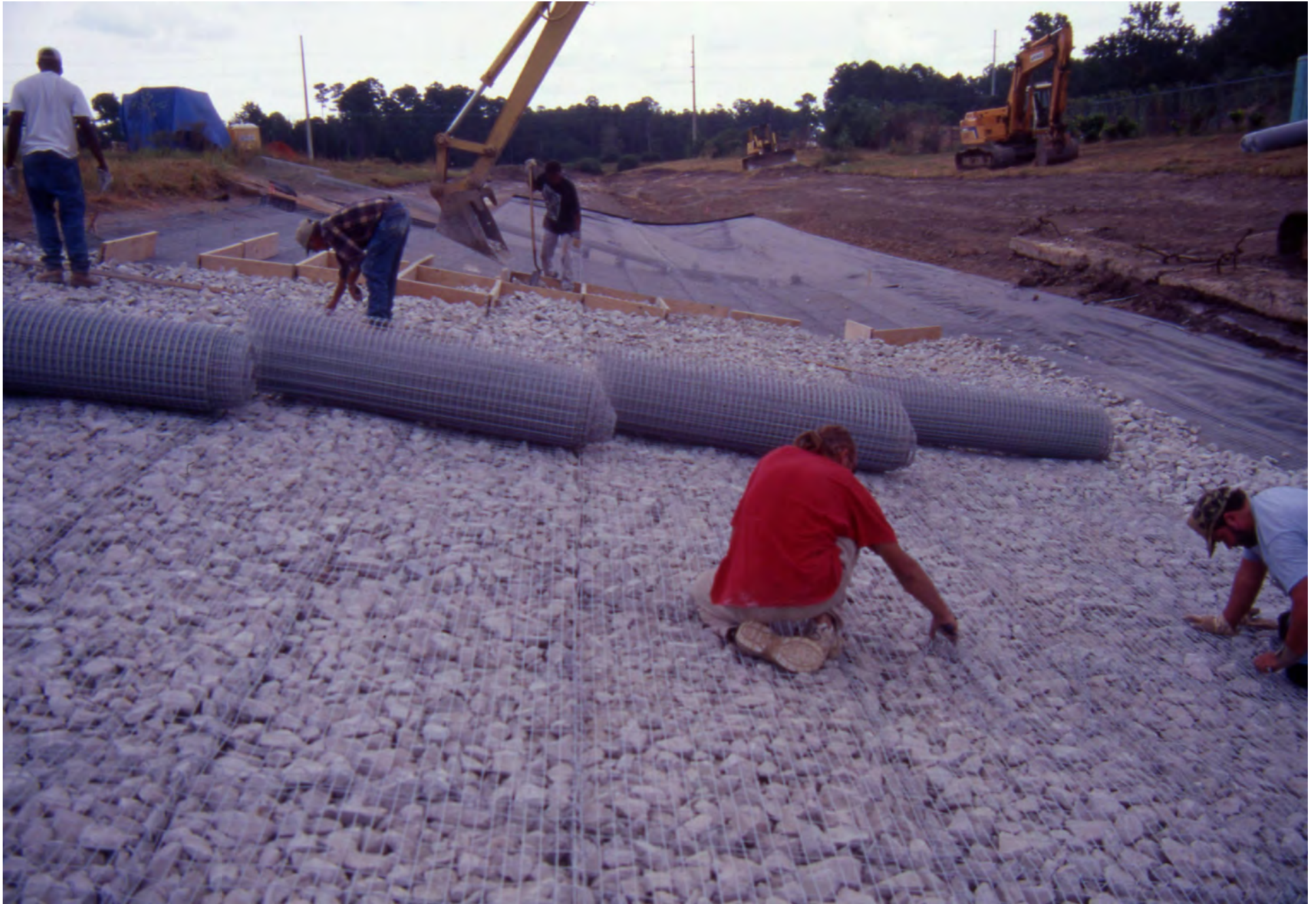
JOINTLESS LIDS FROM “ROLL-STOCK”
