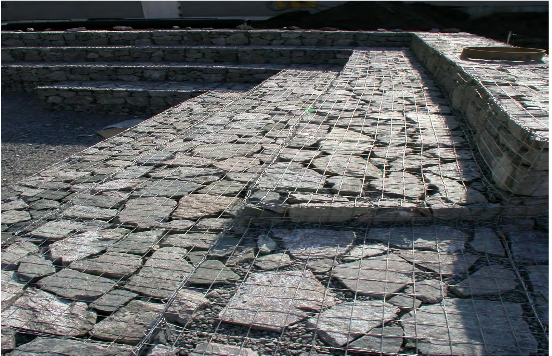
M.I.T. CAMPUS ARCHITECTURAL LANDSCAPING S. S. GABIONS DETAIL
