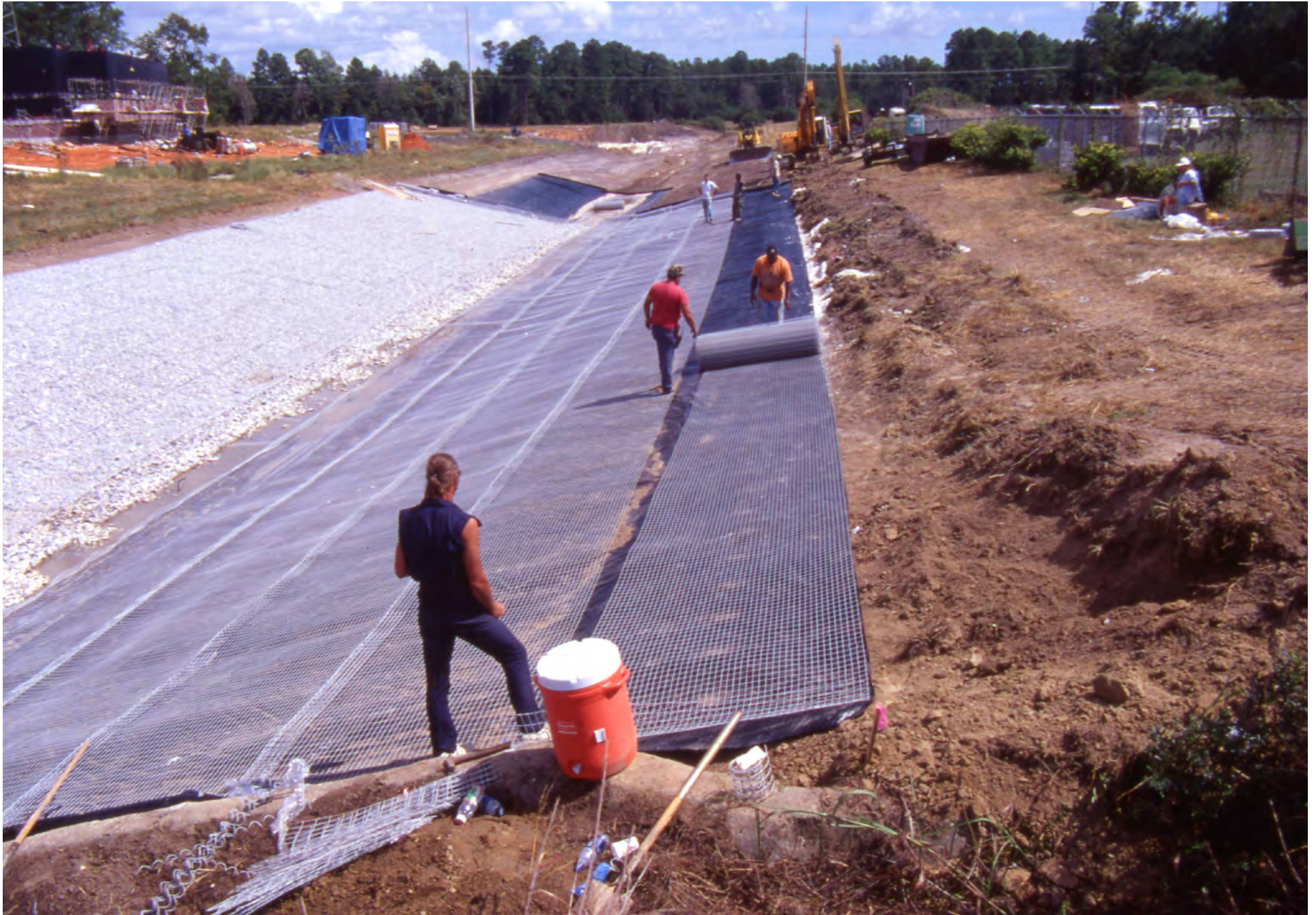
GABION MESH BEING UNROLLED OVER GEOTEXTILE
