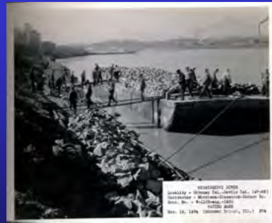
Hand Placing Stone Riprap
