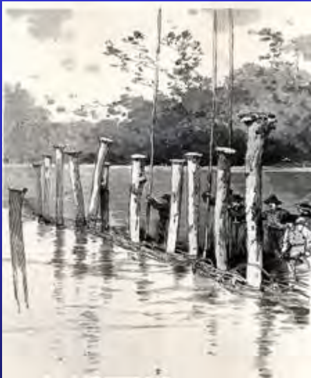
Workers Constructing Pile Dikes
