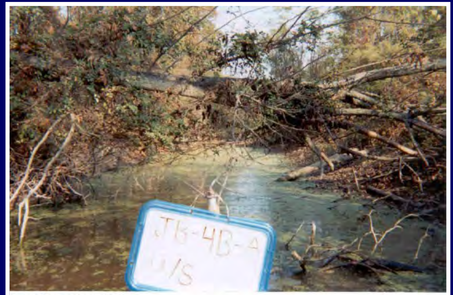
Description: looking upstream Contract No.: DACW38-00-D-0002 Task Order No.: 008 Date: 1/24/2001 Original: 4b_a_us.jpg Filename: jb4baus.jpg
