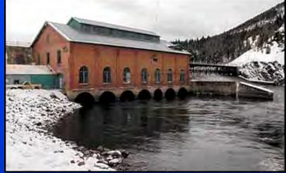
Milltown Dam on Clark Fork River, built 1907 Now part of nations largest Superfund site. Remedial action plan calls for phased removal of dam and contaminated sediments.
