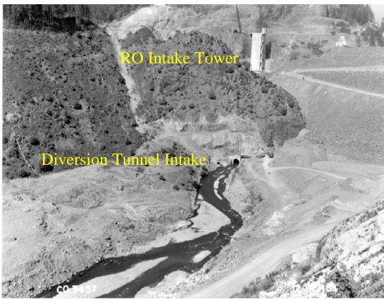
Construction photo, McKenzie River flowing into diversion, intake tower in background, Cougar Dam.
