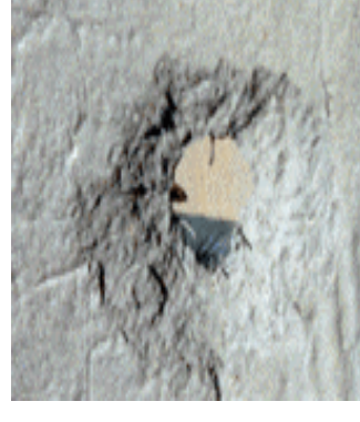
Double reinforced concrete wall
