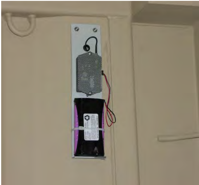
USMC TRICON with prototype Integrated Sensor / RFID
