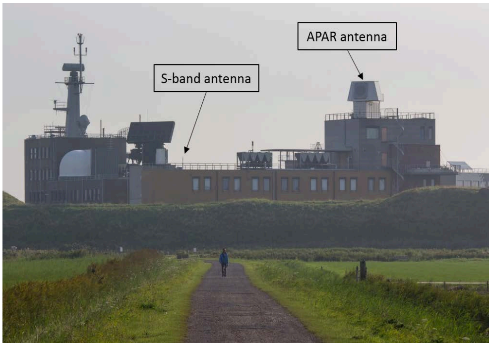
Figure 5. APAR and S-band antenna at the Salamander building.
