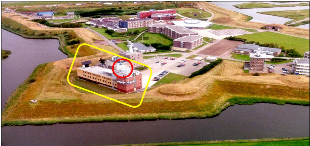
Figure 1. LBTS facility. Salamander building is in the foreground, indicated by the yellow box. The APAR antenna is indicated by the red circle.
