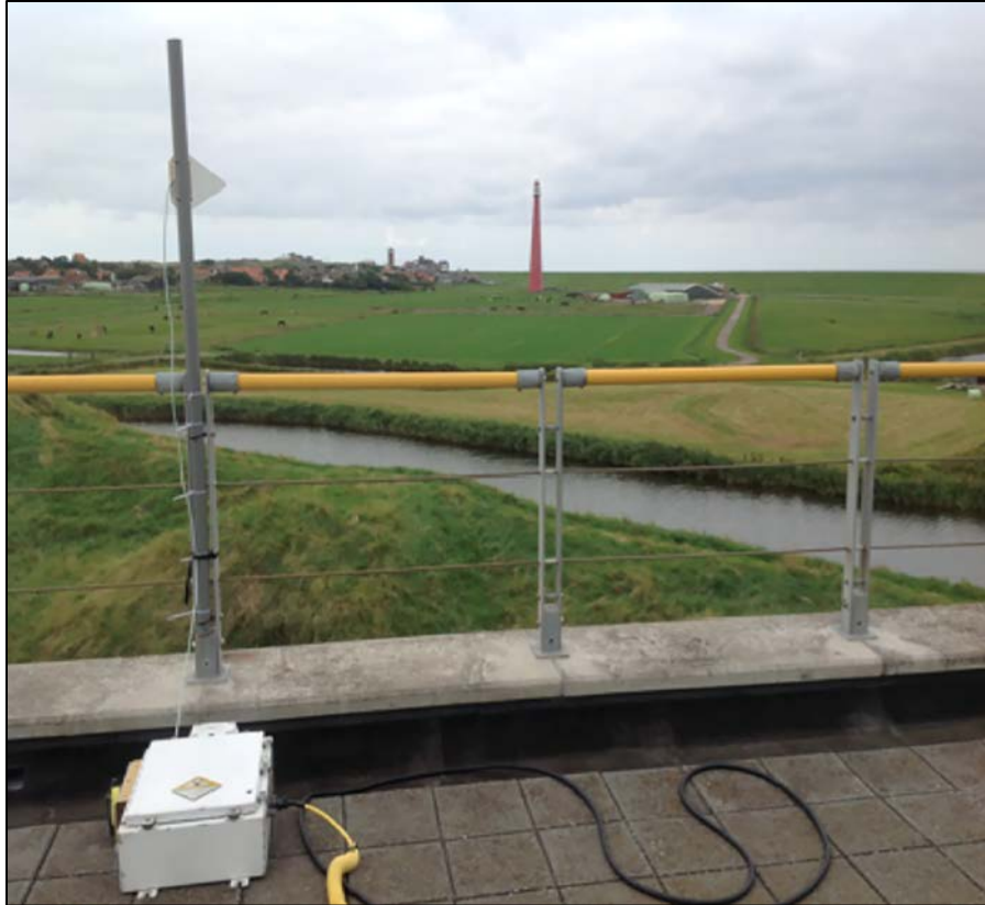
Figure 6. S-band transmitter and antenna on the rooftop of the Salamander building.
